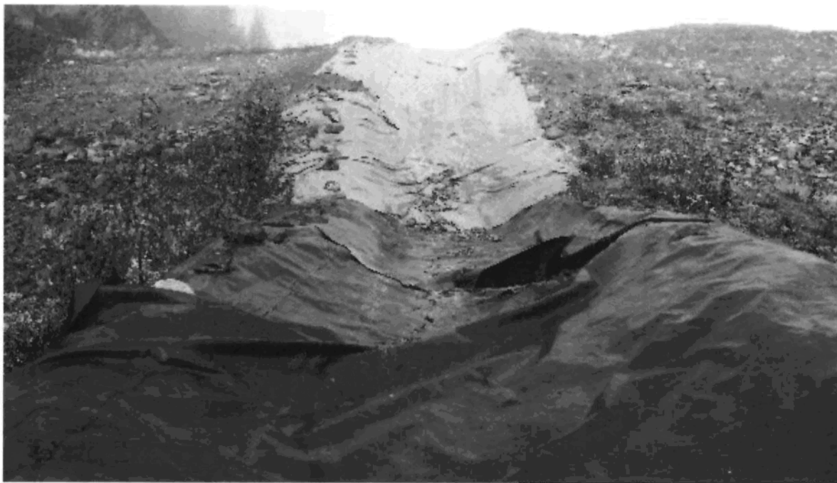
Picture 3: Spill way geo-membrane liner for spill way from Dam. Membrane is poorly installed and anchored.
