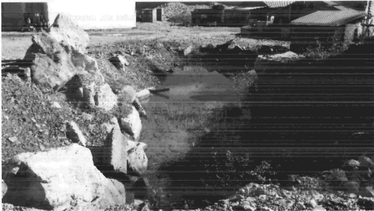
Picture 9: Sump/pond where mine water is collecting. At the time of the inspection, the site representative did not know where the water reported to.
