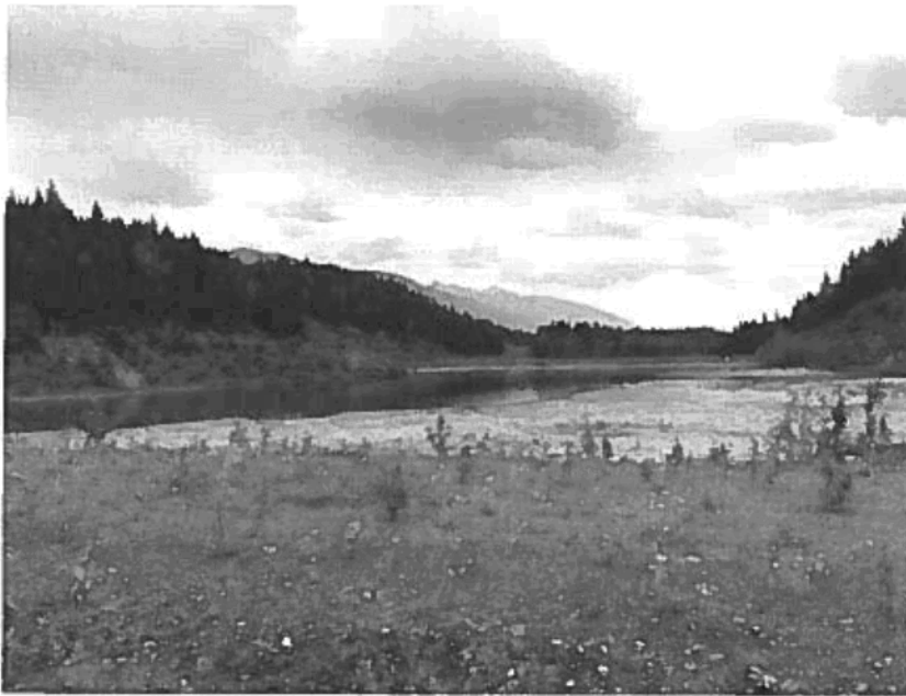
Photo 10. Exposed tailings above the water level along the north dam.
