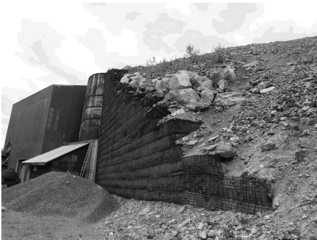
Photo 3: MSE wall retaining waste rock dump
