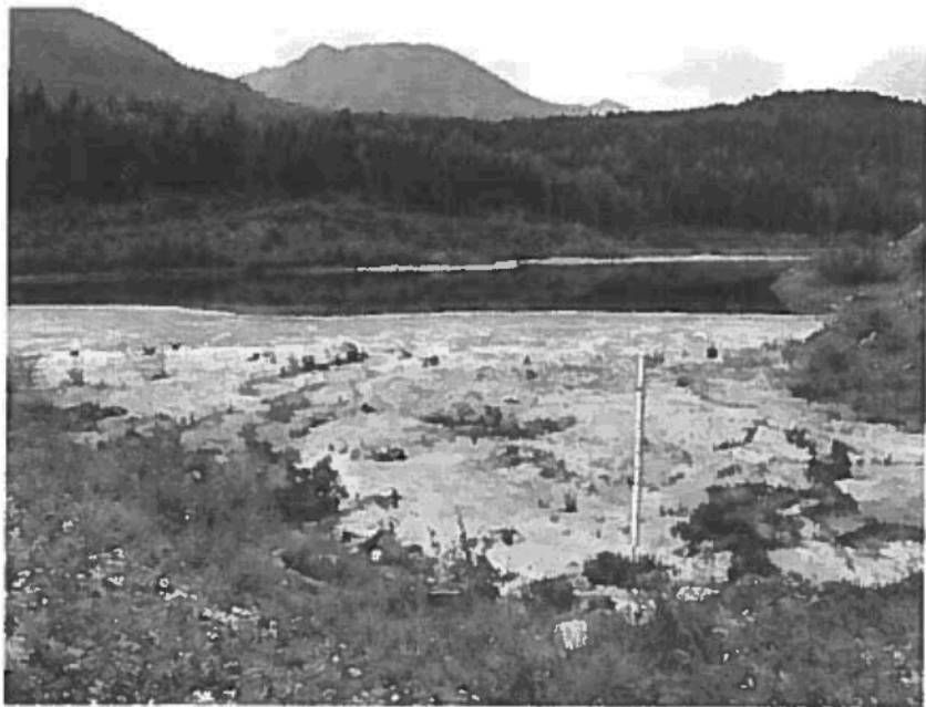
Photo 9. Exposed tailings above the water level along the southeast dam.
