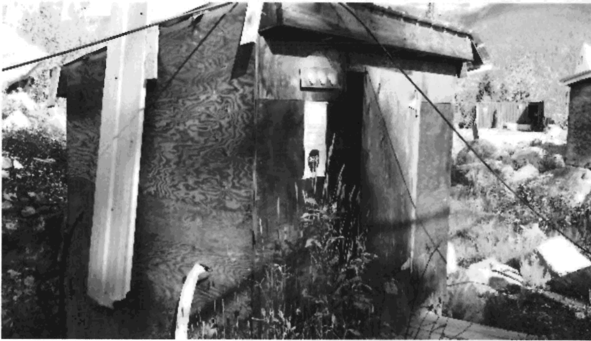
Picture 10: Pump shack and sump near mine entrance. Not appropriately signed and structure was not secured.
