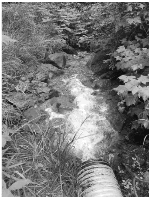
Photo 5. Portal settling pond outflow pipe.
