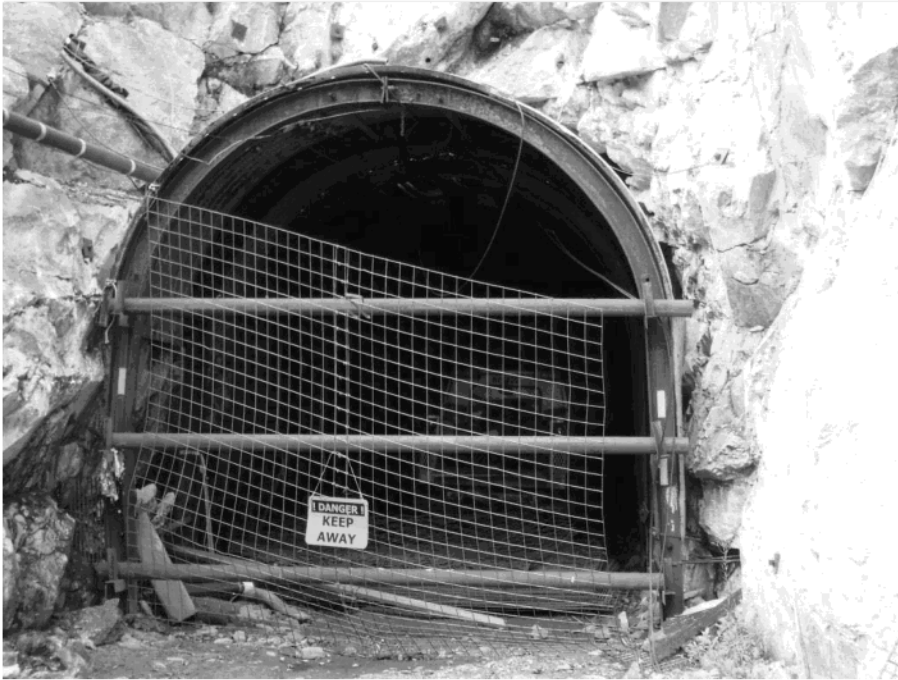
Photo 1: West Portal, note loose mesh
