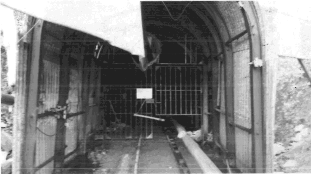
Picture 8: Second mine entrance remained open and unlocked. No effective barrier to access was in place as gate was unlocked. Note water along sides of this entrance.
