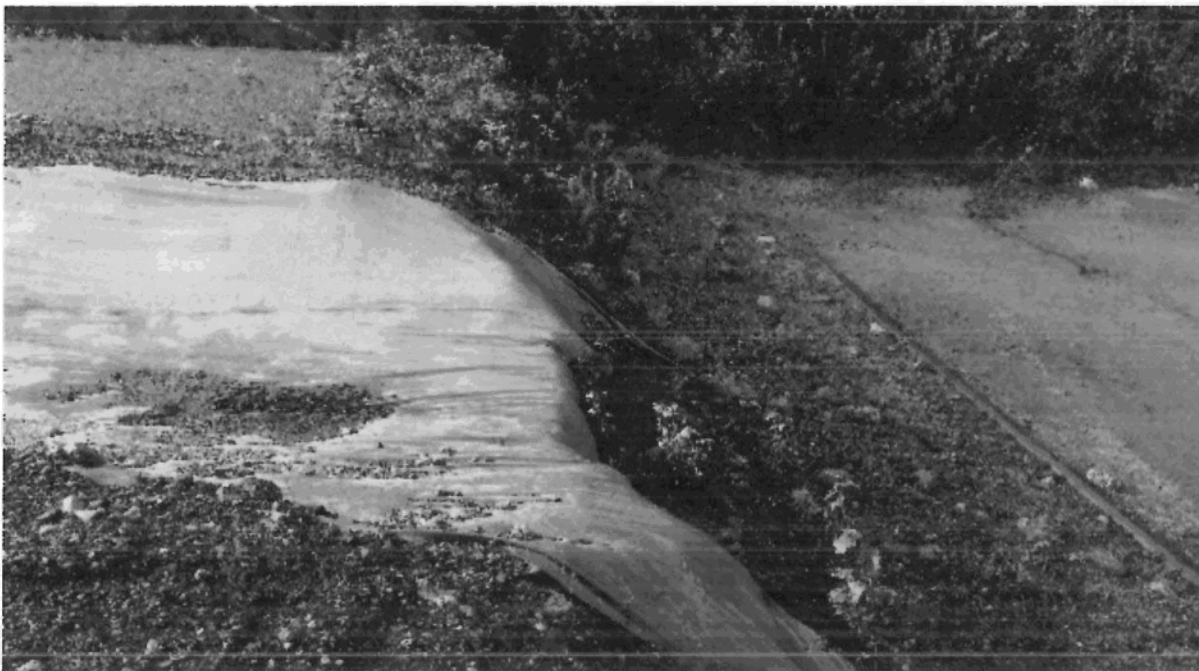
Picture 5: Outlet from tailings pond to the emergency spillway. Note that the edges of the liner are exposed/unanchored.
