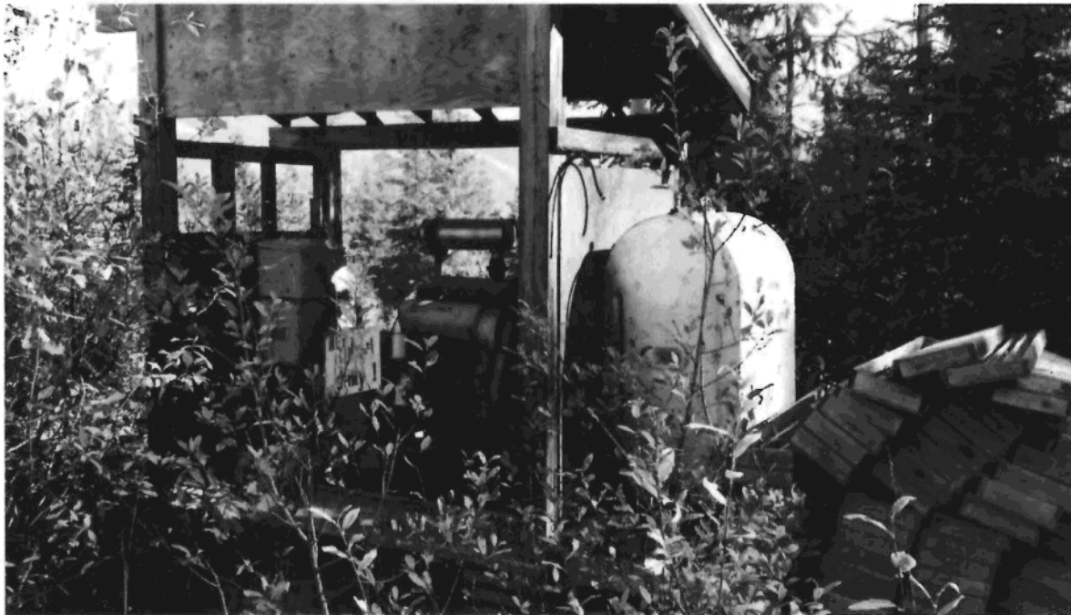
Picture 21: Generator with fuel storage at core storage area.
