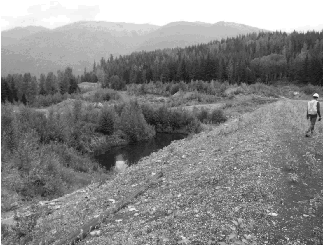
Photo 13: TSF, Northwest Dam downstream slope and ponded water at toe
