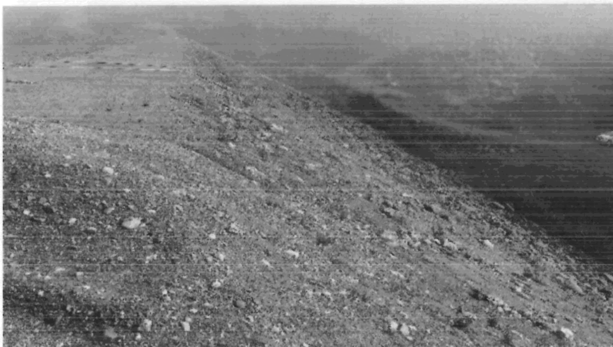
Picture 2: Note riling and minor erosion along crest of dam face. Also, note limited vegetation cover established on the upper section of the dam.
