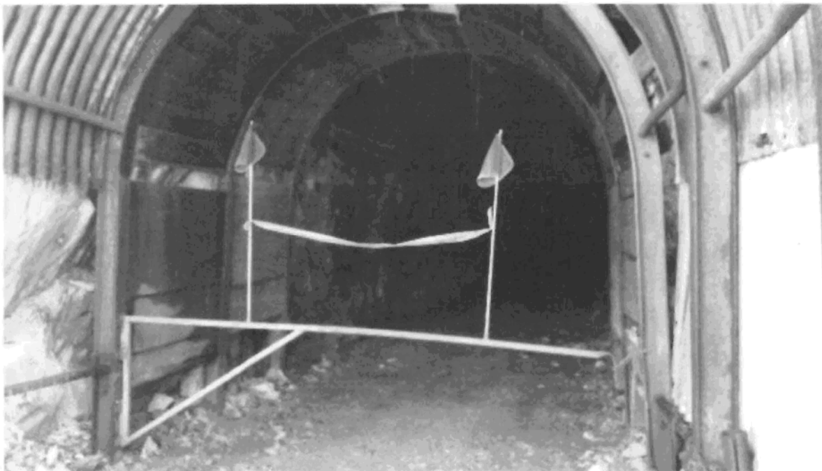
Picture 7: Mine entrance. Note, no gate or barrier to access has been established. The mine vehicle is the only control from accessing the underground.
