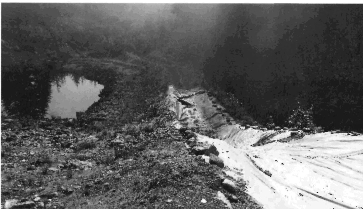
Picture 4: Note over all condition of the liner on the spillway (rips and improperly anchored). Liner does not extend to bottom of spill way.
