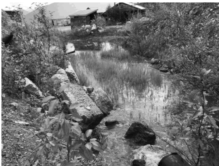
Photo 3. East and West Portal settling pond.
