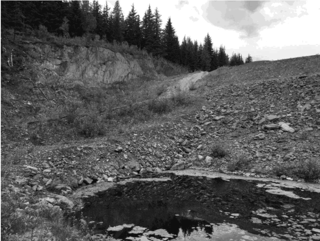
Photo 10: TSF, Southeast Dam downstream slope, note spillway towards left
