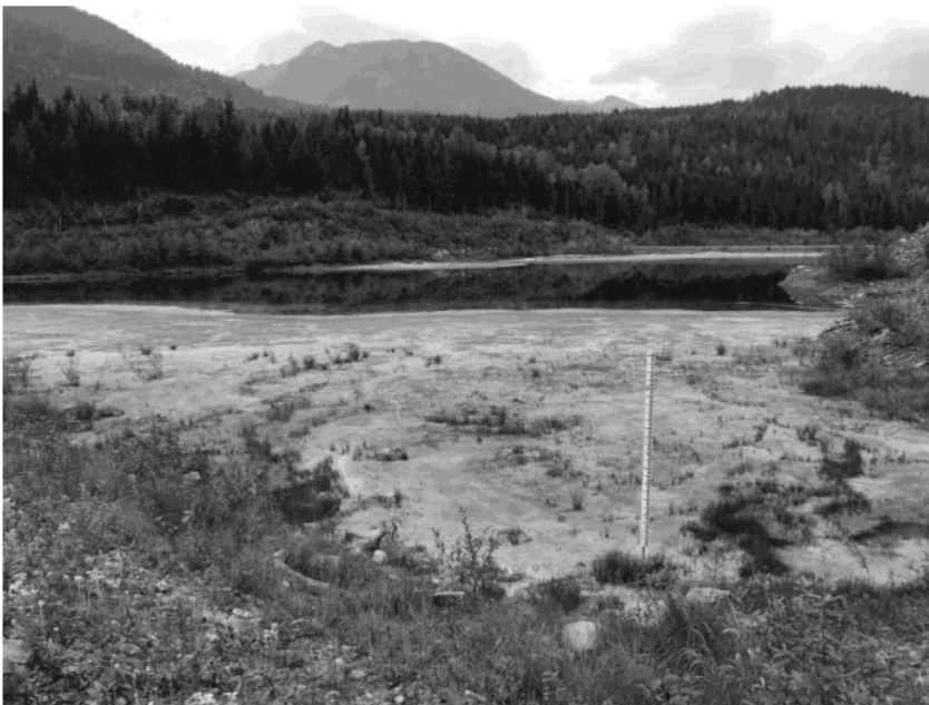
Photo 9. Exposed tailings above the water level along the southeast dam.
