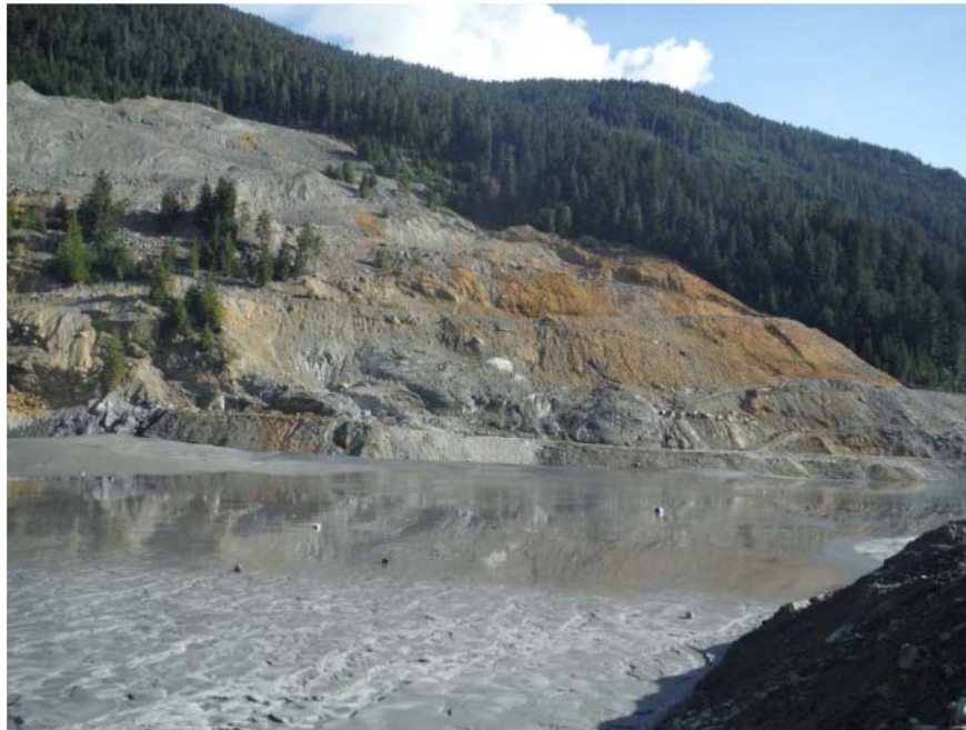
Figure 9. Looking from the crest of the embankment to the north-east across the surface of the tailings. In the foreground is sand, and behind this is the wet upper surface of tailings. Rising from the surface of the tailings are the natural bedrock slopes and waste rock dumps above the Lynx TDF.
