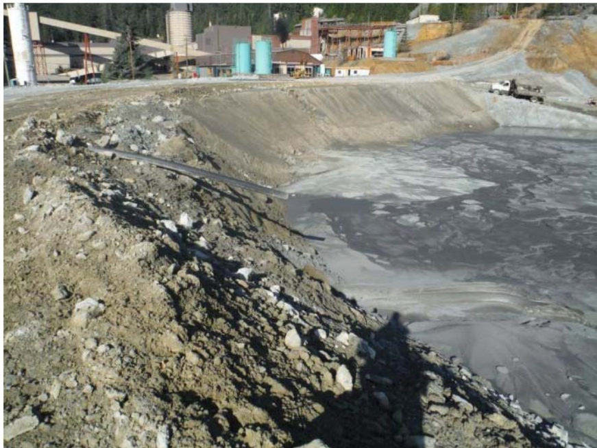
Figure 8. Looking east to west along the upstream crest of the embankment. Sand is deposited from the pipe in order to control the beach and hence to push standing water back and away from the embankment—a operating procedure that is considered to be good practice.
