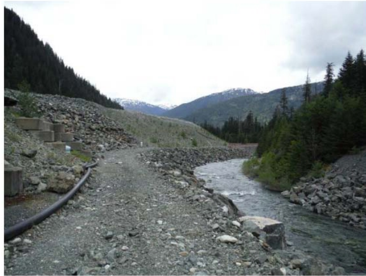
Figure 15. Looking east along the south face of the seismic berm. Note the large boulders (just beyond the concrete blocks) that constitute the spillway just to the left of the photo.
