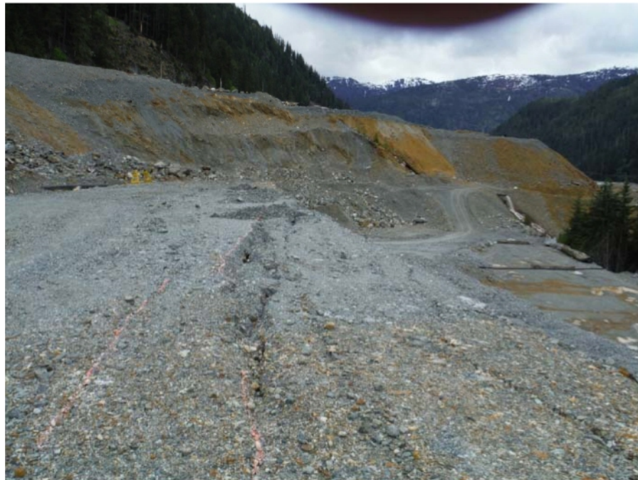
Figure 3. Cracking along the downstream crest of the embankment as observed in June 2013. The cracked zone was, reportedly, removed and replaced as part of 2013 embankment raising.
