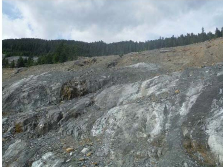
Figure 12. Seepage from joints in the bedrock on the north side of the Lynx TDF. Flow quantities vary in response to precipitation. The zone of bedrock seepage is relatively large and extends some meters up the slope.
