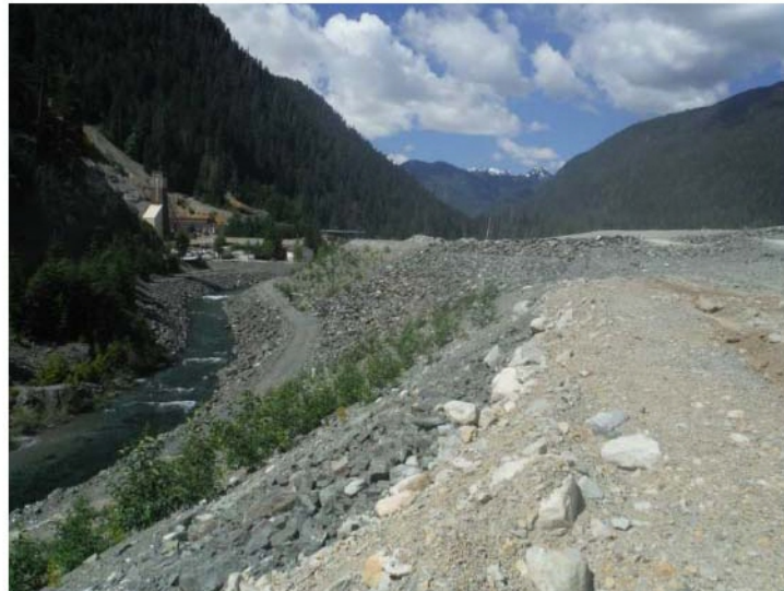
Figure 14. The outer face of the seismic berm, looking north. Note from left to right: Myra Creek; the toe access road; and the sloping face of the berm with new vegetation.
