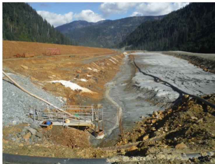
Figure 9. The Strip Area looking east. Surface water runs in the “channel” to the decant facility, which is seen in the foreground of the photo.
