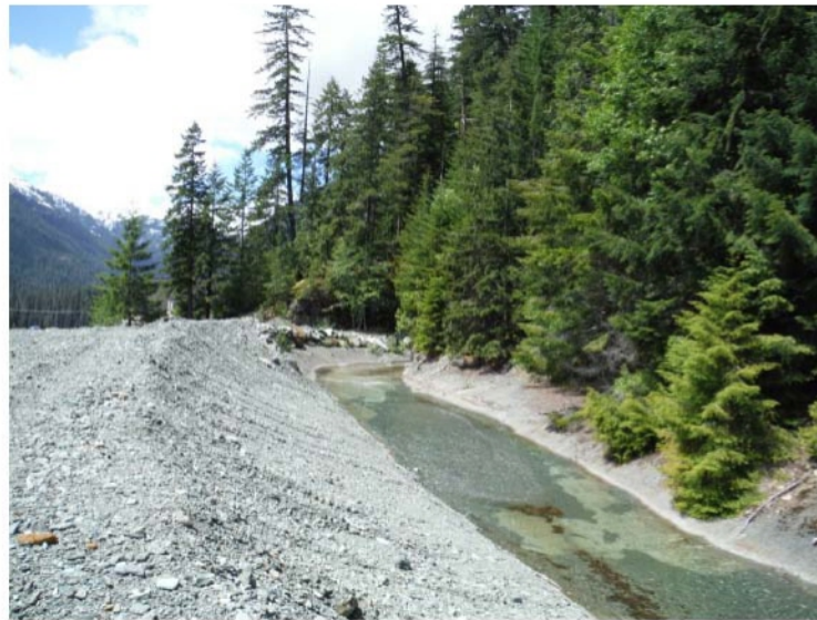
Figure 1. The Upgradient Drainage Channel on the north side of the TDF. Note the shotcrete lining on the upgradient side. The light-colored material on the downstream side is gravel that accumulated in the channel and was subsequently removed from the channel.
