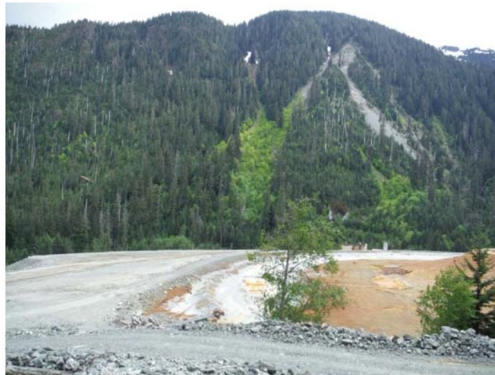
Figure 11. The top surface of the old tailings and seismic buttress. The surface was being regraded to comply with closure requirements.
