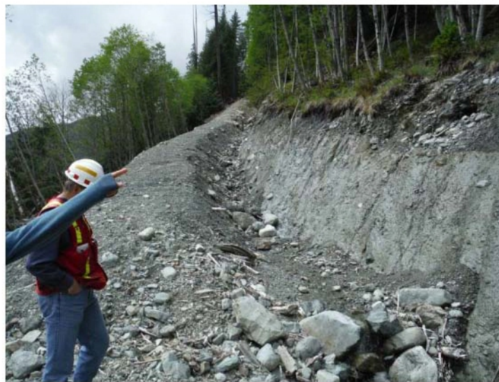
Figure 2. The Secondary Upgradient Channel. Note the steep cut into consolidated clay on the upgradient side. Note also the accumulation of gravels and boulders in the channel.
