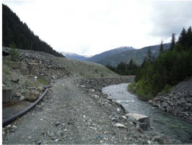
Figure 15. South face of seismic berm. Note the large boulders that constitute the spillway just to the left of the photo.
