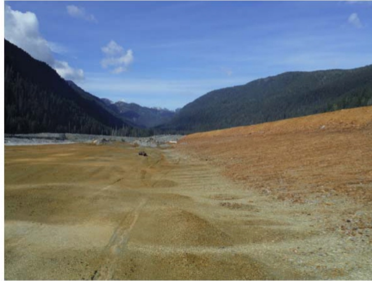
Figure 10-A. The toe of the paste berm looking west. This is the general area where wet and soggy conditions were observed on the flat surface at the toe of the berm.
