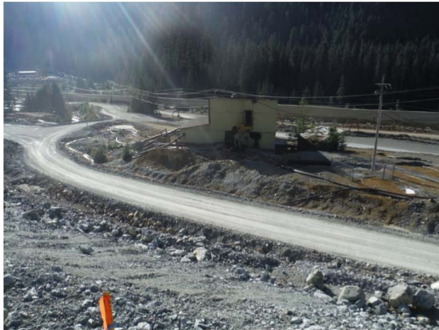
Figure 5. The access road along the toe of the embankment. To the bottom left of the picture is the inclined downstream face of the embankment. Above, and to the right of the access road are various material stockpiles and other facilities that will be removed to make way for the embankment as, in the future, additional embankment raising is undertaken.
