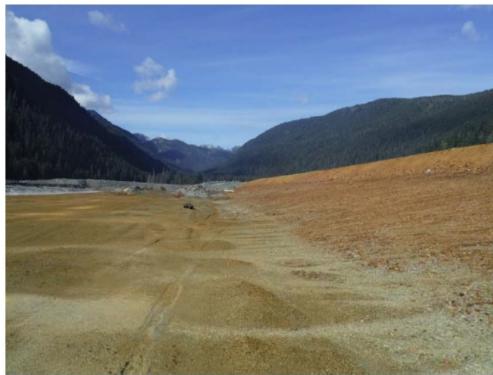
Figure 10-A. The toe of the paste berm looking west. This is the general area where wet and soggy conditions were observed on the flat surface at the toe of the berm.
