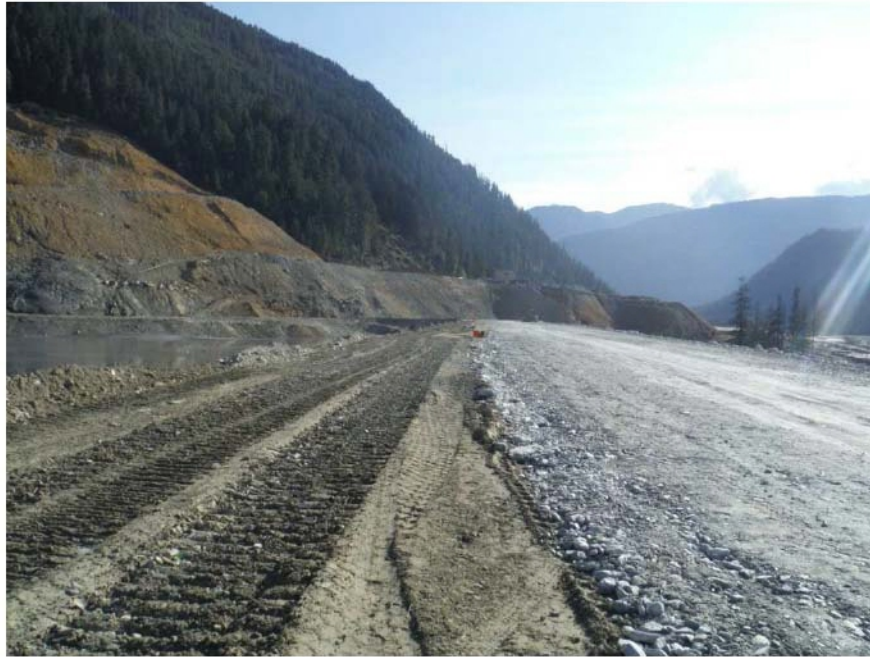
Figure 6. Looking west to east along the upstream crest of the embankment. To the left is the compacted finer-grained material of the filter zone; to the right is the top surface of the compacted waste rock.
