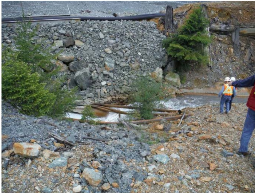
Figure 16. The area downstream of the embankment where tailings bleed water may report via an underdrain at the base of the starter dam.
