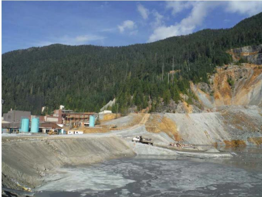
Figure 11. The truck has just dumped refuse at the right-hand end of the road that slopes down to the tailings surface. Note also the significant difference in elevation shown here between the top of the tailings and the crest of the embankment.
