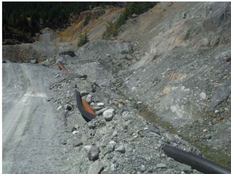
Figure 13. The channel to the east end of the north side of the Lynx TDF. The channel is formed of the bedrock and piled-up waste rock, Seepage is collected in the channel and flows east.
