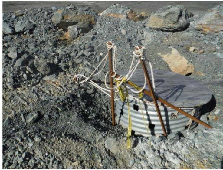
Figure 7-C. The inlet to the decant pipe from the Amalgamated Paste Area. Note the wooden top. Water is intended to pass through the square openings in the pipe.
