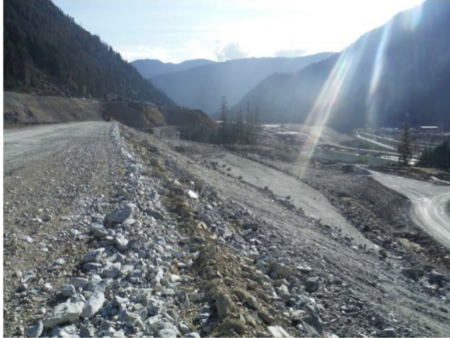
Figure 4. Looking west to east along the downstream crest of the embankment dam in September 2013. To the left of the crest line is the top of the embankment, which is a compacted surface of waste rock. To the right of the crest line is the downstream face of the embankment which is also compacted waste rock.
