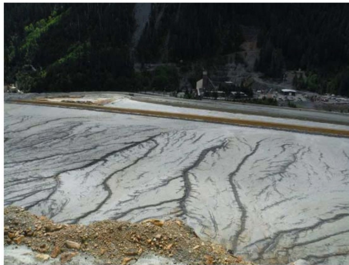
Figure 6. Erosion of the upper surface of the paste tailings, looking from north to south.
