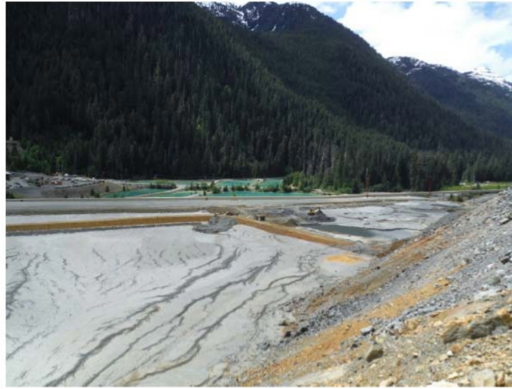
Figure 7-A. The decant location at the south-west corner of the paste tailings area. The sand management area (Section 4.8) is to the west. At the bottom right of the photo are the steeper slopes of the waste rock dump.
