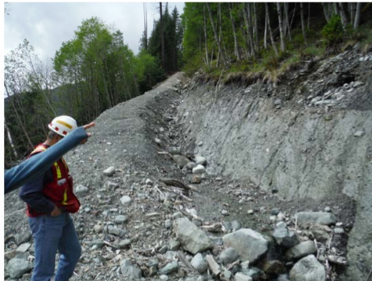
Figure 2. The Secondary Upgradient Channel. Note the steep cut into consolidated clay on the upgradient side. Note also the accumulation of gravels and boulders in the channel.
