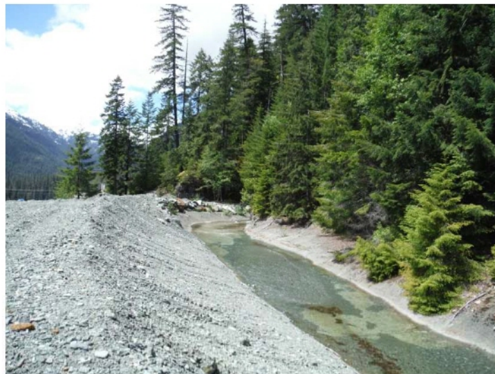
Figure 1. The Upgradient Drainage Channel on the north side of the TDF. Note the shotcrete lining on the upgradient side. The light-colored material on the downstream side is gravel that accumulated in the channel and was subsequently removed from the channel.
