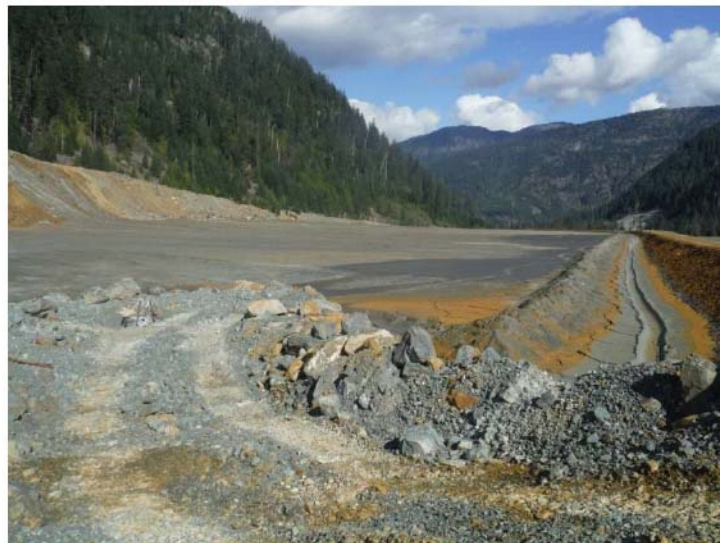
Figure 7-B. Looking east along the paste berm. The Amalgamated Paste Area decant facility as seen from the south-west corner of the area. Note surface water runs east to west in the channel to the right of the photo, then ponds to flow into the area of rock in the middle of which is the decant pipe leading to the Super Pond which is located at the upstream end of the site's water treatment system.
