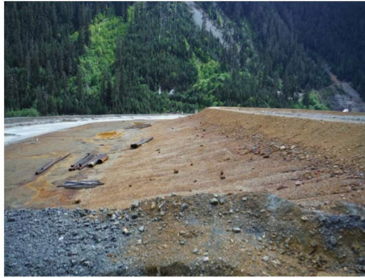
Figure 8. The downgradient side of the paste berm. Note the variable slope inclination leading to the tailings surface on the left side of the photo.
