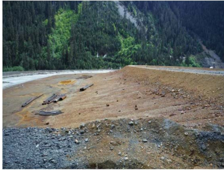
Figure 8. Looking southwest along the paste berm from the east end of the paste berm area. The downgradient side of the paste berm. Note the variable slope inclination leading to the tailings surface on the left side of the photo.
