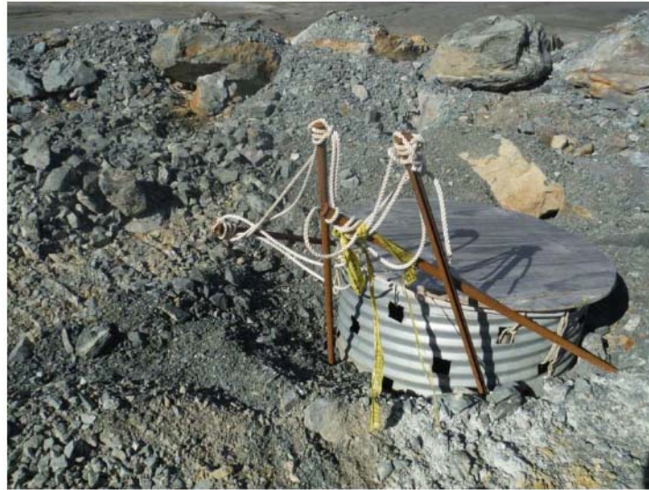
Figure 7-C. The inlet to the decant pipe from the Amalgamated Paste Area. Note the wooden top. Water is intended to pass through the square openings in the pipe.
