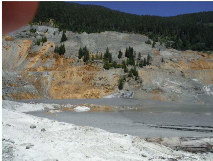
Figure 15. The slopes upgradient and to the north of the Lynx TDF. Some interception and diversion of runoff is achieved via the roads and channels of this area.
