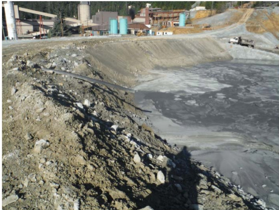
Figure 8. Looking east to west along the upstream crest of the embankment. Sand is deposited from the pipe in order to control the beach and hence to push standing water back and away from the embankment.
