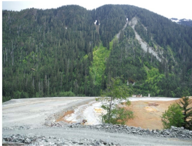
Figure 11. The top surface of the old tailings and seismic buttress. The surface was being regraded to comply with closure requirements.
