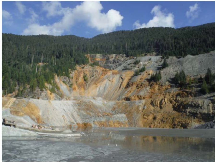
Figure 10. Looking from the crest of the embankment to the northwest across the surface of the tailings. Rising from the surface of the tailings are the natural bedrock slopes and waste rock dumps above the Lynx TDF
