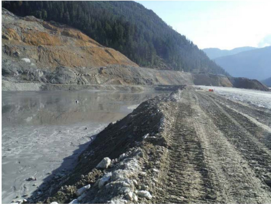
Figure 7. Looking west to east along the upstream crest of the embankment. To the left is the surface of the tailings
