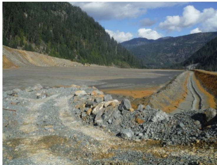
Figure 7-B. The Amalgamated Paste Area decant facility as seen from the south-west corner of the area. Note surface water runs east to west in the channel to the right of the photo, then ponds to flow into the area of rock in the middle of which is the decant pipe leading to the Superpond.
