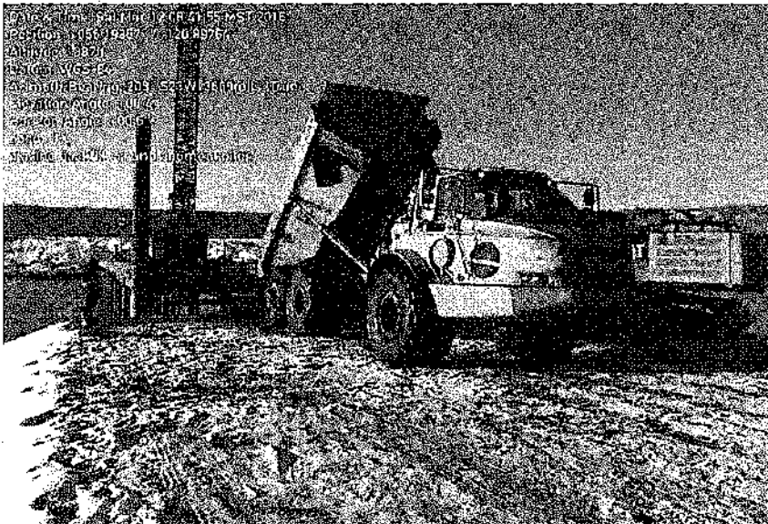
Figure A2 Contractor backfilling the approach to the Peace River Construction Bridge
