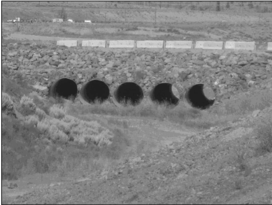
PHOTO 7 – Culverts installed in spillway channel. Culverts installed in 2011 by New Gold.
