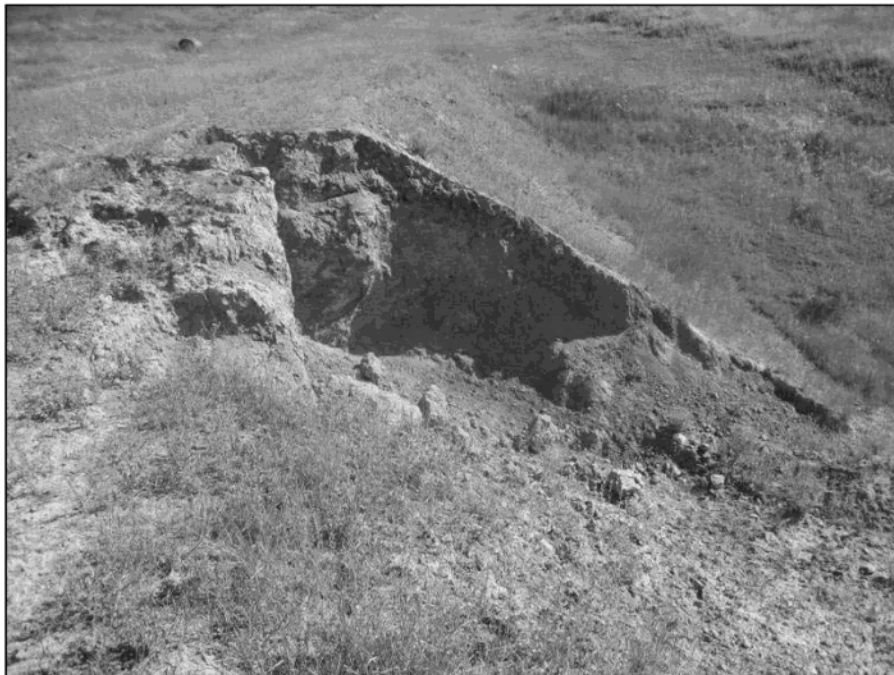
PHOTO 8 – Eroded section of the southwest seepage dam.
