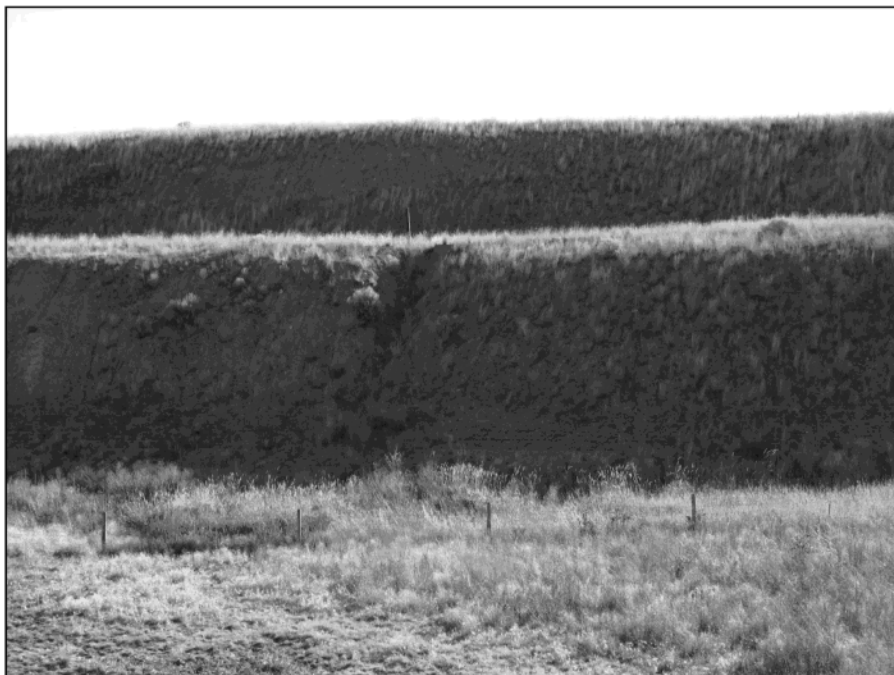
PHOTO 2 – Downstream toe of West Dam showing small erosion gullies.
