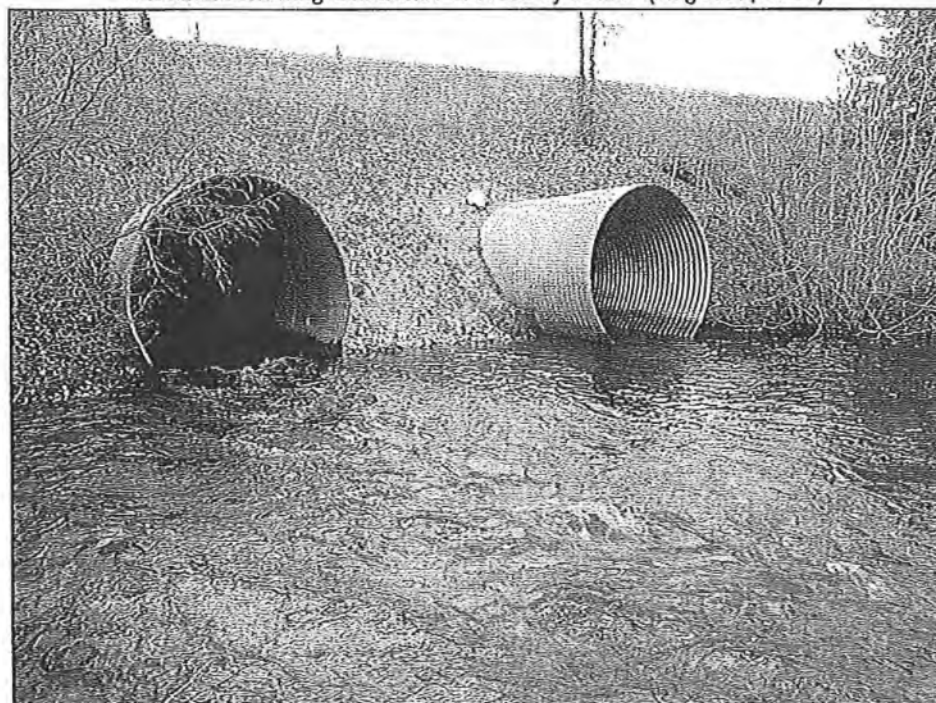
Plate 8 Yellowhead Creek: View upstream towards culvert outlets showing inundation of both culvert outlets under fall low-flow conditions (October 17, 2011).
