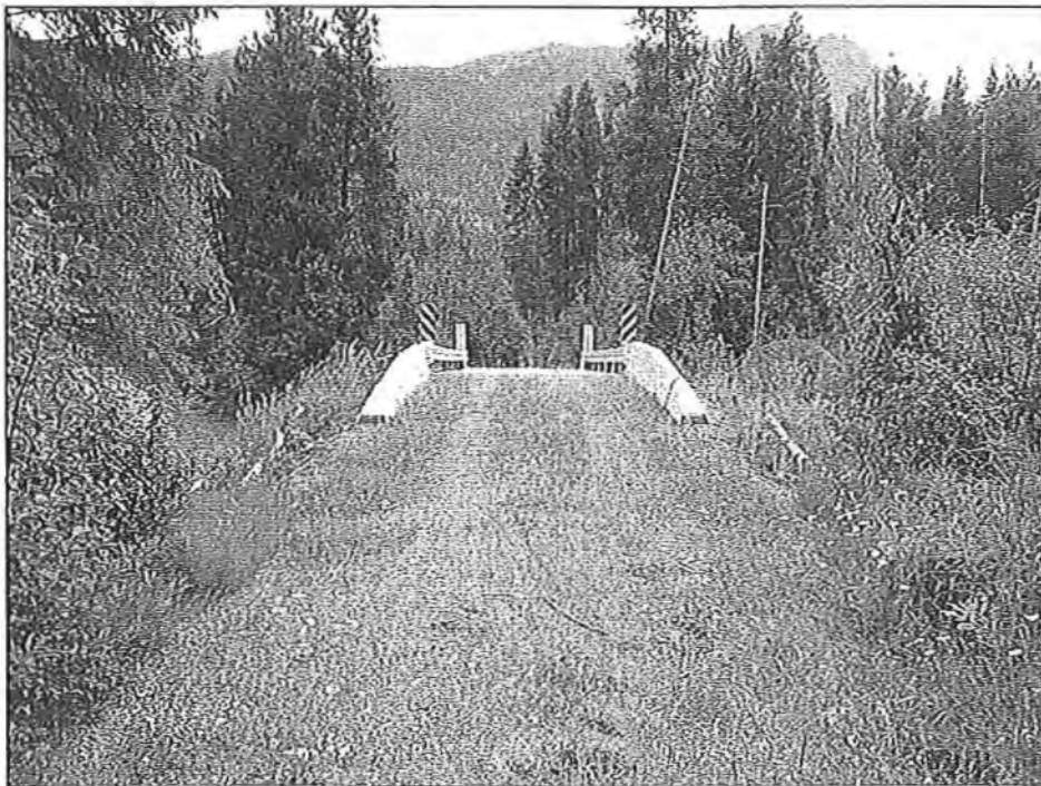
Plate 12 Fraser Back Channel: View north along left bank approach ramp showing regenerating vegetation on ramp shoulders (August 7, 2011).
