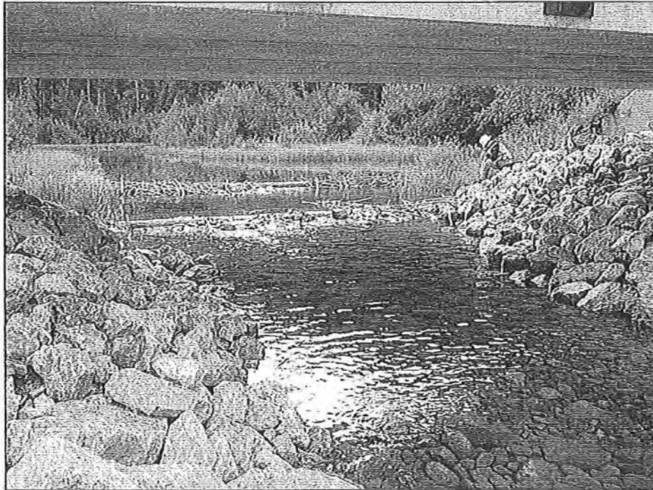
Plate 10 Fraser Back Channel: View upstream through new channel showing the two log weirs and cobble lined pool created under bridge deck (August 7, 2011).
