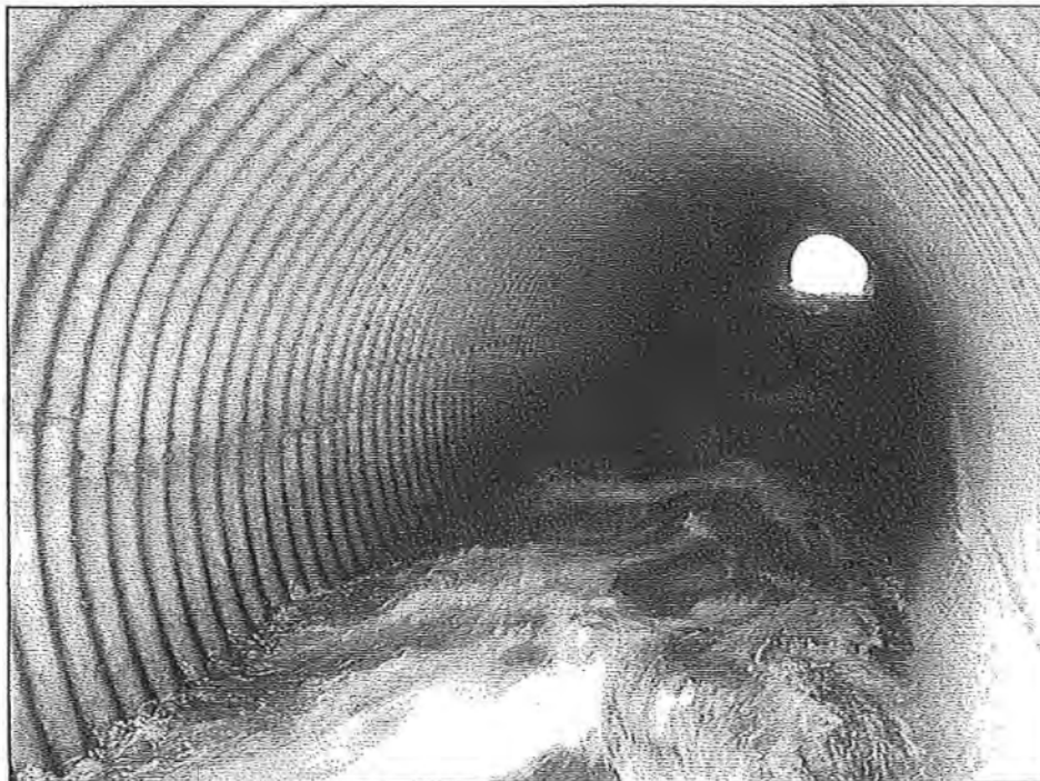
Plate 7 Yellowhead Creek: View downstream through west culvert under moderate flow conditions showing turbulence created by baffles (August 7, 2011).
