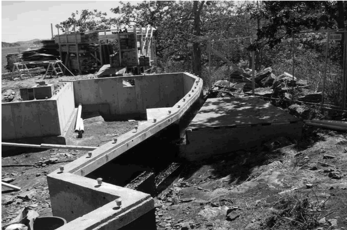
Plate 1: View of Rock Feature #10 housed within a plywood box. The interior portion of this feature is enclosed in concrete.
