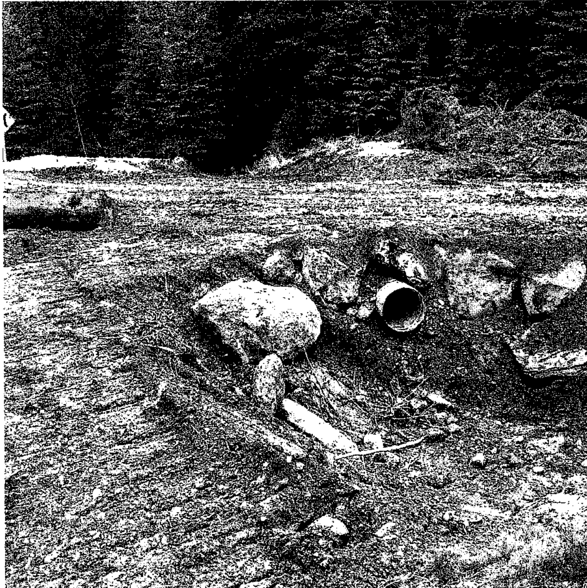
Figure 10: New culvert on the Jumbo Forest Service Road, example of GRL road improvements (From EAO Environmental Assessment Office – Substantially Start Site Inspection, October 13, 2014)
