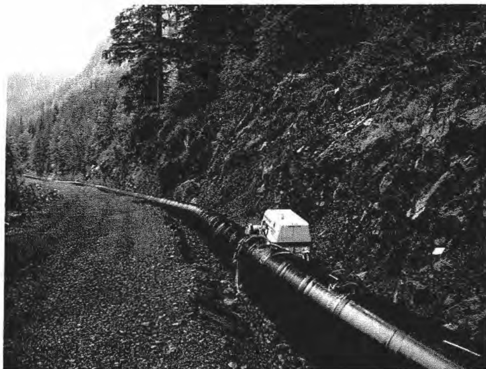
Figure 5. Penstock being put in place during construction.
