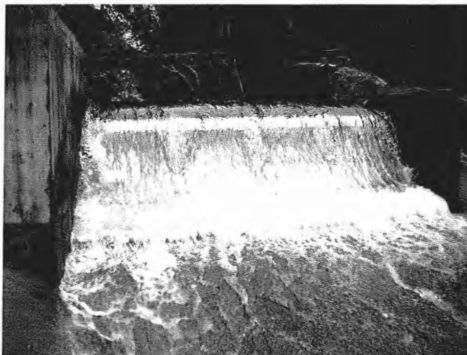
Figure 1. Marion 3 Coanda screen intake.
