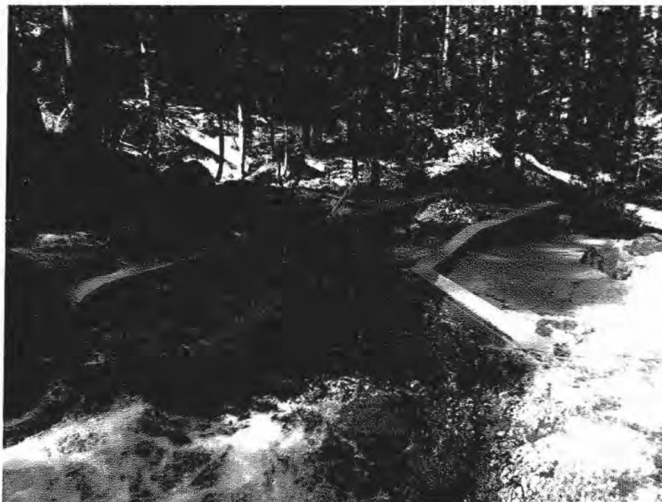
Figure 2. Marionette Creek Tyrolean weir intake.
