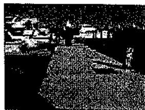
CONCRETE BREAKWATER WITH ALUMINUM FINGERS
