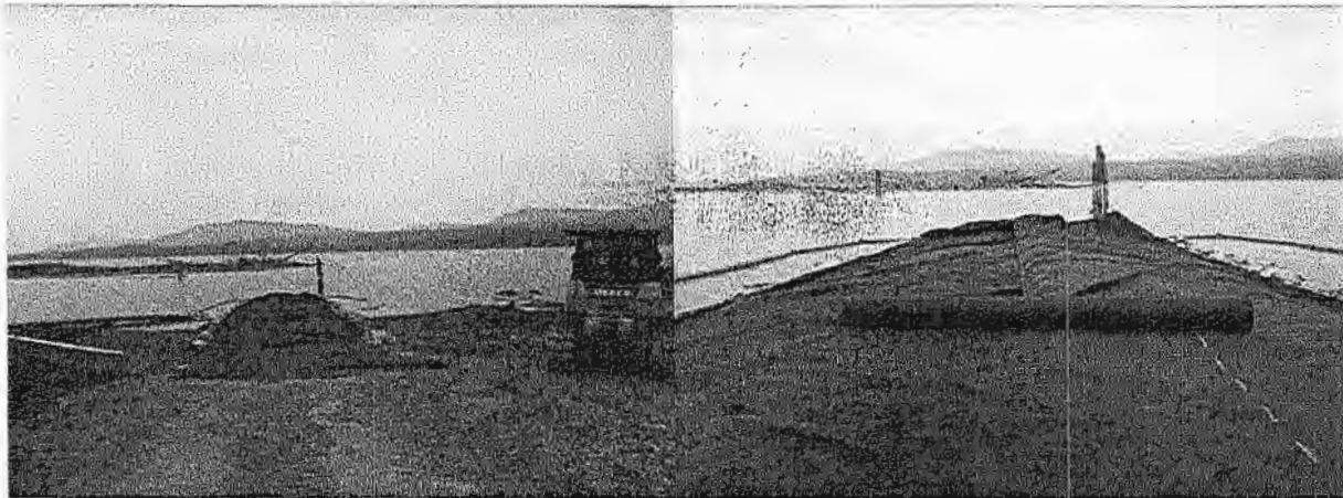
FIGURE 5: GEO MEMBRANE OVERLAYING THE RIP RAP
