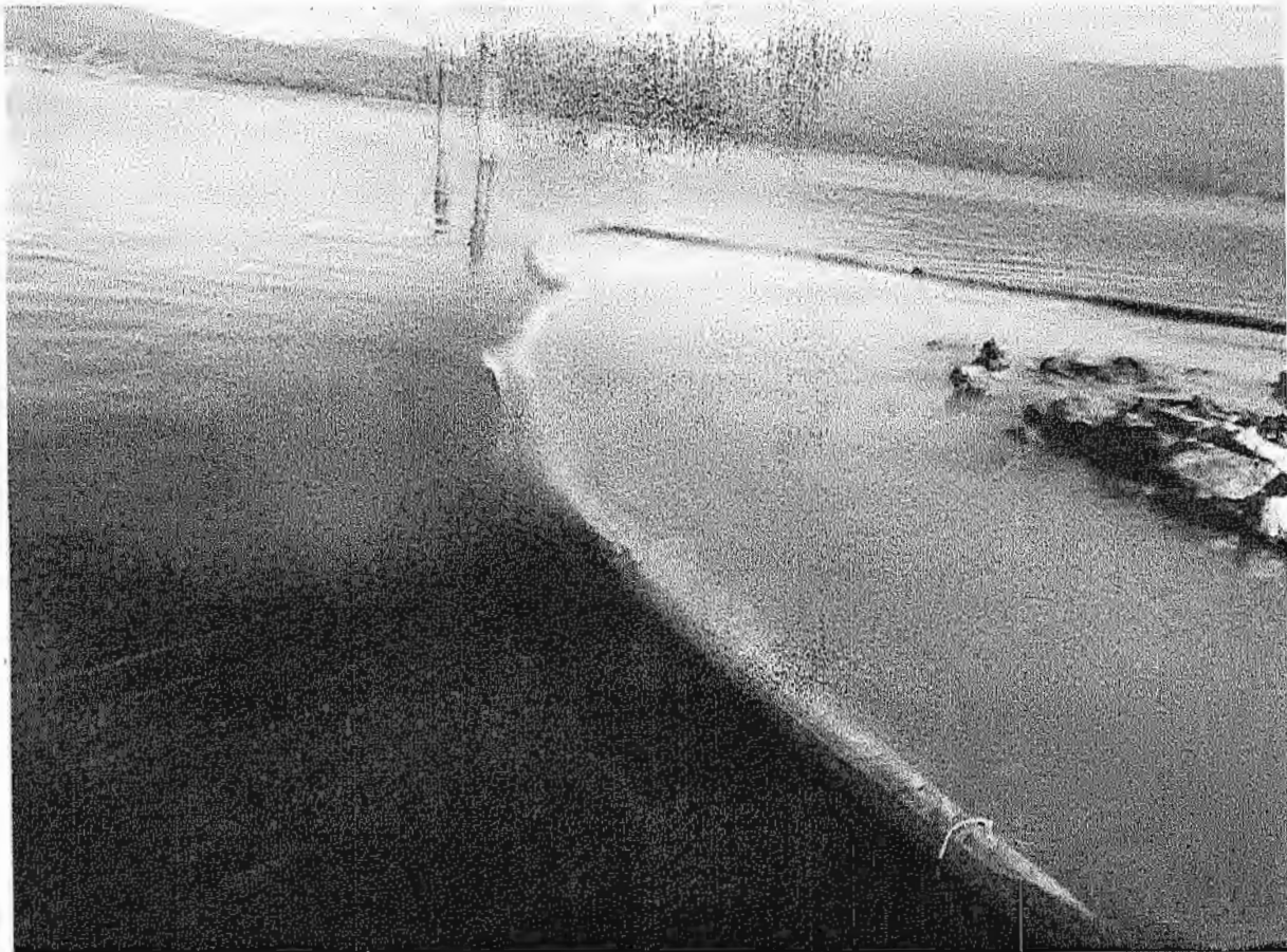
FIGURE 9: THE SILT CURTAIN EFFECTIVELY CONTAINED MOST OF THE FINES DURING CONSTRUCTION
