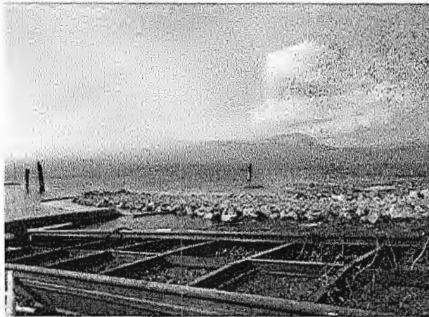
FIGURE 3: COMPLETED RIP RAP FOUNDATION
