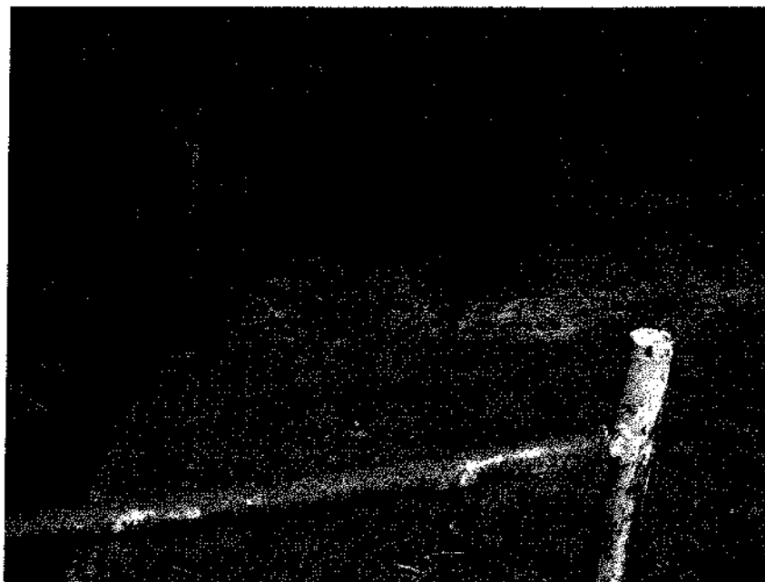
Downstream toe of dam – note seepage approx 3m from toe of dam- may be associated with road drainage- inspect and monitor
