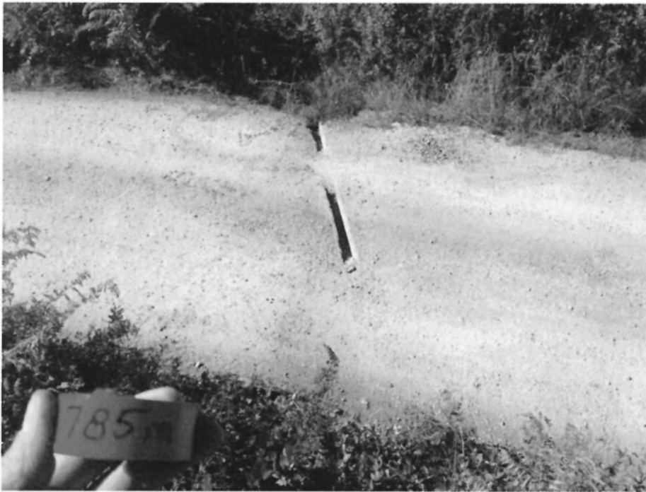
Figure 9: Sakinaw Woods Section 1 - 785m hand built cross drainage. Clean
