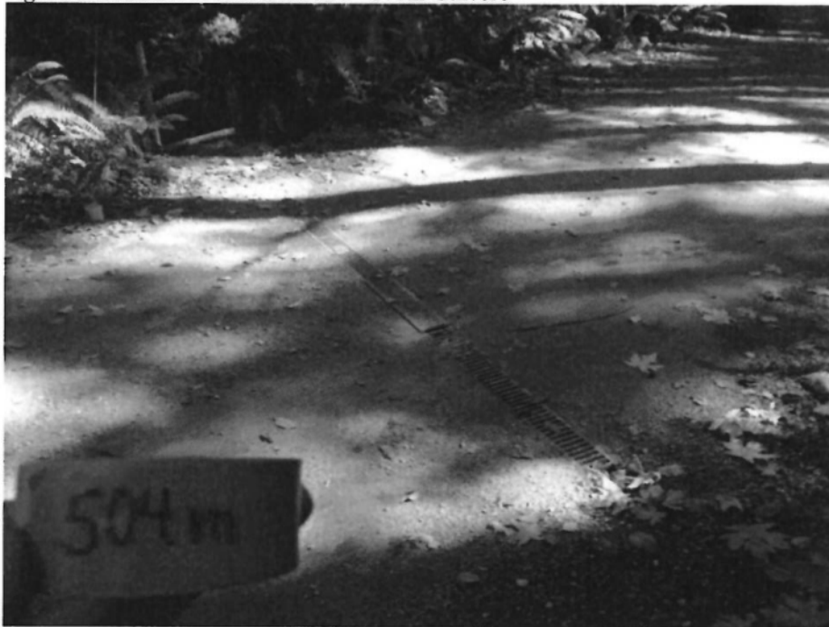
Figure 6: Sakinaw Woods Section 1 - 504m steel grate drainage. Clean outlet
