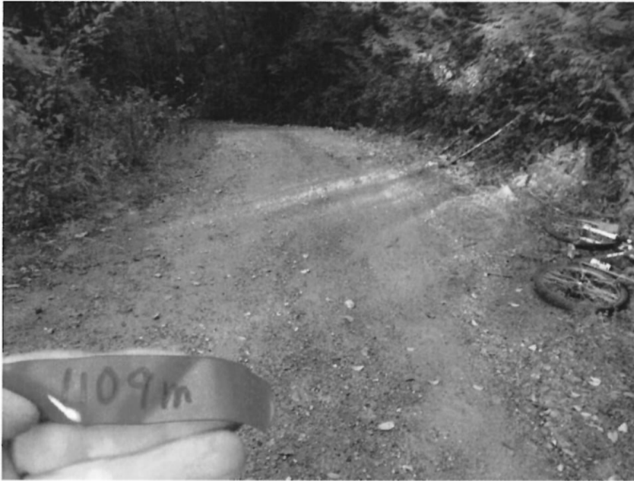
Figure 17: 1109m Start of steep pitch. Add double kicker to use both ditchlines
