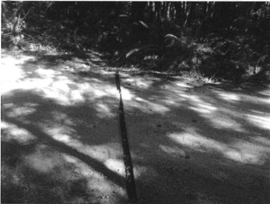
Figure 4: Sakinaw Woods Section 1 - 310m Hand built waterbar. Clean out
