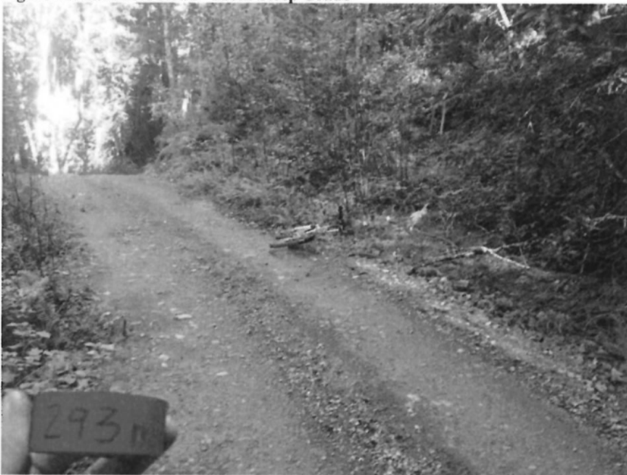
Figure 12: Saunders Road - 293m waterbar and old borrow pit
