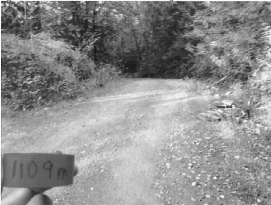
Figure 16: 1109m Start of steep pitch. Add double kicker to use both ditchlines
