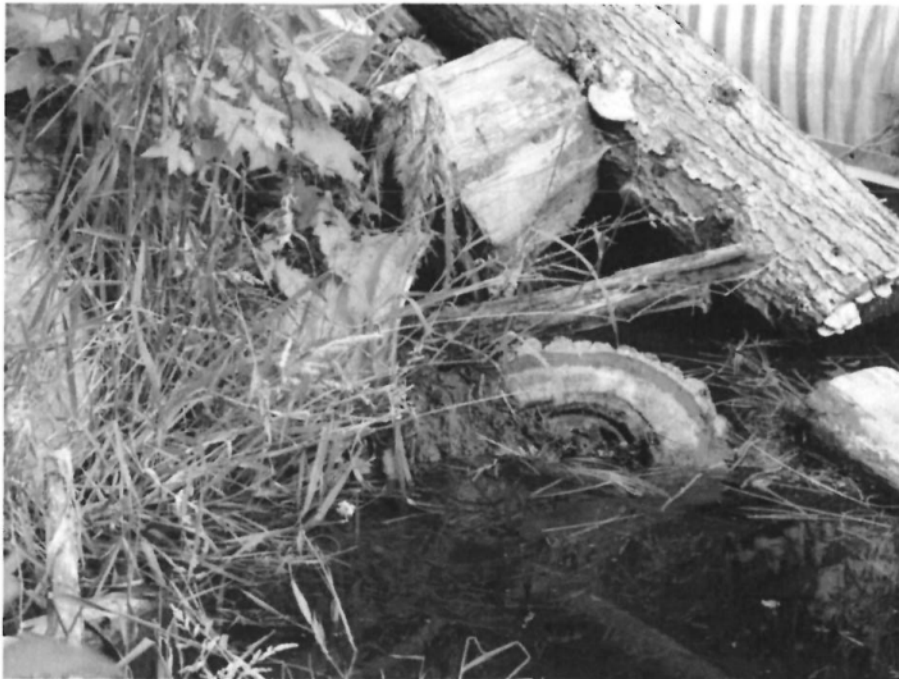
Plate 12: Dale Fennell photograph from July 12, 2013, showing the inlet of the lower culvert on the road crossing. The culvert appears to be partially jammed with debris as water is halfway up the culvert but it may still be active and controlling the lake level.
