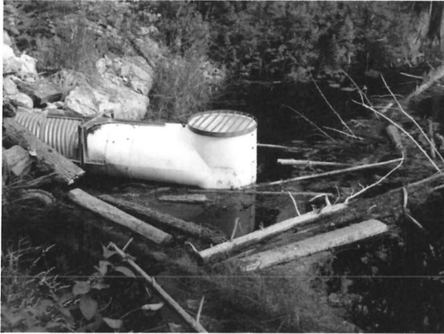
Plate 11: Dale Fennell photograph from July 12, 2013, showing the inlet of the upper culvert on the road crossing. Woody debris around the inlet is cut by humans. The base of the upper culvert is at lake level, suggesting that this culvert may be controlling lake level and that the lower culvert is partially blocked.
