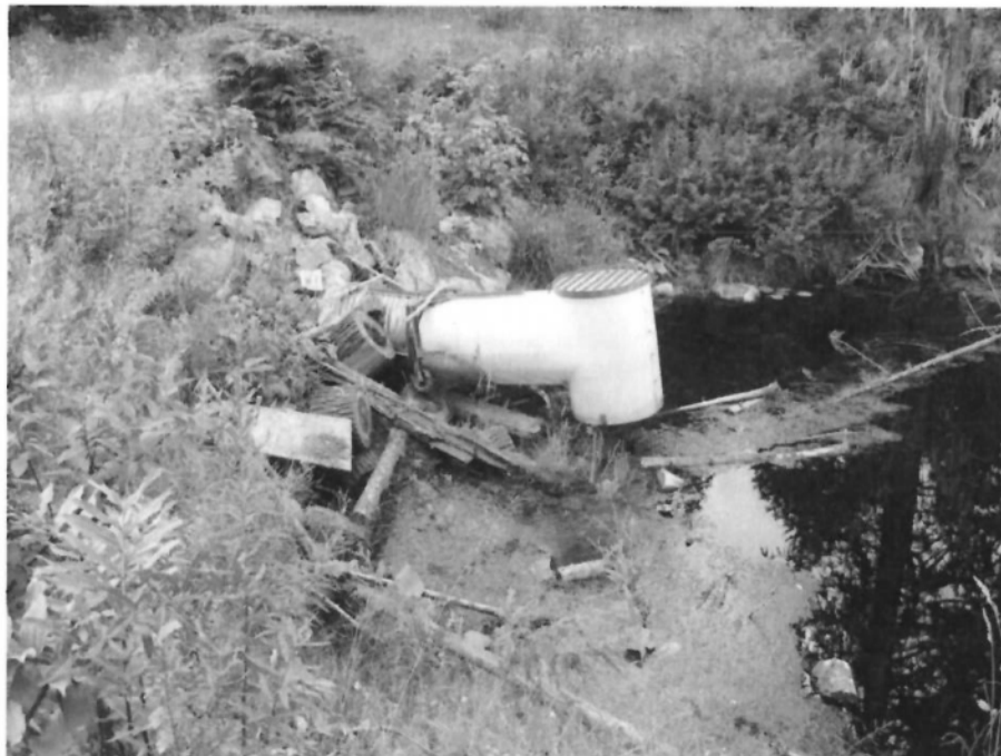
Plate 10: Dale Fennell photograph from August 21, 2012, showing the inlet of the upper culvert on the road crossing. The lower culvert is not visible but the lake is below the base elevation of upper culvert suggesting the lower culvert is allowing some flow and controlling lake level.
