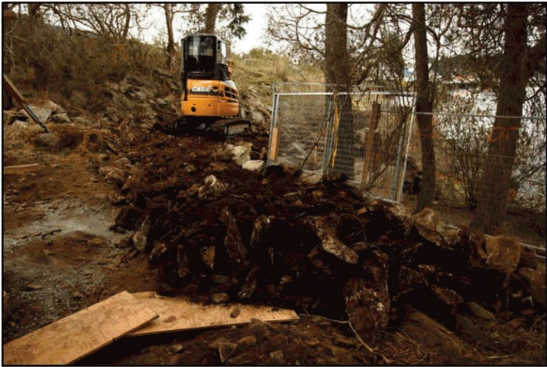
Figure 33. Overburden removed along the entrance ramp right-of-way is re-deposited to form pathway to house entrance stairway. Nothing was found along the entire right-of-way.
