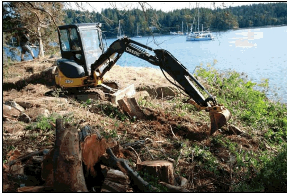
Figure 7. Picture showing clearing of the staging area on the northeast side of the Islet. Note all of the materials in view have been previously disturbed. This area consists of primarily fill materials from previous surface activities.
