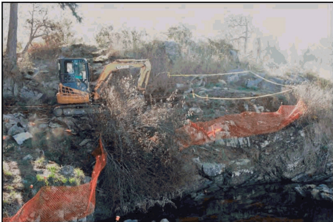
Figure 32. Clearing of soil and rock debris overburden along proposed entrance-way ramp location. Nothing was found along the entire right-of-way. All overburden was removed and re-deposited closer to the building.
