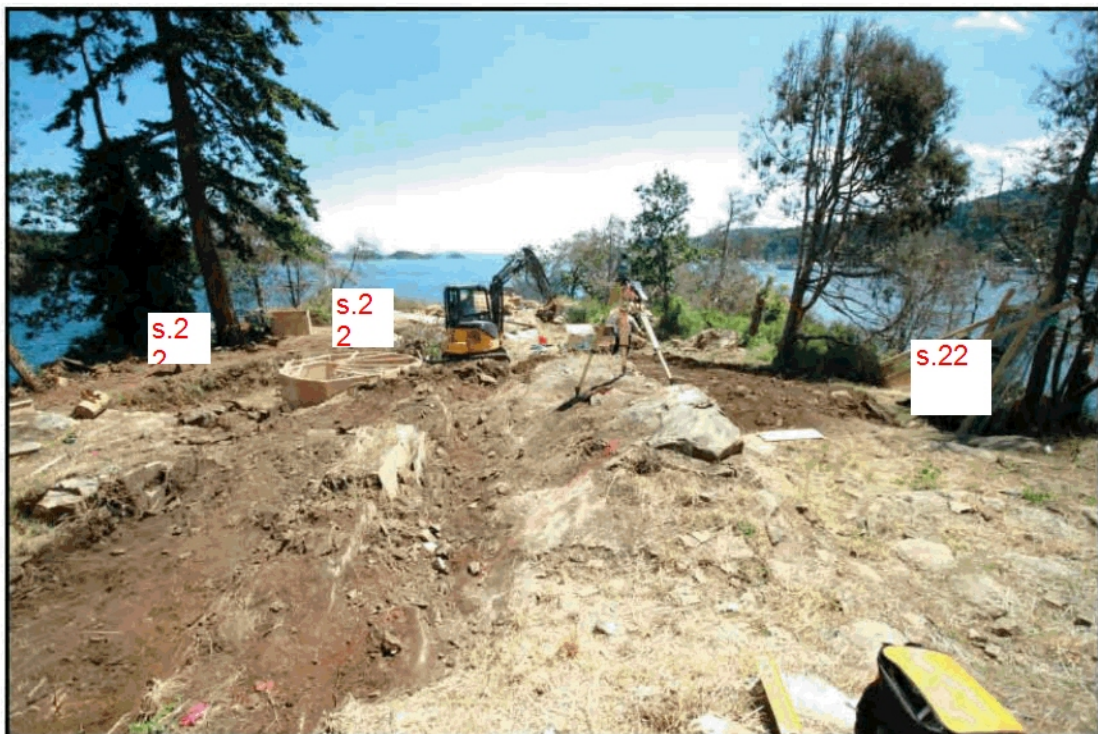
Figure 10. Picture showing the scraping of the soils and grasses covering the parent sandstone rock. All soils and littermat/duff were removed from the surface down to the parent material.
