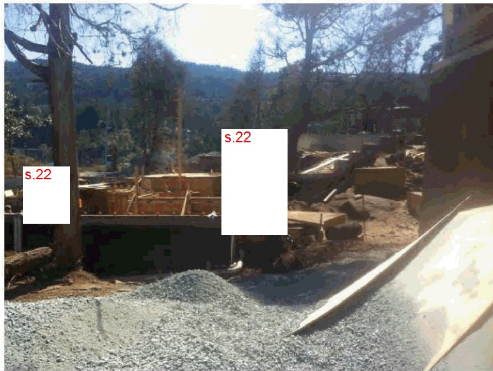
Figure 22. Crushed rock shown in the foreground was placed around foundation periphery using a backhoe and wheel barrows.
