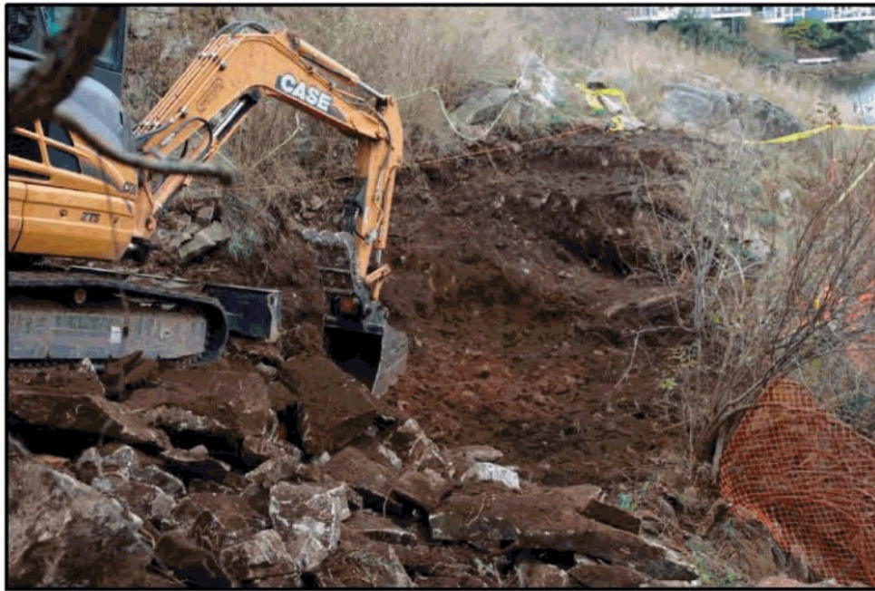
Figure 31. Clearing of overburden along access route for entrance ramp. Unconsolidated soil and rock debris was removed down to parent rock and gravels.
