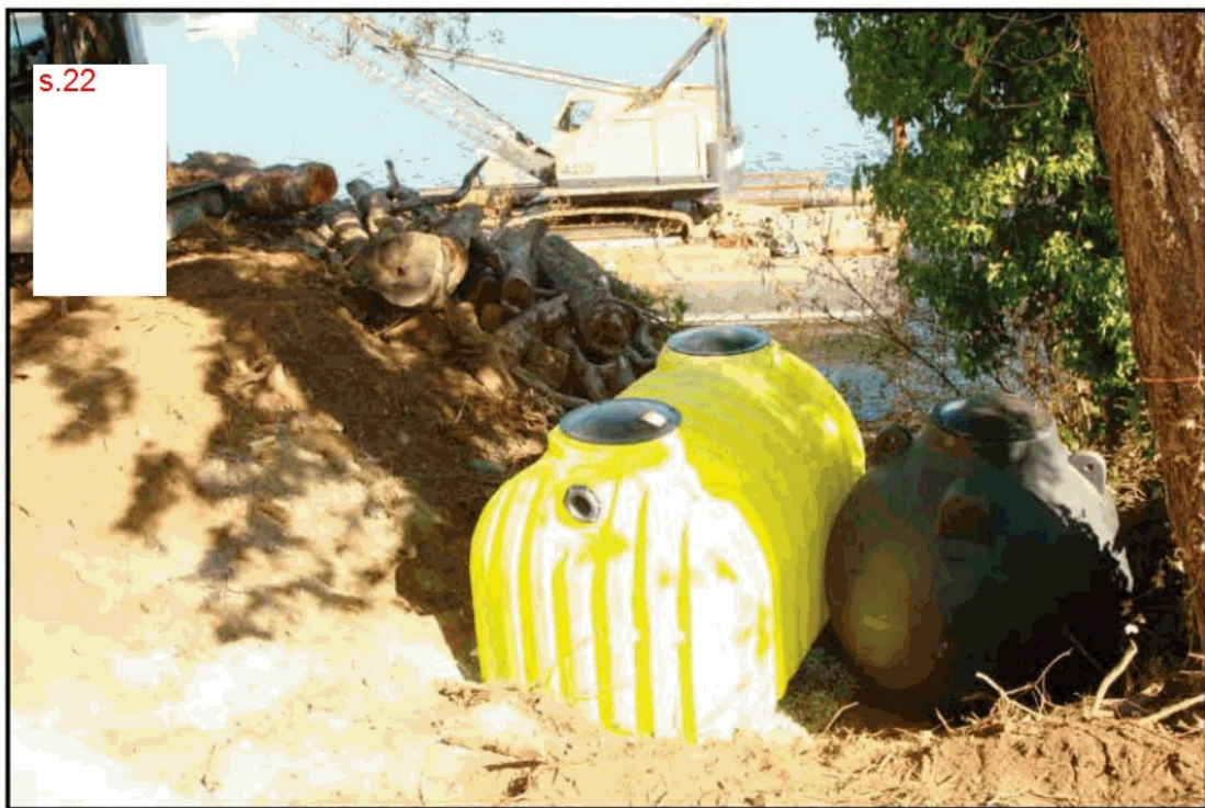
Figure 30. Water and sewage containers placed in excavated area.
