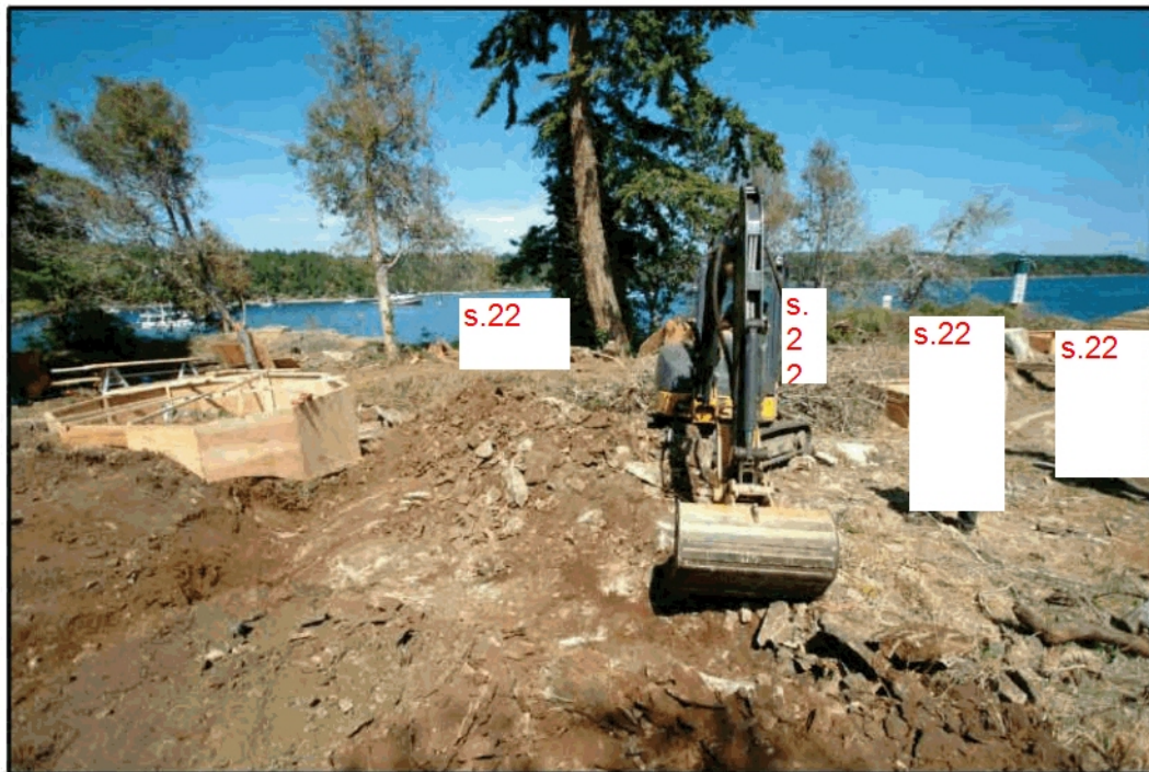
Figure 11. Picture showing the clearing ongoing (June 4, 2014). All soils and littermat/duff were removed from the surface down to the parent material.
