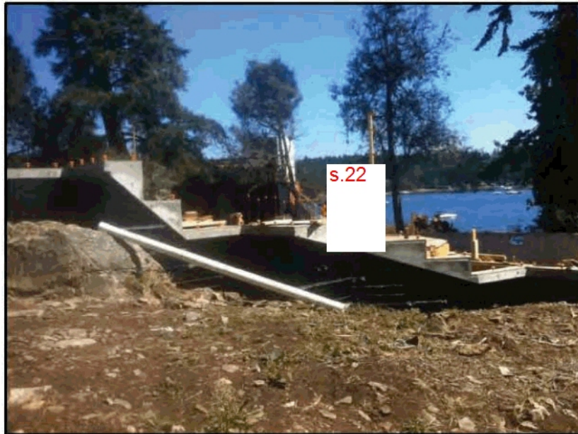
Figure 20. Monitoring was undertaken on July 29, 2014 to facilitate the installation of weeping tile (foreground) around the outside edge of the foundation.
