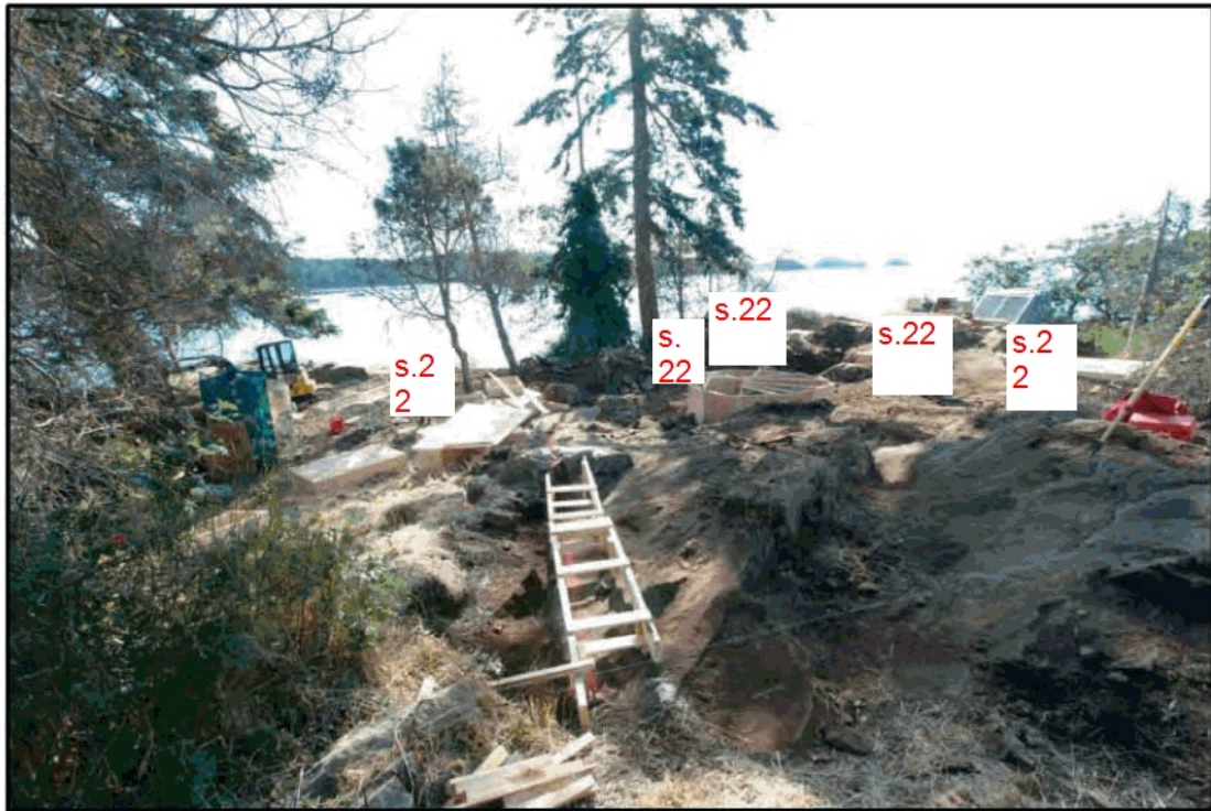
Figure 17. Picture showing the status of the construction on the morning of Friday June 6, 2014. Box enclosures were all but complete, exposure of parent rock almost complete. The last remaining area being along the northeast side in the area of a previously excavated trench. The start of the foundation forms are shown in the center of the picture.
