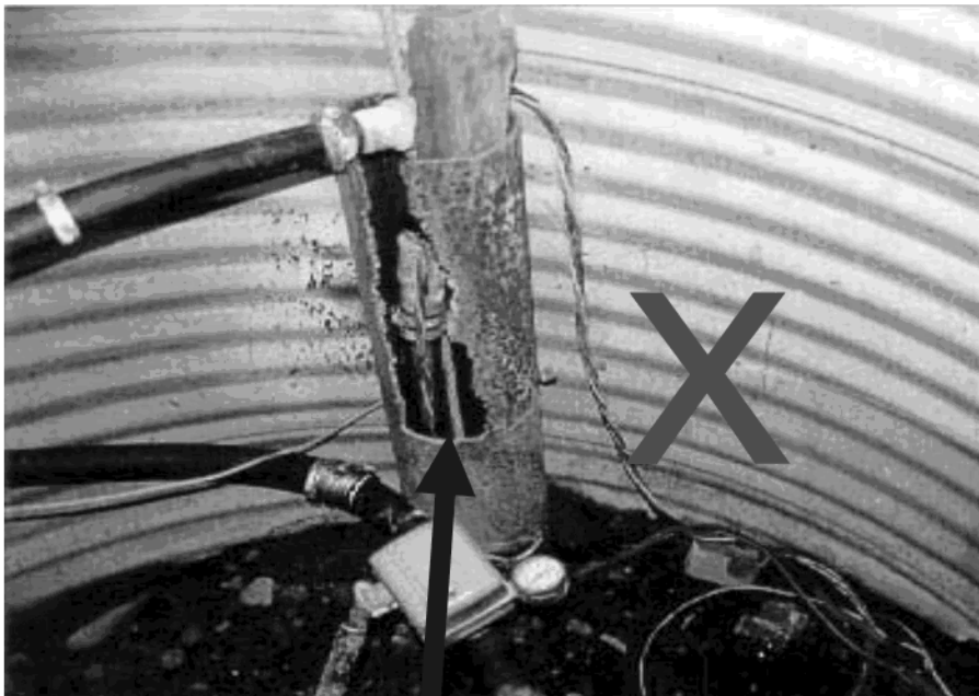
Well Casing deliberately cut to drain flood water
