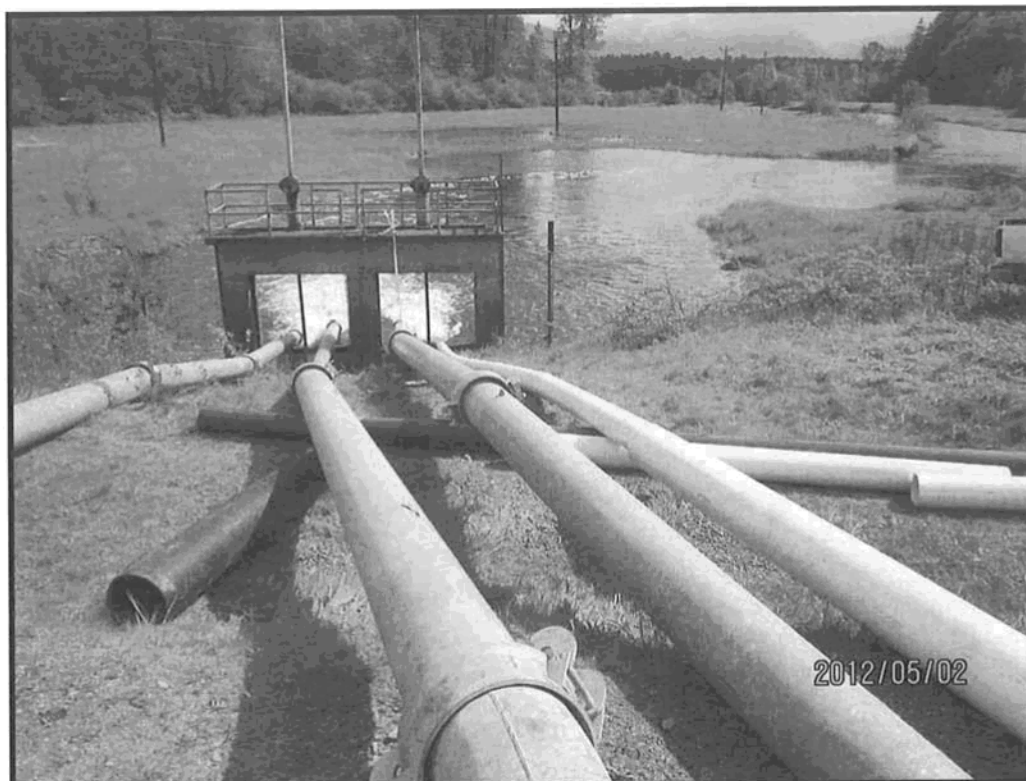
Photograph 5. Emergency Pumps Discharging downstream of the Hammersley Pump Station (May 2, 2012)
