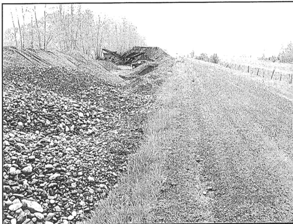
Photograph 4. West view of gravel stockpiled against the dike (April 27, 2011)
