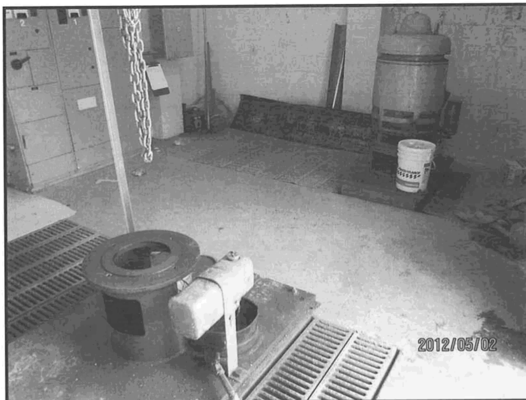
Photograph 6. Looking inside Hammersley Pump Station with 125 hp pump removed; 50 hp pump is still in operation (May 2, 2012)a
