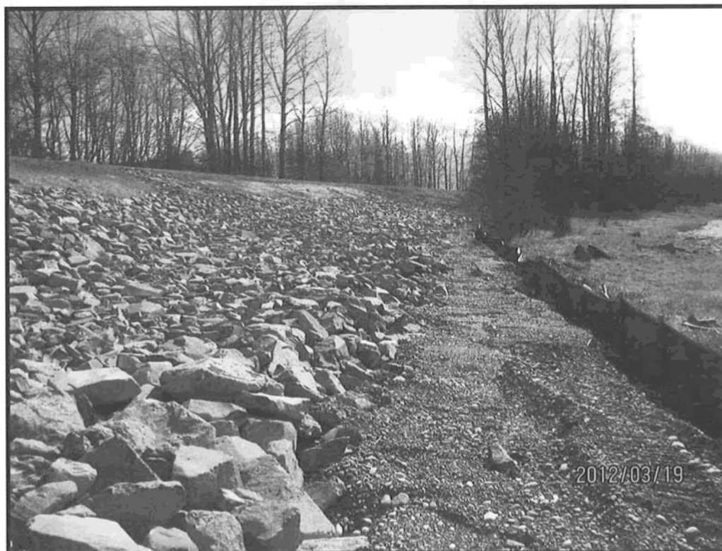
Photograph 2. South view of rip rap work performed on Dike D to combat erosion (March 19, 2012)
