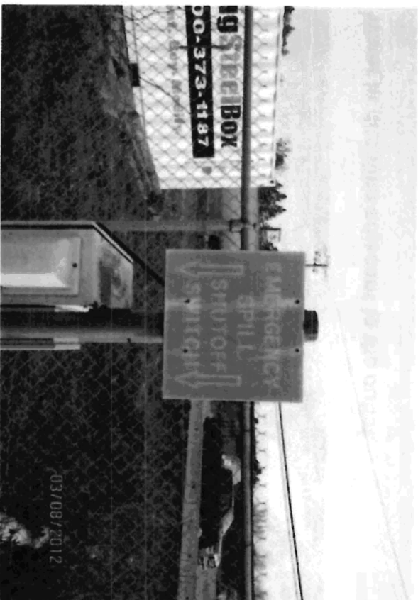
Emergency shut off switch for the oil water separator. There is also a manual shut off valve.
