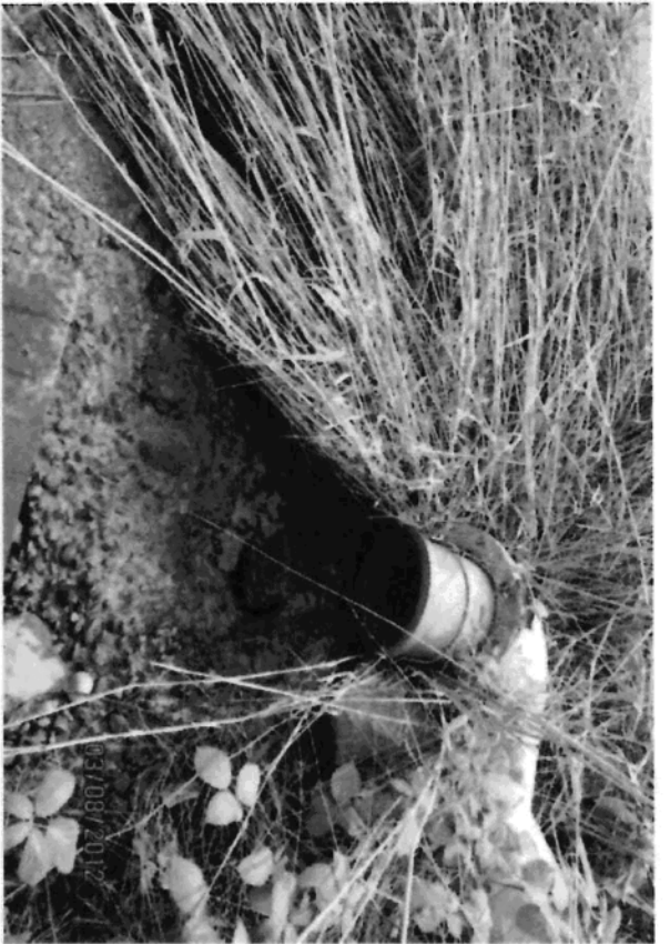
Oil water separator outlet to the environment, ditchline along Lickman Road.
