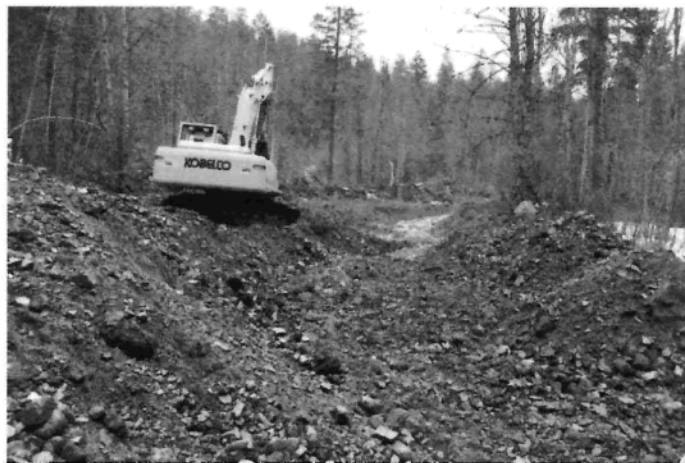
Photo 2. New channel being constructed.
