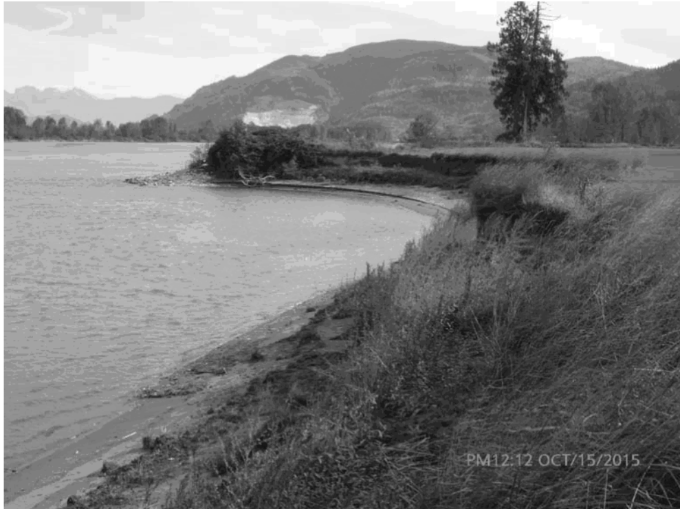
Figure 18: Dyke - Station 95+00 – One of the Erosion Arcs
