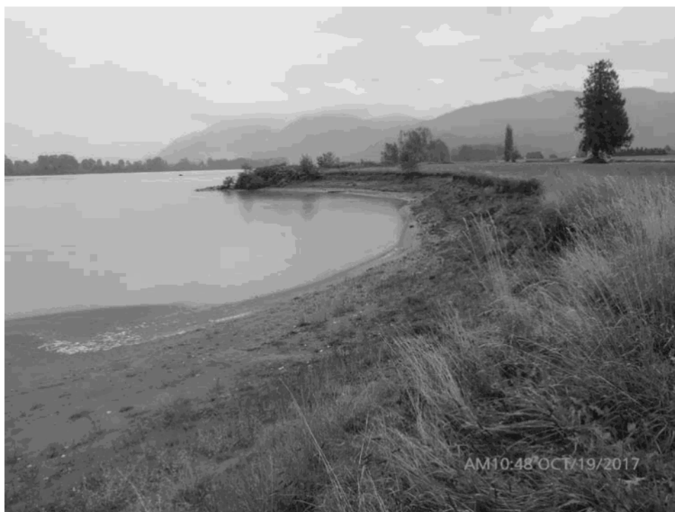
Figure 18: Dyke - Station 95+00 – One of the Erosion Arcs
