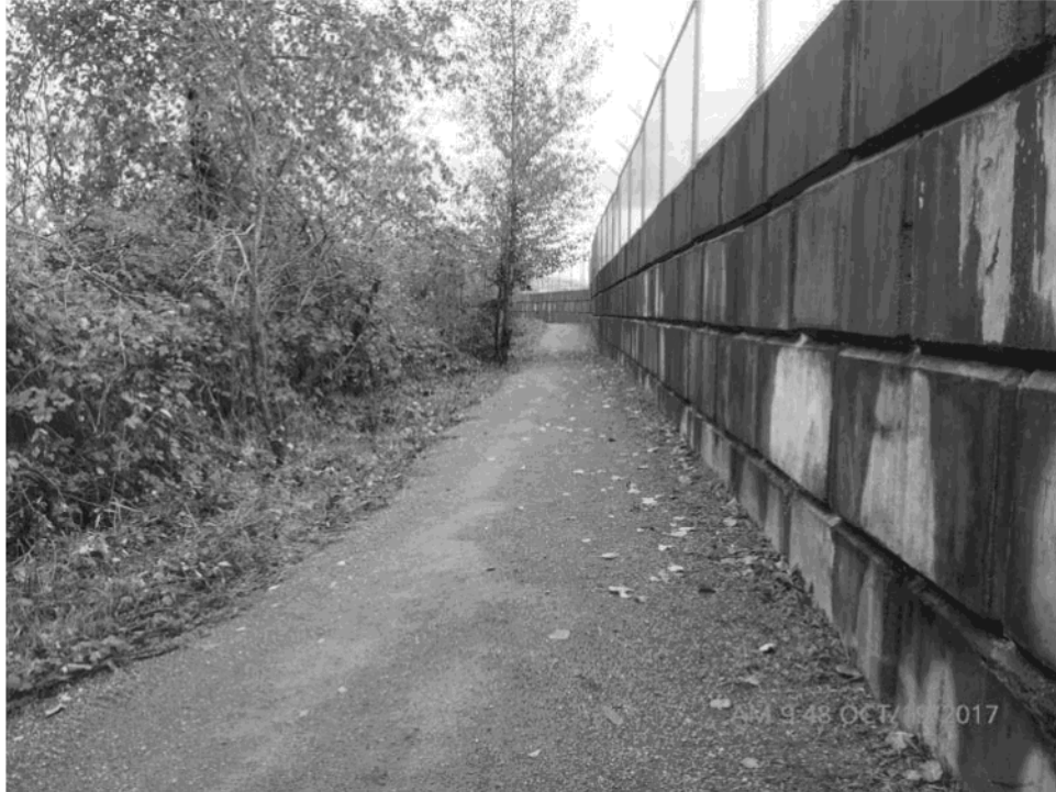
Figure 9: Lock Block Section of Dyke - Station 33+50
