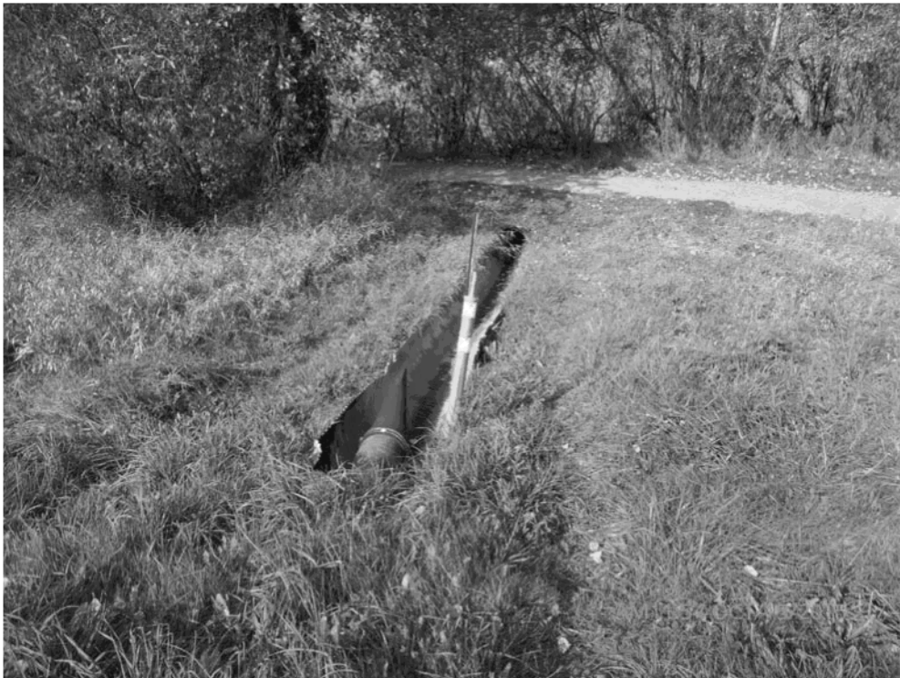
Figure 32: Vanderloo Pump Station - Tide Flex Valve - Station 65+00
