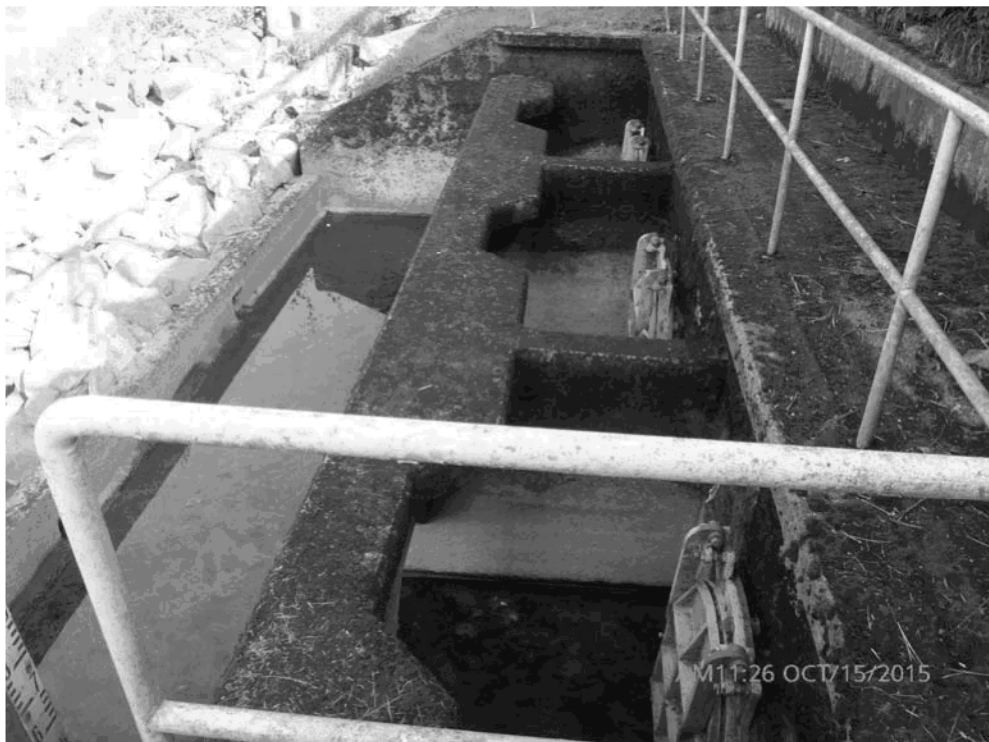
Figure 28: Matsqui Station Flap Gates - Station 34+50
