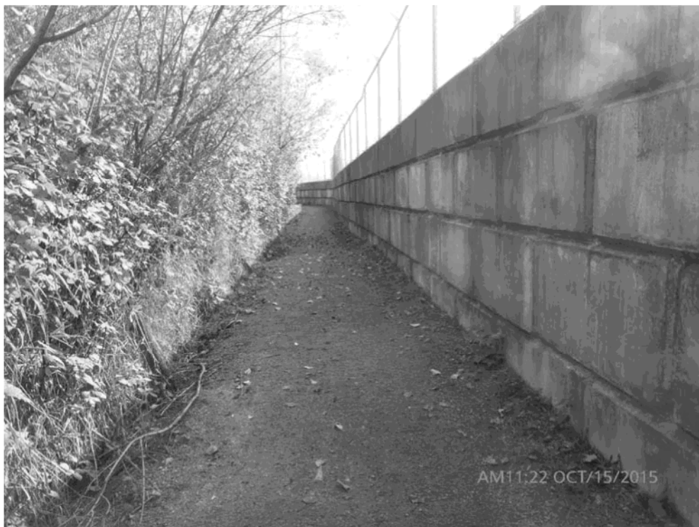
Figure 9: Lock Block Section of Dyke - Station 33+50
