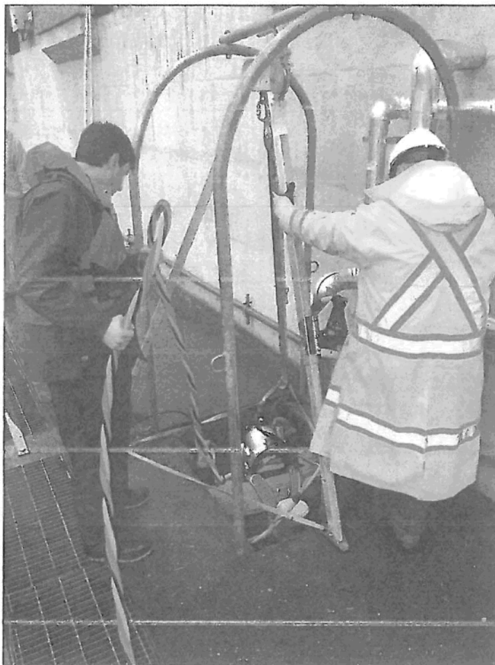
Ref.8 One of three stop log sections being lowered in place. Diver waits by ladder until stop log lands on bottom.
