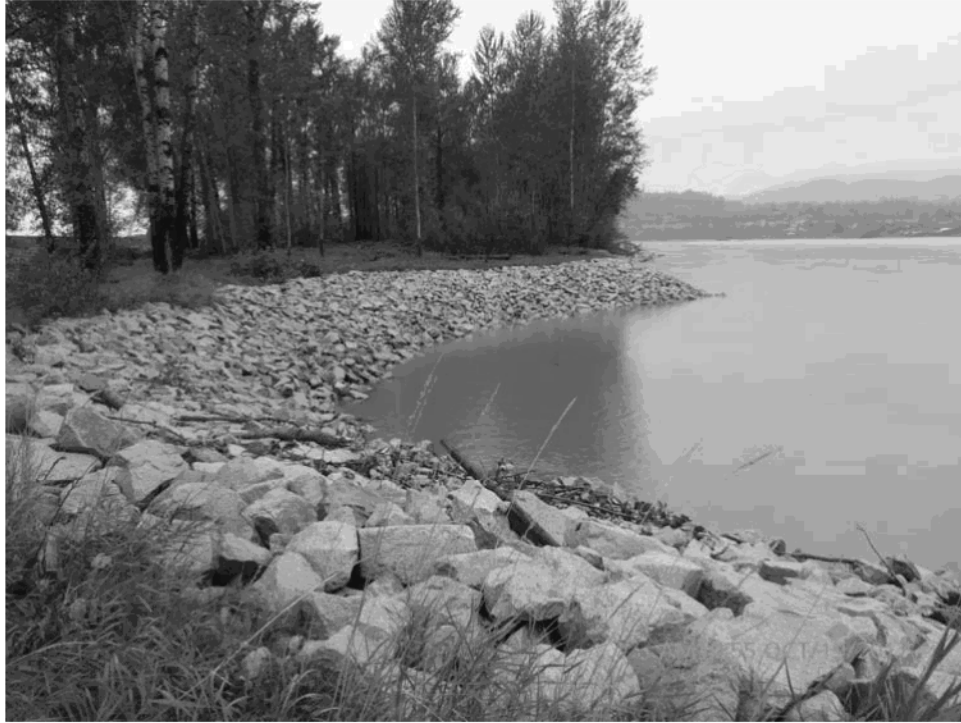
Figure 21: Dyke - Station 110+00 – One of the Erosion Arcs
