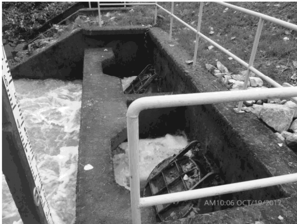
Figure 224: McLennan Station Flap Gate - Station 18+50
