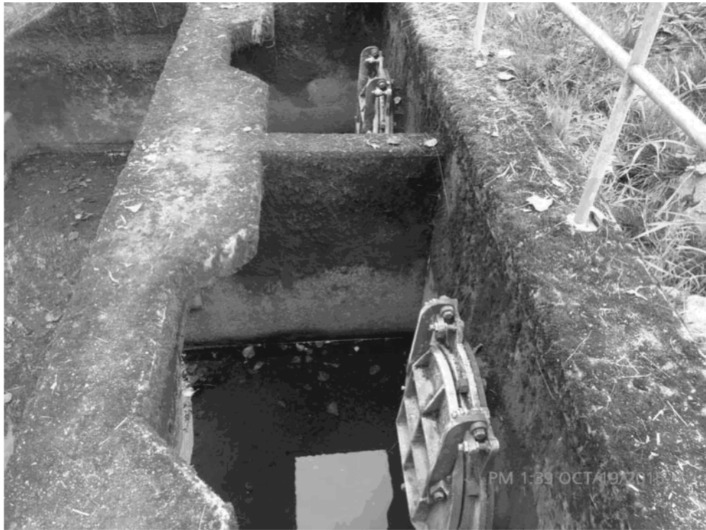
Figure 23: McLennan Station Flap Gate - Station 18+50
