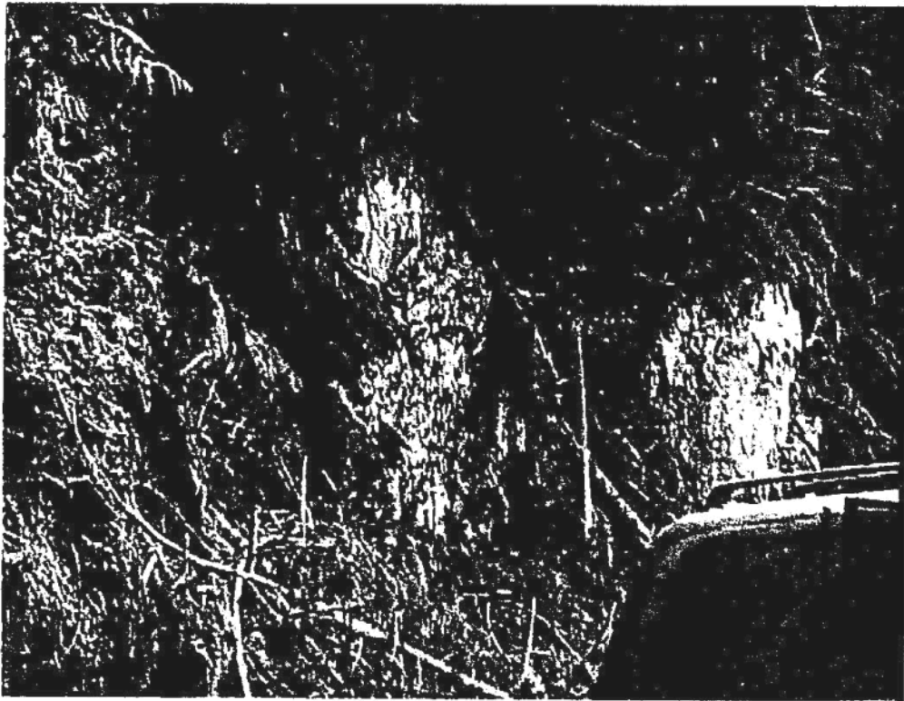
Photo 8. Unstable cut slopes with highly fractured rock.
