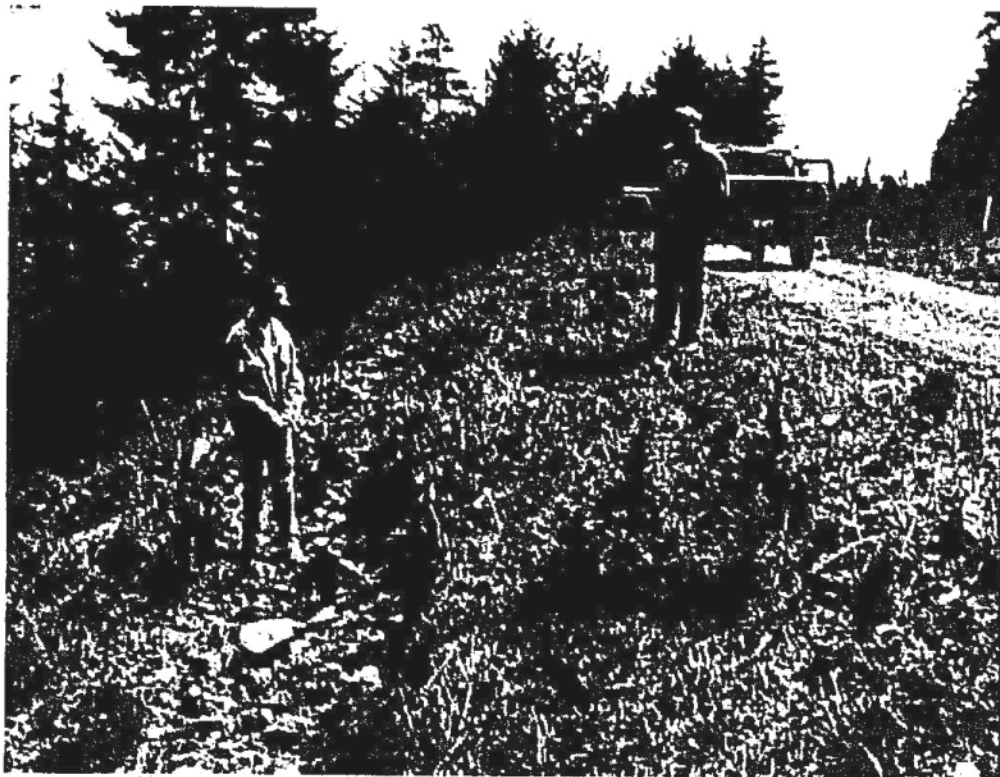
Photo 4. Tension crack approximately one metre drop.
