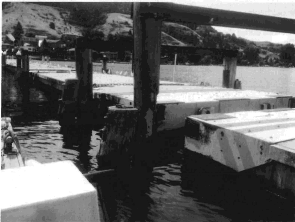
Photo 4. Looking at the damage done to the concrete breakwater floats west of the marina during the July 2014 storm (photo submitted by client)
