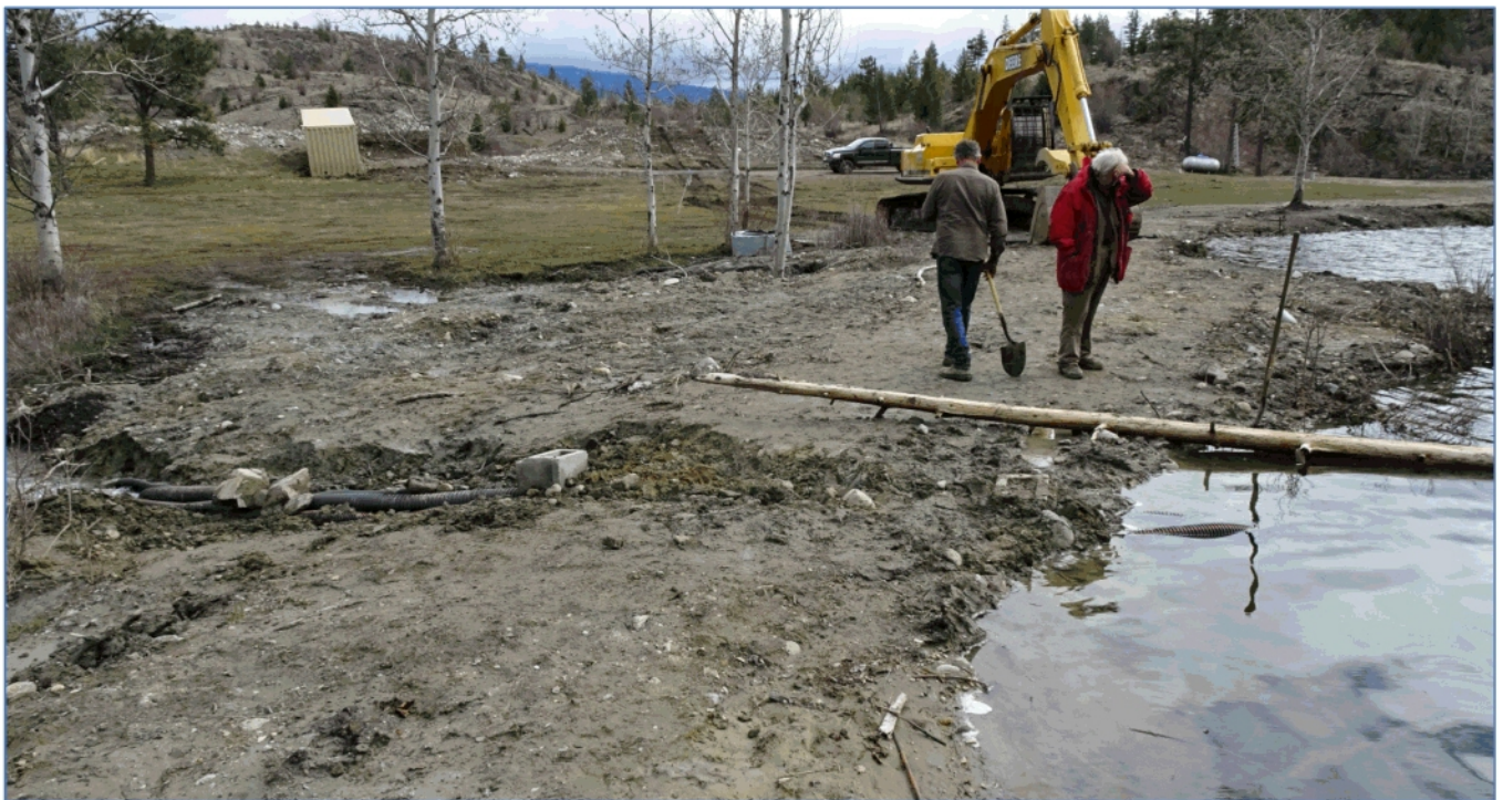
Photo 6. Hand excavated trench with plastic pipe.
