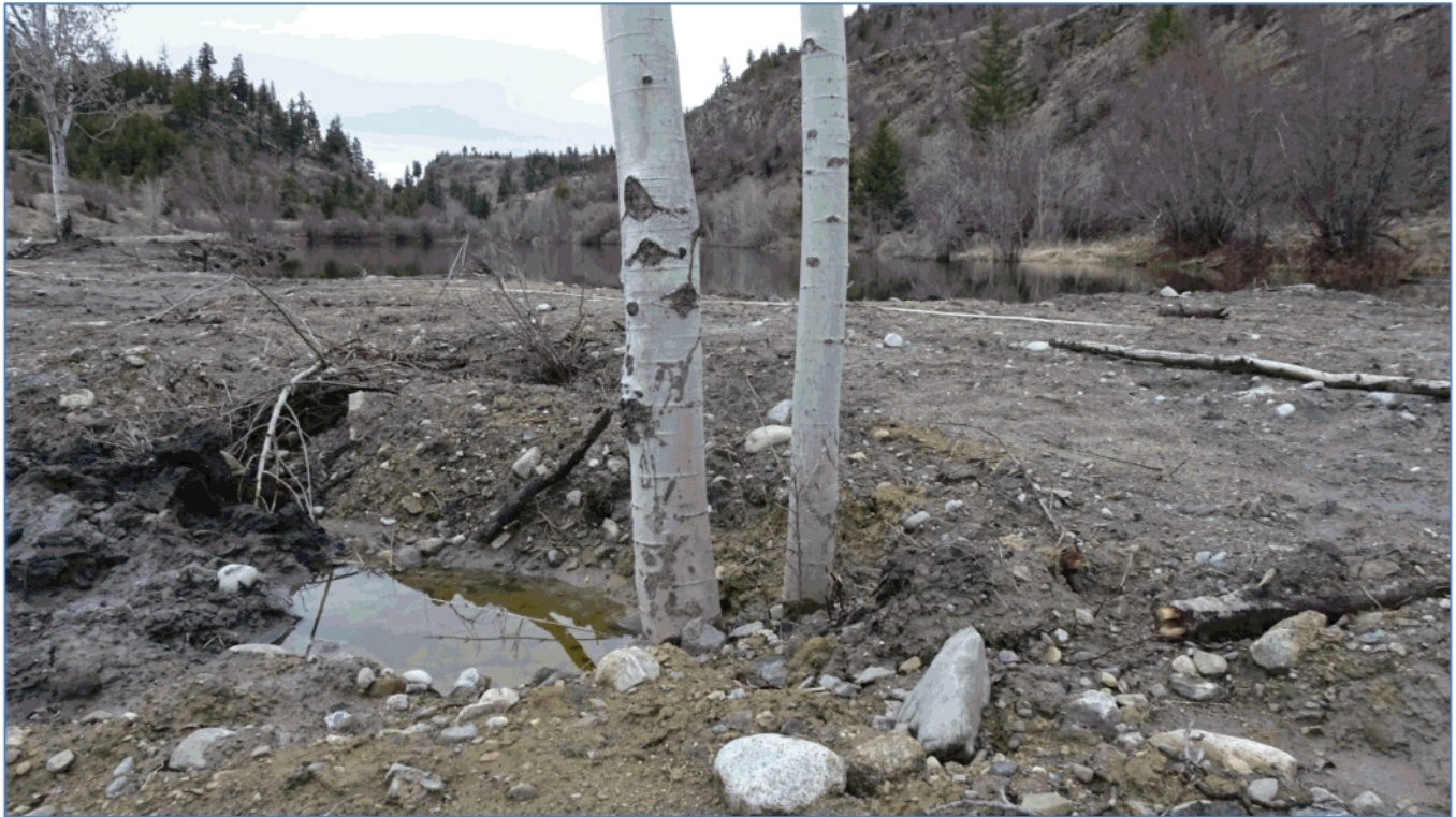
Photo 3. Dam appears to be 1-2m in height. Note partially buried trees.
