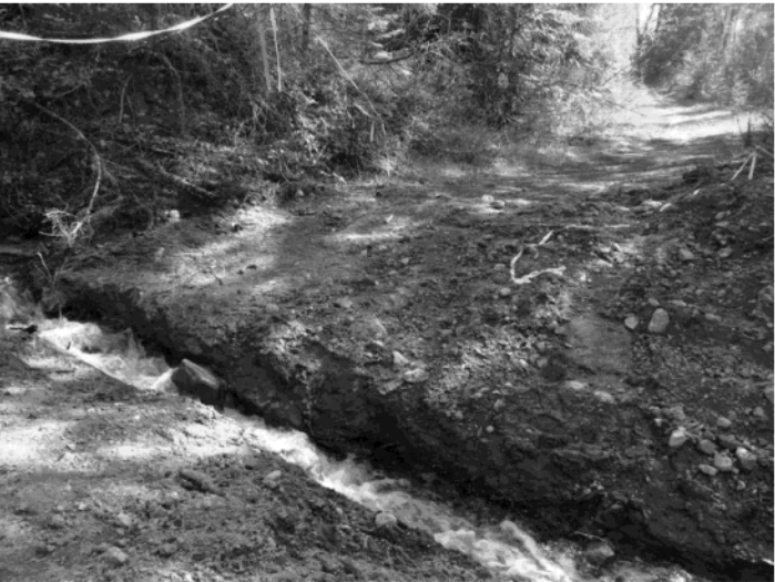
Photo 3 – Cross-drain culvert removed at Wpt 201.
