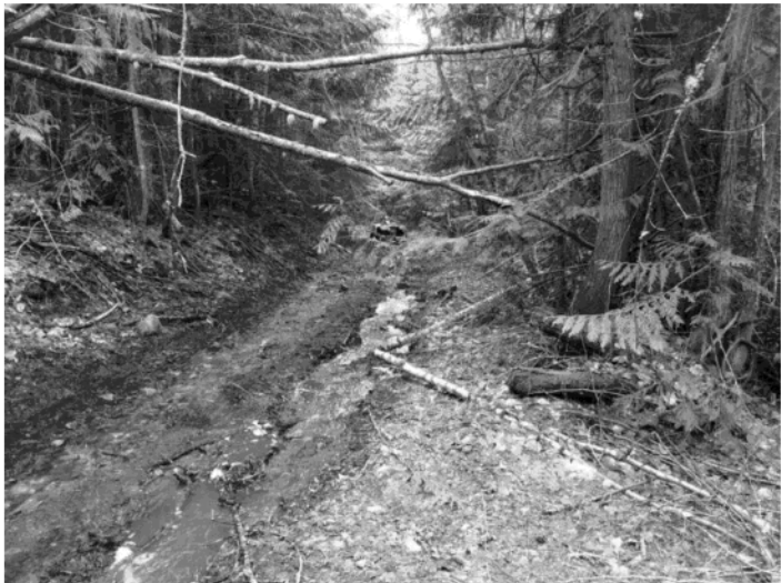
Photo 18 – Road surface erosion between Wpt 1000 and 1005.
