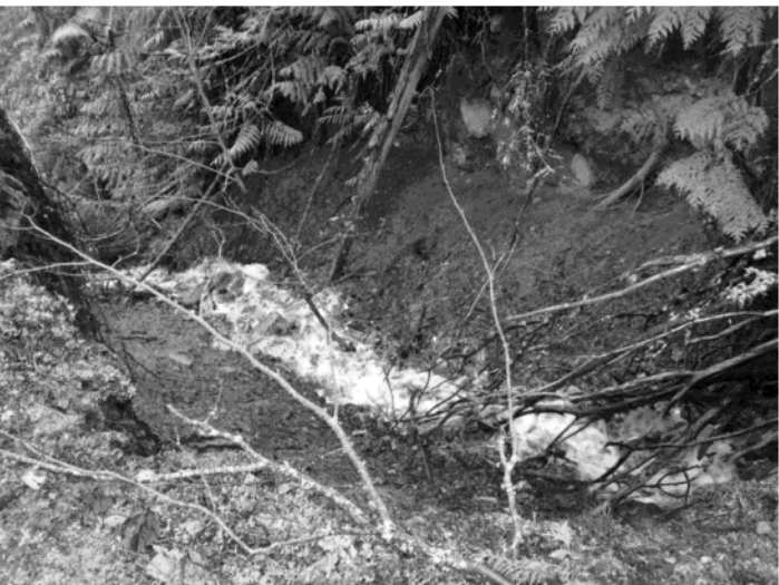
Photo 16 – Eroded take-off ditch at Wpt 149 drains into Gully A.
