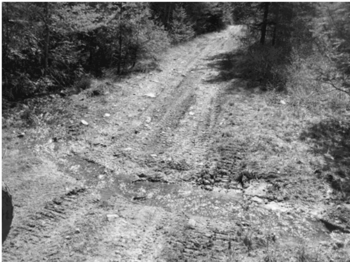
Photo 9 – Cross-ditch at Wpt 169 drains to Slide 2 headscarp. Photo taken May 1 and faces towards town.
