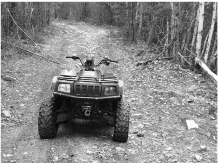
Photo 14 – Road surface erosion between Wpt 137 and 139 suggests drainage was likely diverted along the FSR prior to removal of the culvert at Wpt 137. Photo is located at Wpt 139 and faces towards the bush.
