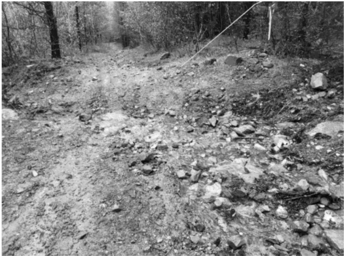
Photo 13 – Culvert recently removed at Wpt 137. Significant road surface erosion noted towards town.
