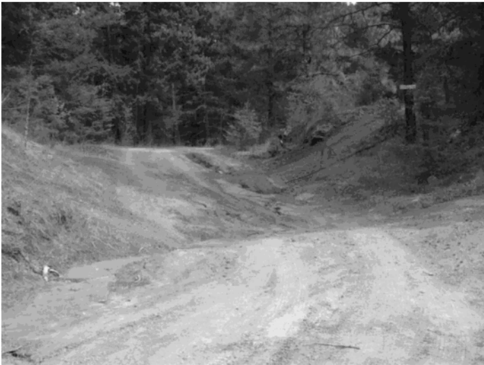
Photo 2 – Surface erosion at Wpt 629.
