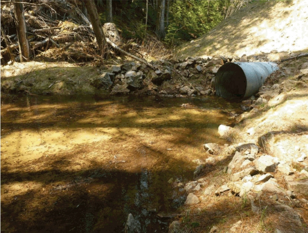
Photo 3. Intake of culvert from right bank
