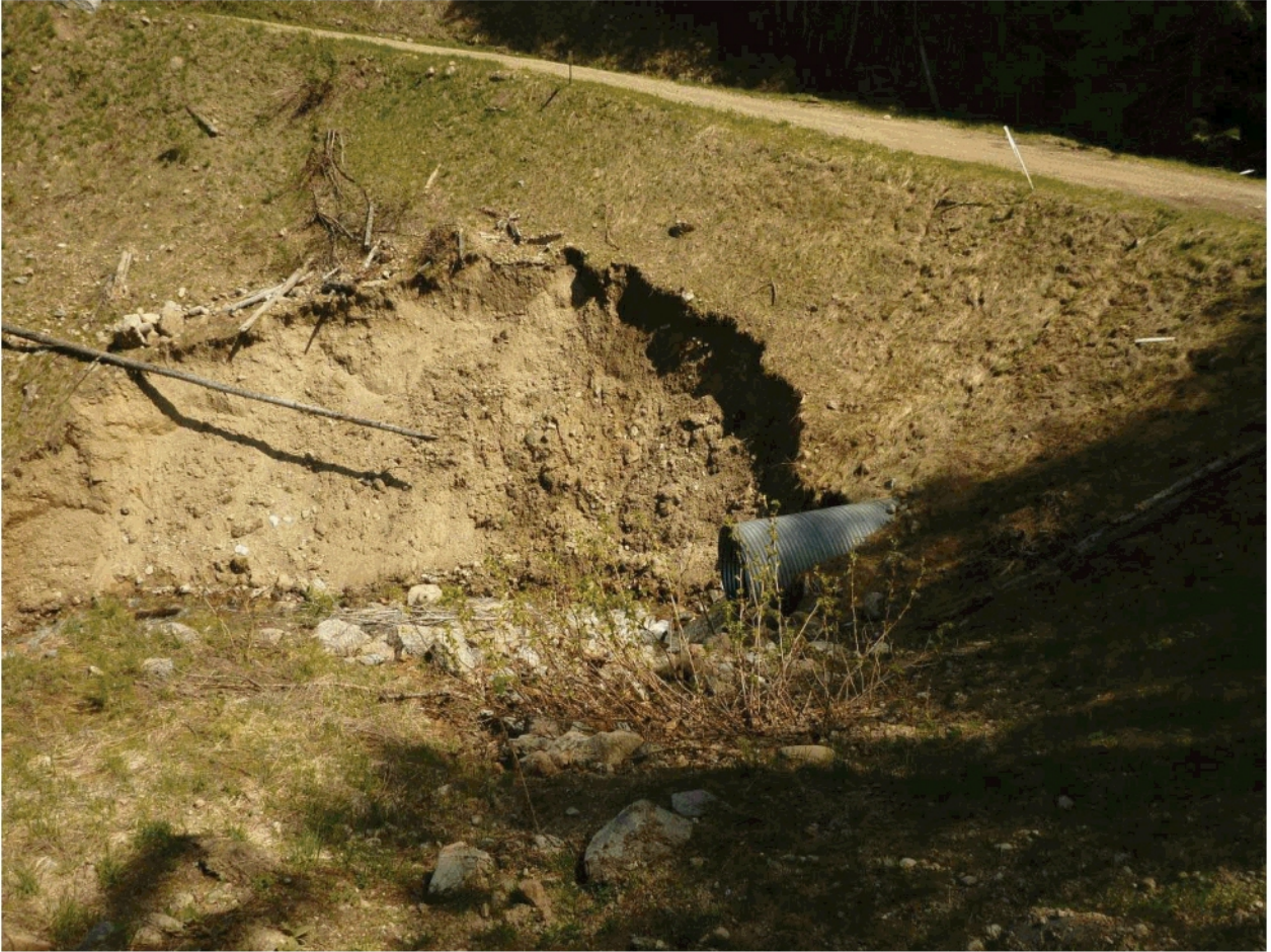
Photo 6. View of scour from bank on west side. No tension cracks were observed on the fill above the scoured area.
