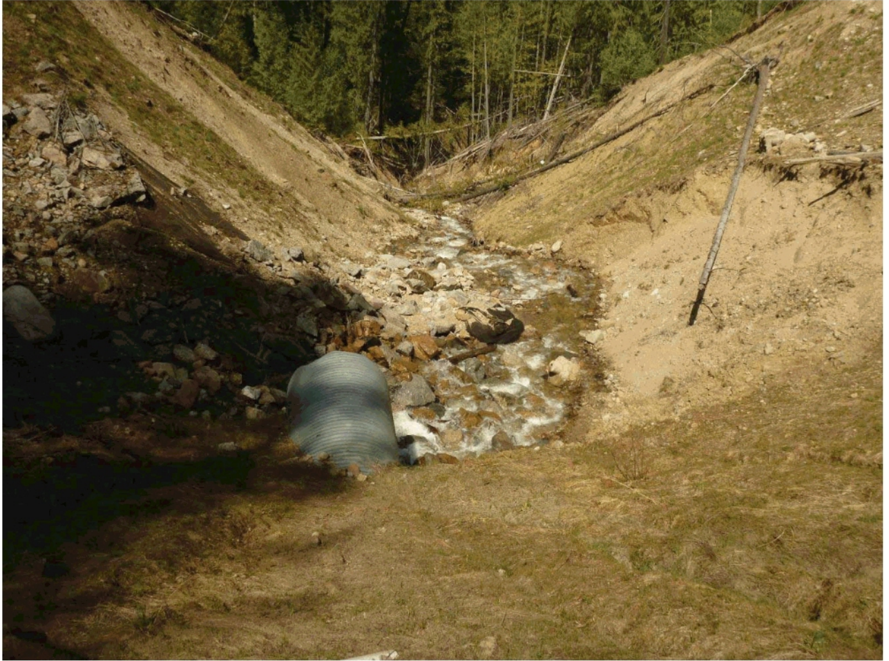
Photo 2. View of outlet on May 15, 2018. The bank on the left has slumped down over the past 5 years causing rock armour to divert the flow of the stream into the opposite bank. Riprap on the right bank is gone and needs replacing.
