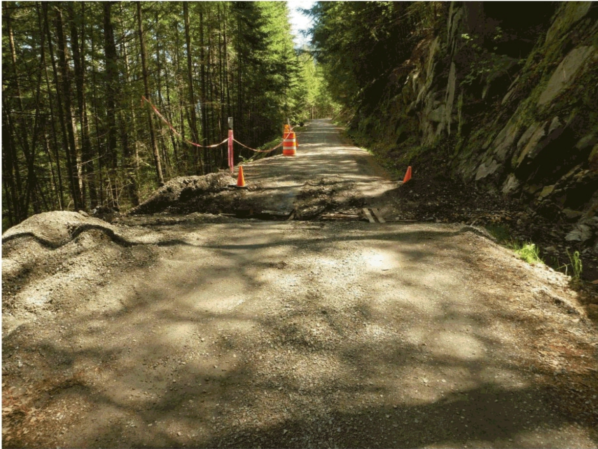
Photo 5. View of waterbar and rock bluff to the east. Note the safety warnings and straight horizontal alignment. A sign is also posted about 30m to the east.
