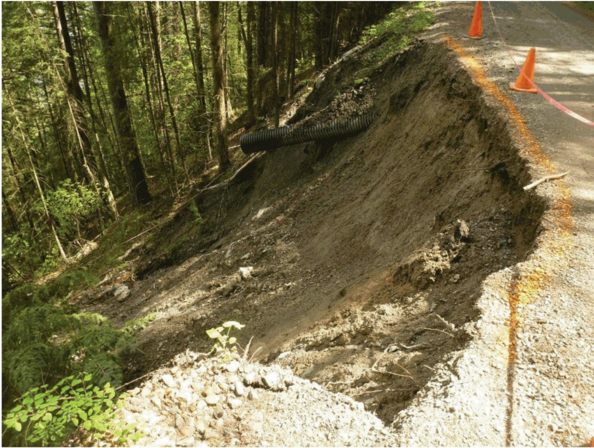
Photo 1. View of failure from west end. Note that although water coming out of the culvert may have triggered the failure, the fill material was likely saturated from seepage flowing about 30cm below the trail surface.
