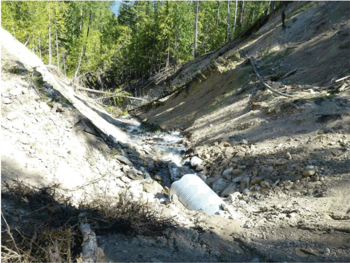
Photo 1. Outlet of culvert on May 7, 2013 shows riprap and channel properly located with straight runout of stream flow.
