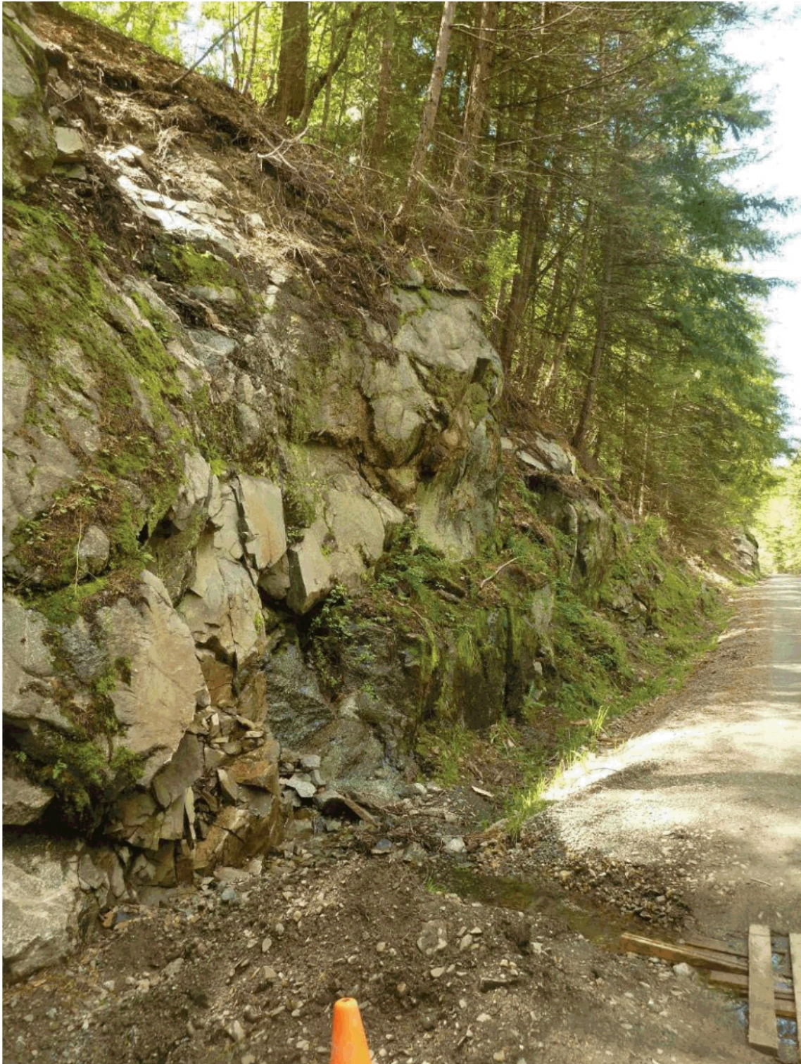
Photo 4. View of rock face on west end of section, showing the recently installed water bar. This is where the most runoff from above the rock occurred. The culvert was installed about 10m downgrade to the east because of solid rock underneath the trail at this point.
