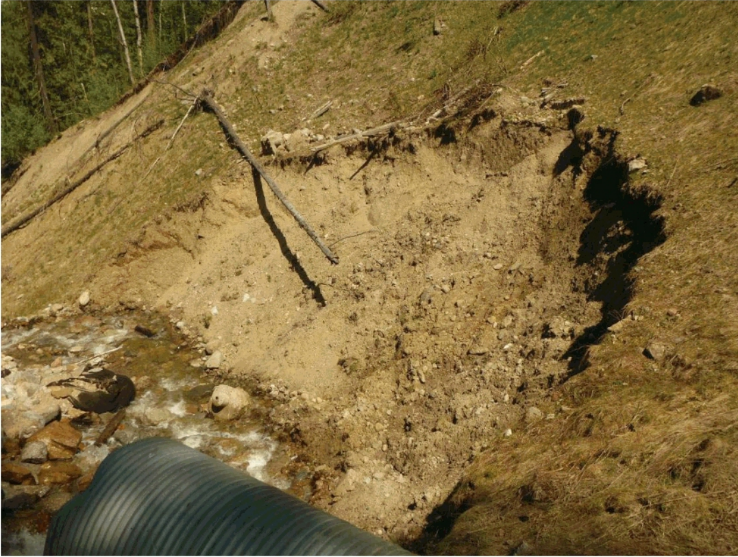
Photo 5. View of scour from outlet.
