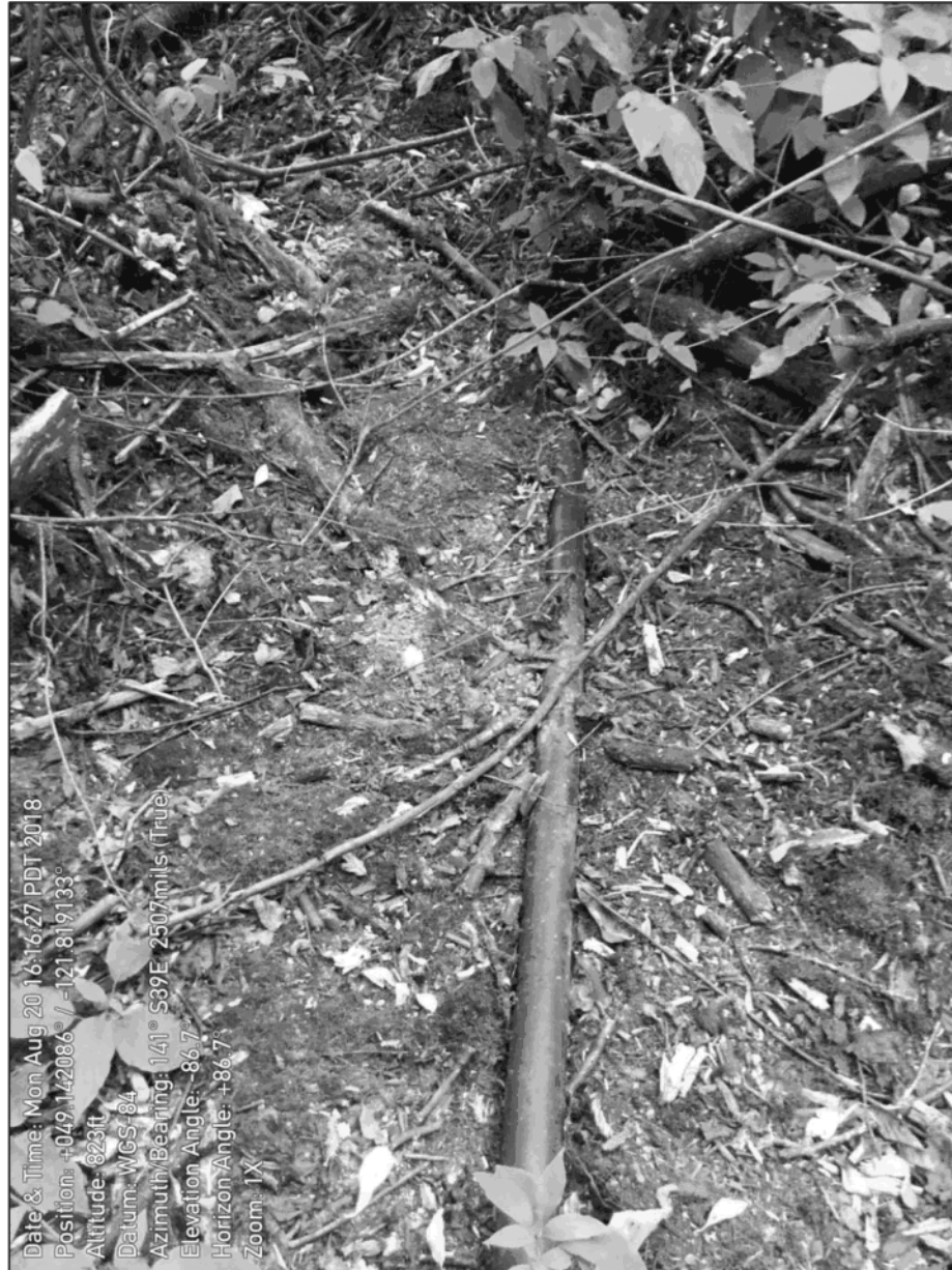
IMG_0280: Southern section of original water main line partially exposed to the surface
