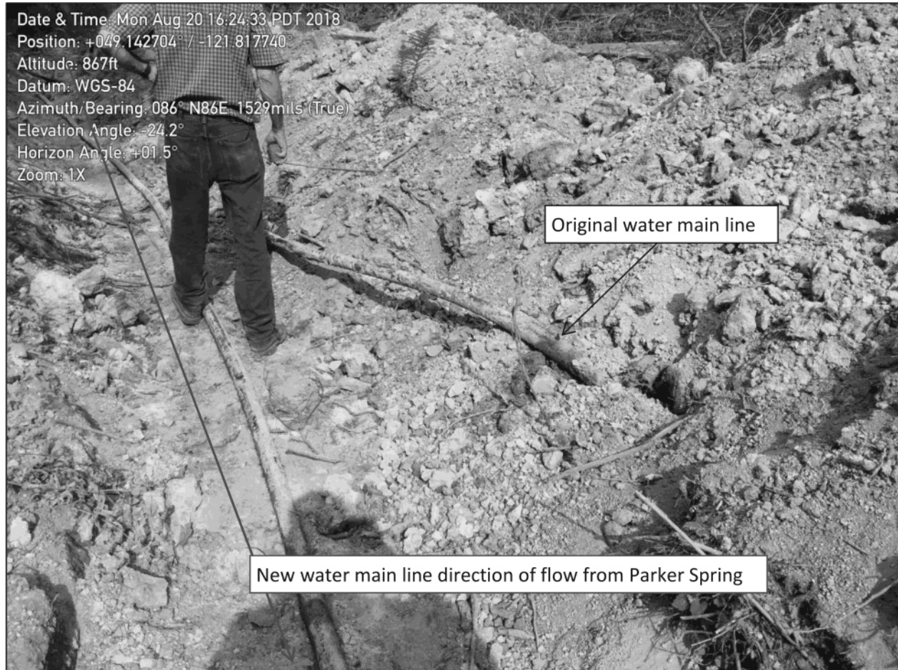
IMG_0284: Original water main line adjacent to the new water main line replaced by DICKEY.
