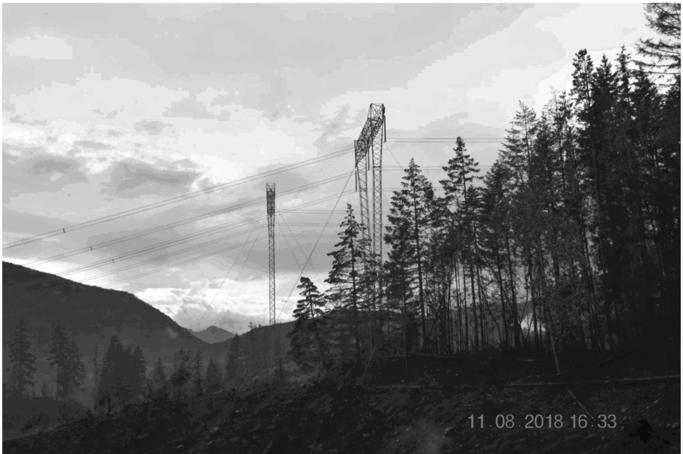
Figure 17: Powerlines were located approximately 83 m to the west of the origin area. Investigators observed no damage to the powerlines, insulators or towers. Fire spread indicators showed the fire did not originate at the powerlines (TAB 10 PHOTOS MORRISON FOC DSC_0934).
