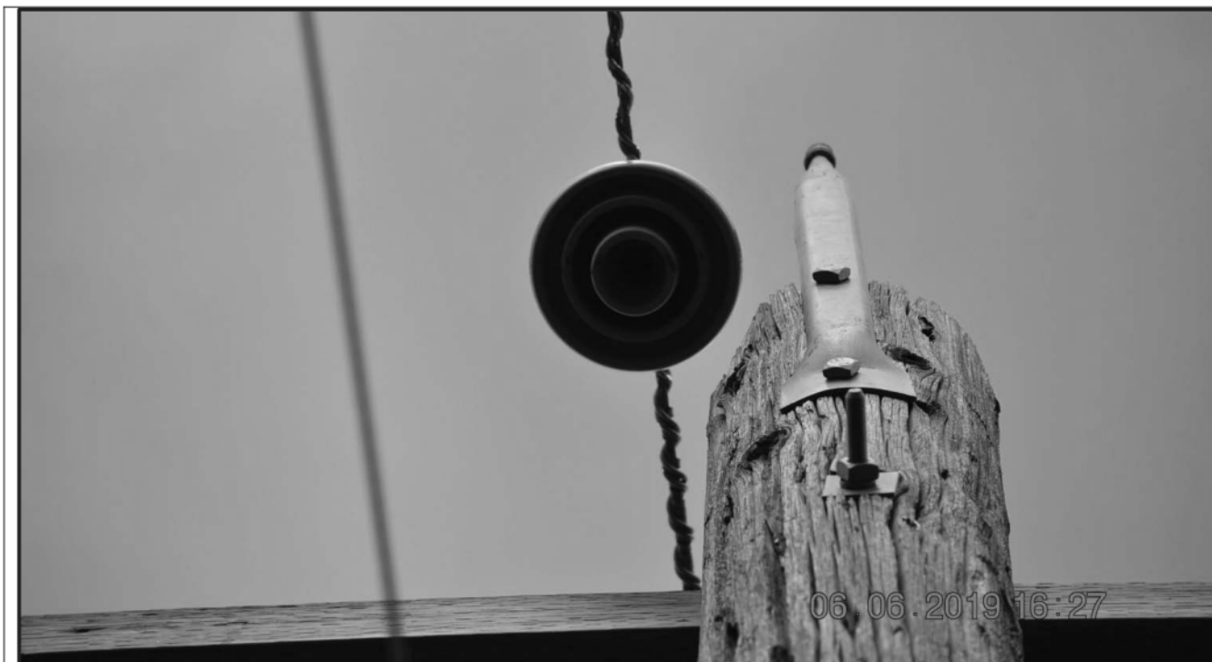
Figure 12: View from below of the insulator dislodged from its support post on Pole 13 (TAB 9 DSC_0120).
