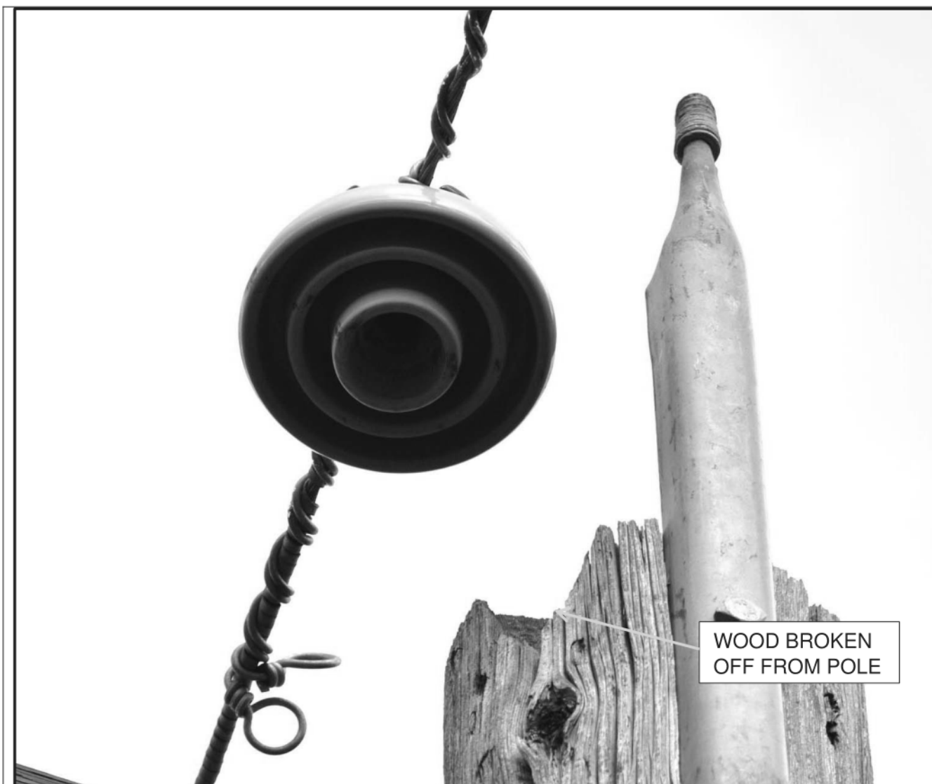
Figure 9: The wood of Pole 13 was old and weathered. A piece of wood had broken off (TAB 9 DSC_0012).
