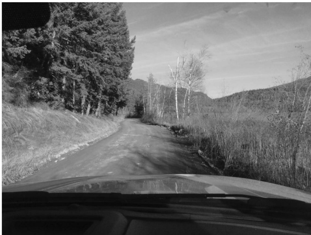
Fig.3 – Photo of proximity of road adjacent to White Lake – causing excessive siltation in Spring and wet conditions being so close to Lake edge.
