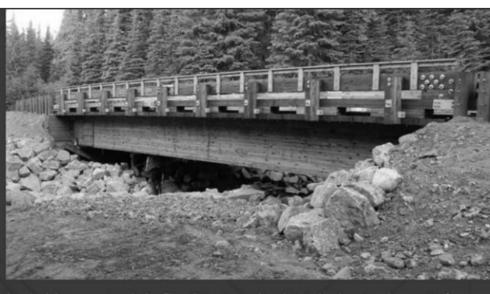
overlain with a laminated subdeck and solid sawn running planks. The substructure and crash-tested curb system also consist of glulam timbers. This bridge, located seven kilometres east of Sun Peaks Resort, was designed, fabricated/pre-assembled off-site and reassembled on-site, as a demonstration of what is possible for timber bridges for BC, with durability by design concepts incorporated.
