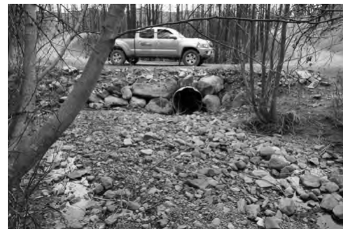
Photo 3 – Looking downstream along Shouz Creek towards the 900 mm diameter culvert under the Shouz Creek FSR. The culvert constricts the creek as it passes under the road and at high flows will back up flow. This may cause sediment deposition above the inlet which may further restrict flow.
