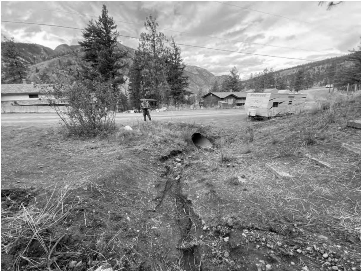
Figure 2-3. Culvert intake for Devil's Creek at Nicomen River Road. Note the travel trailer parked in the foreground and two houses downstream of the culvert in the background of the photo. Photo: BGC looking downstream (north). September 29, 2021.
