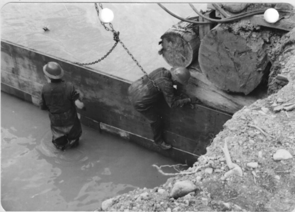
Placement of prefab forms on far side.
