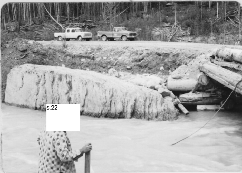
Looking to-wards near side- rock cleaned
