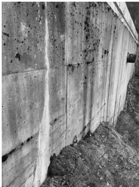
Hairline crack at top of white deposits
