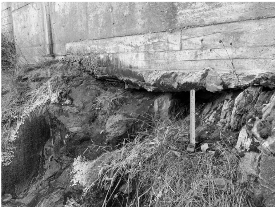
Erosion of foundation 1.5m left (upchain) of culvert.
