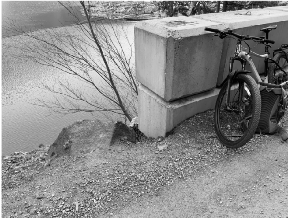
Potential surface flow erosion location
