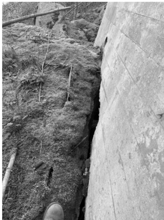
Concrete interface on large Boulder. Boulder has moved 7 inches away from wall
