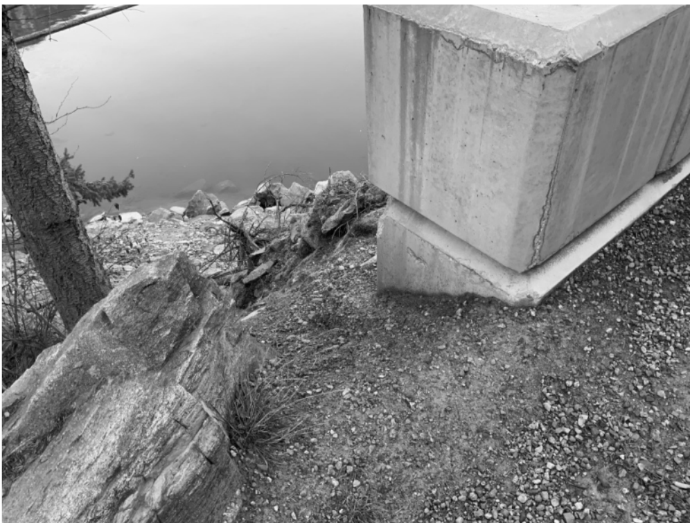
Left (up chain) side potential for surface erosion issues on lateral slope.
