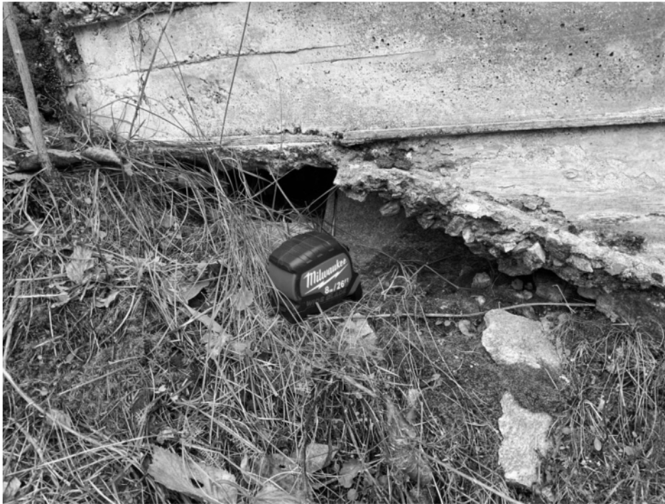
2m right of culvert plunge location, 20cm into wall, 40cm wide, 14cm high
