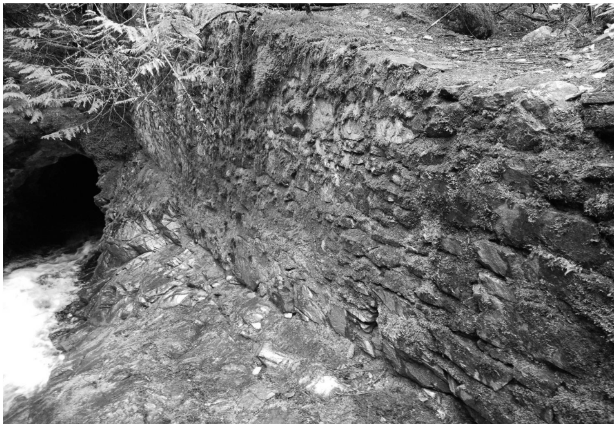
2.5m rock and mortar headwall at inlet
