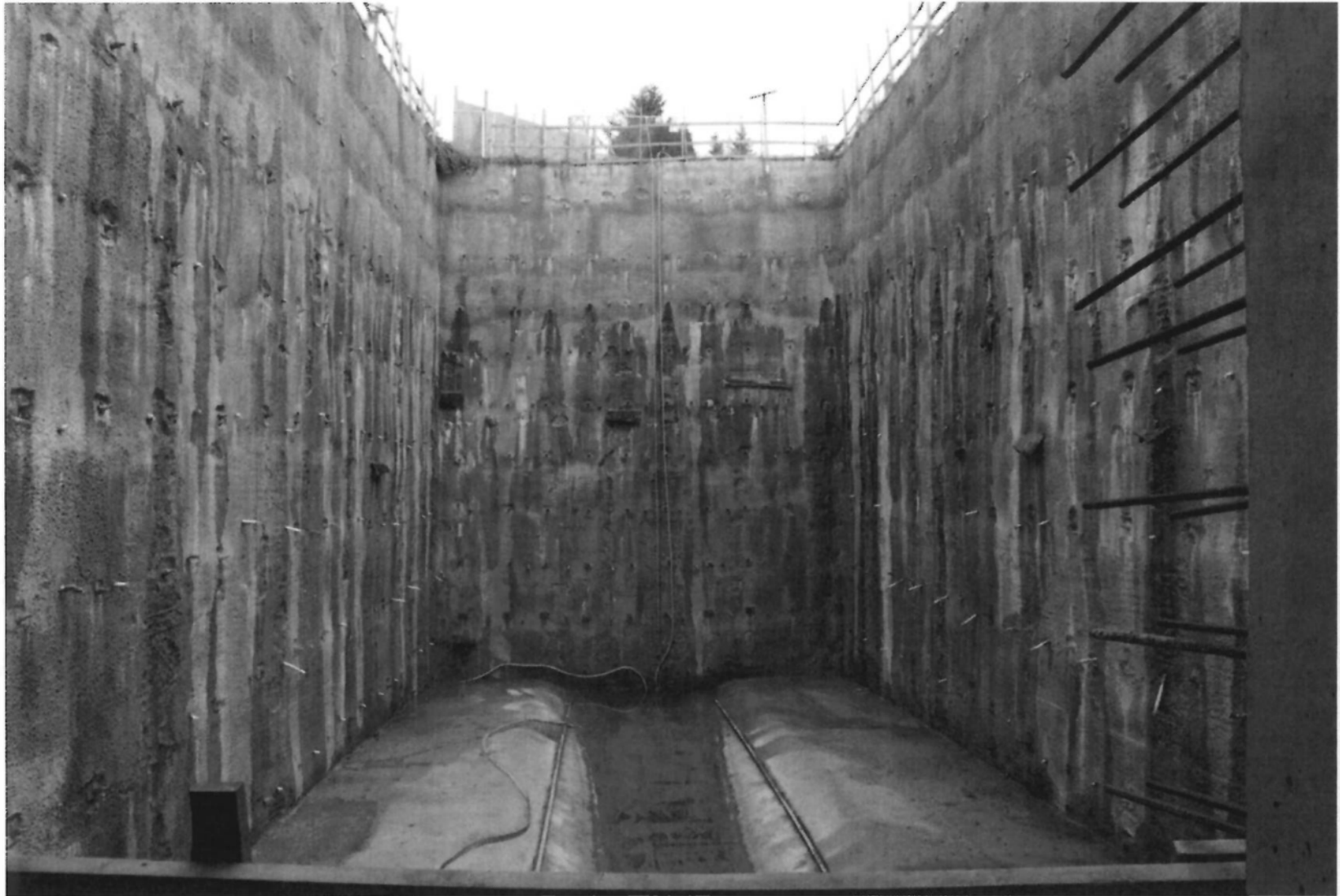
Tunnel boring machine reception pit at the south end of the tunnel in Burquitlam
