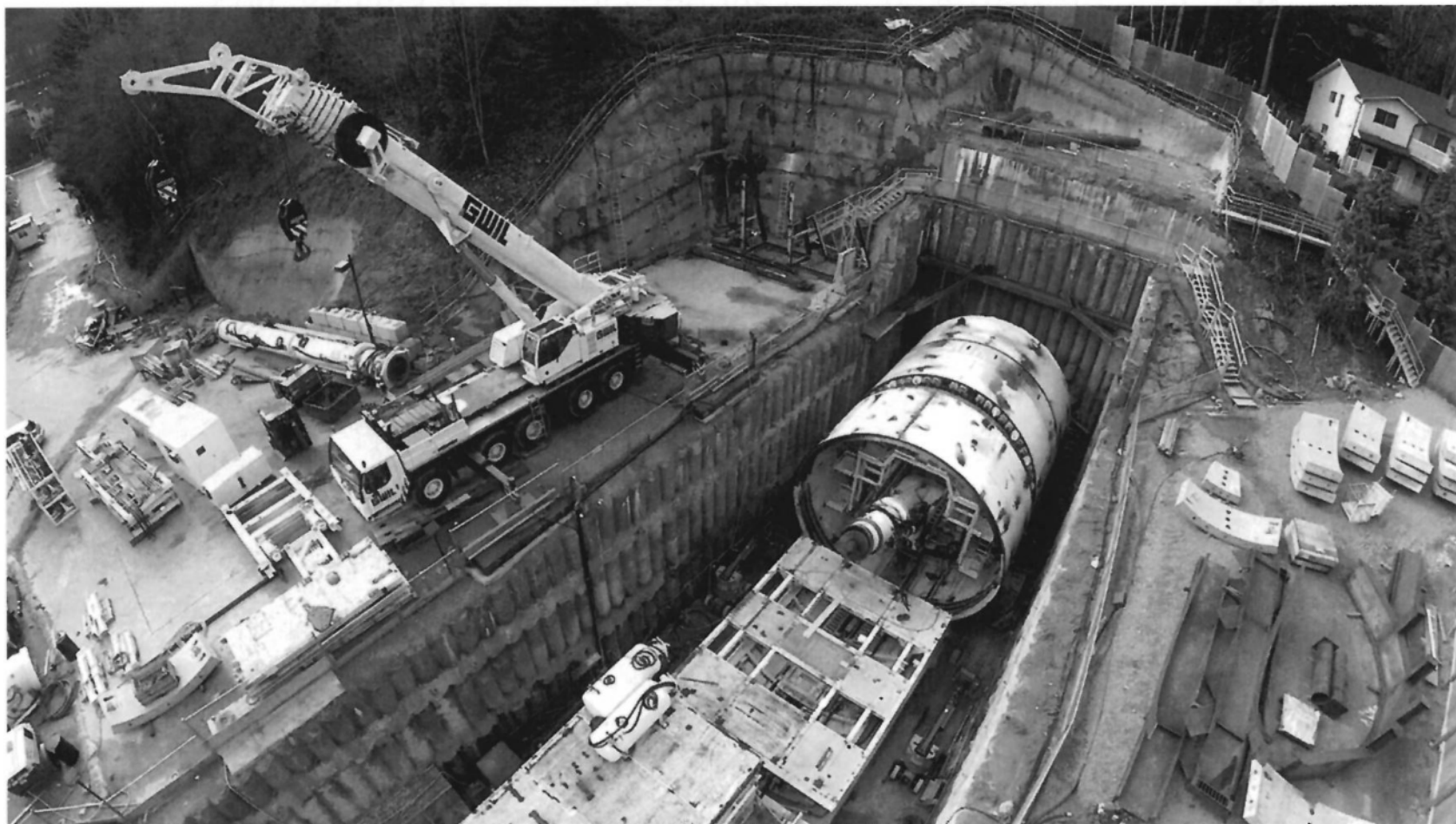
Tunnel boring machine being assembled in the TBM worksite at the start of the tunnel in Port Moody
