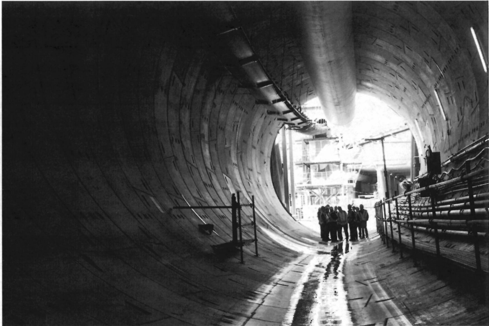
Inside the Evergreen line tunnel looking back at the start. The spoils removal conveyer belt and a ventilation system run along the top of the tunnel and electrical cables and grout piping along the side.
