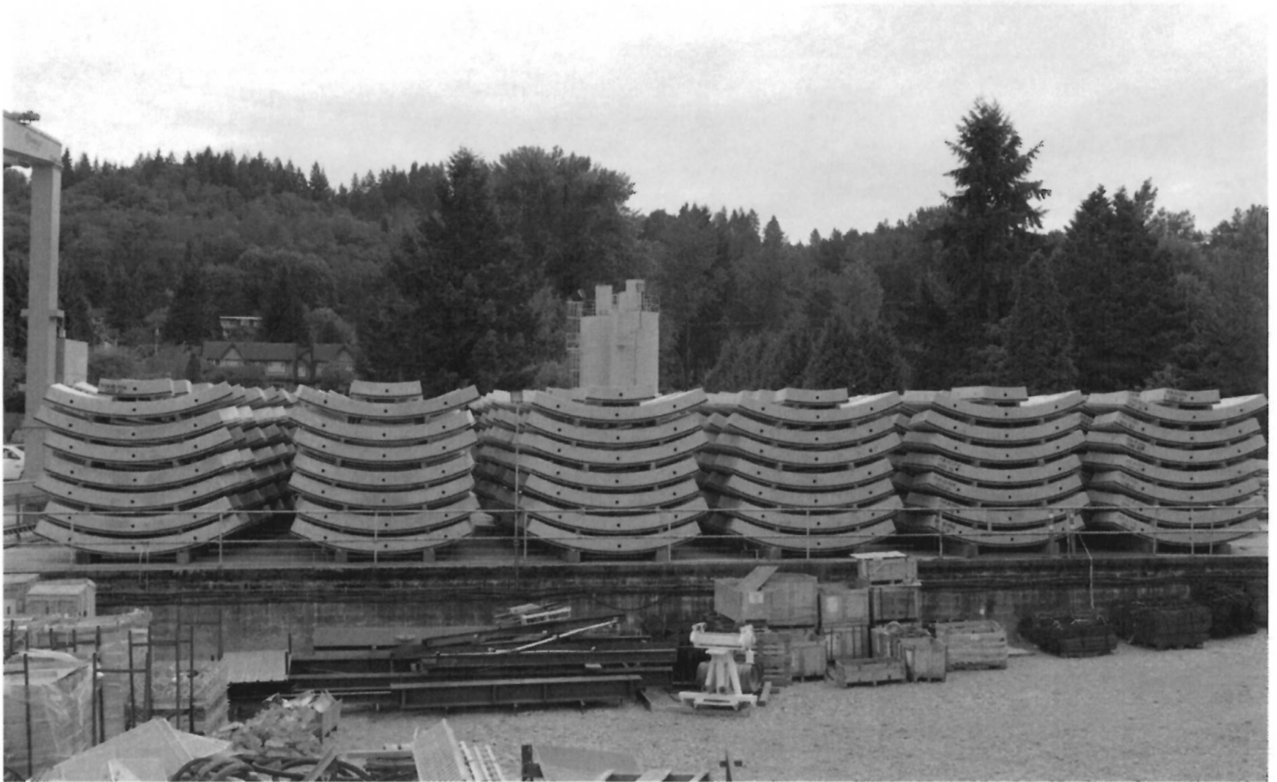
Tunnel liner rings waiting to be installed. Eight concrete segments are used to create each tunnel liner ring.
