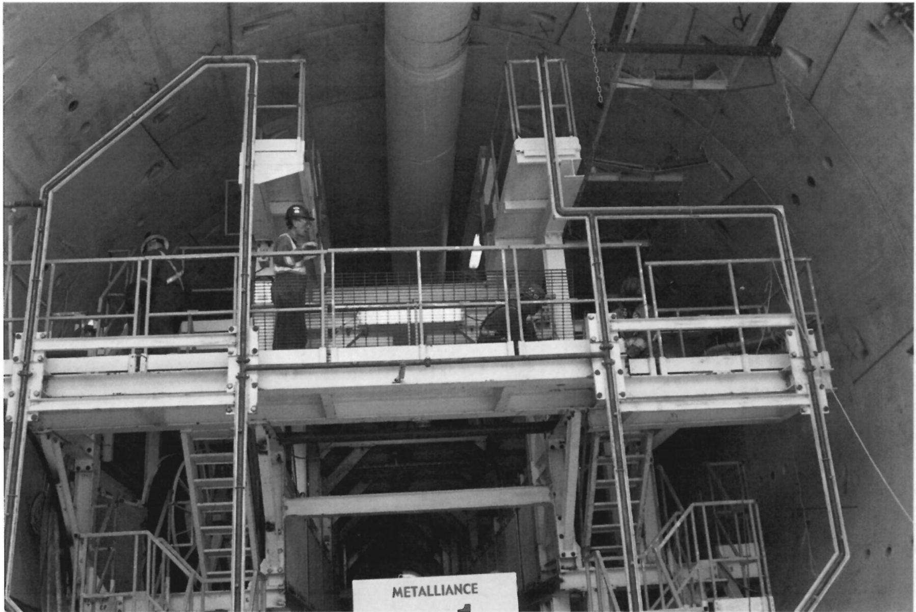
Crews assembling the TBM back up systems
