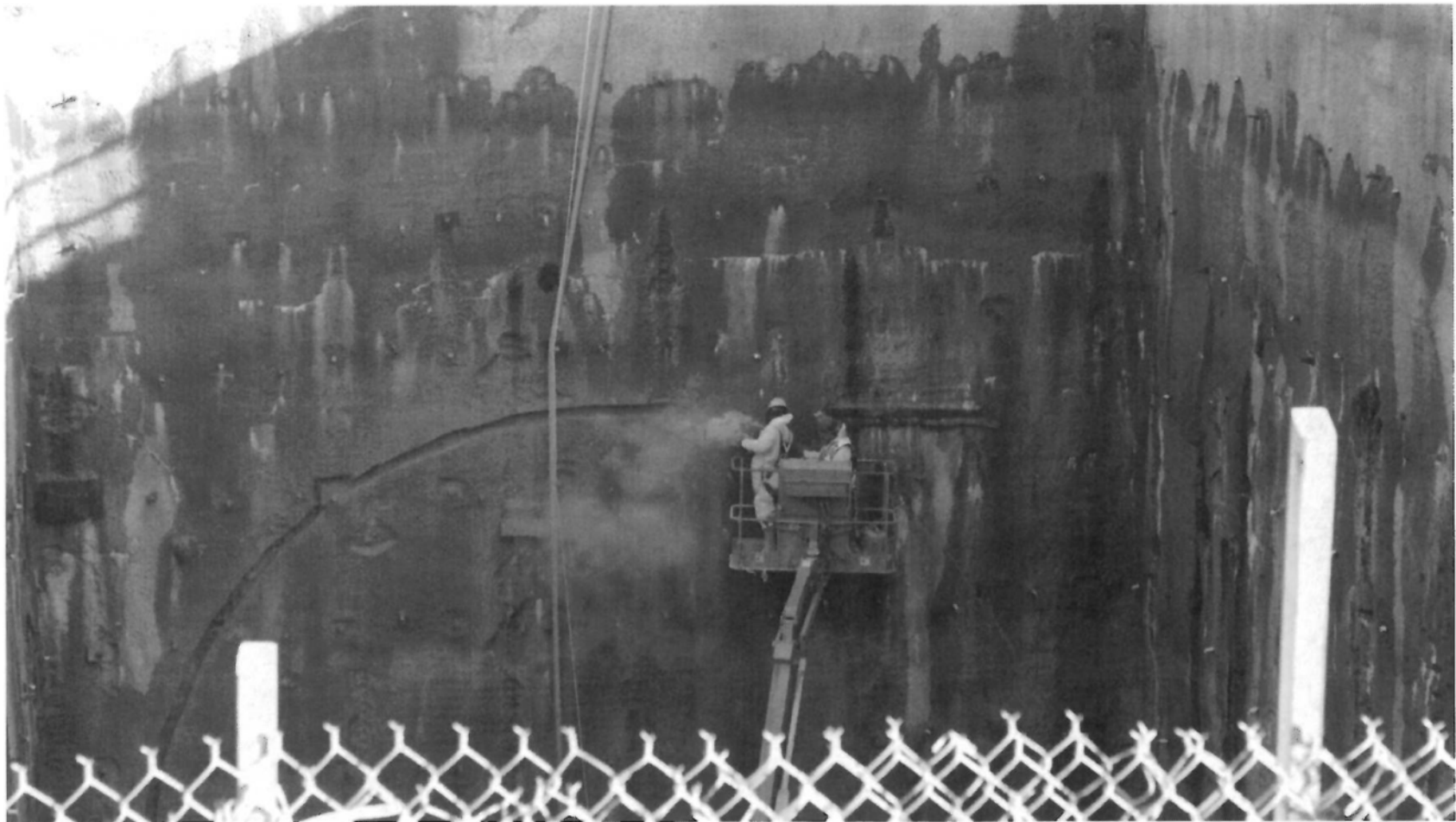
Crews pre-scoring the concrete in the TBM reception pit in anticipation of the TBM arrival
