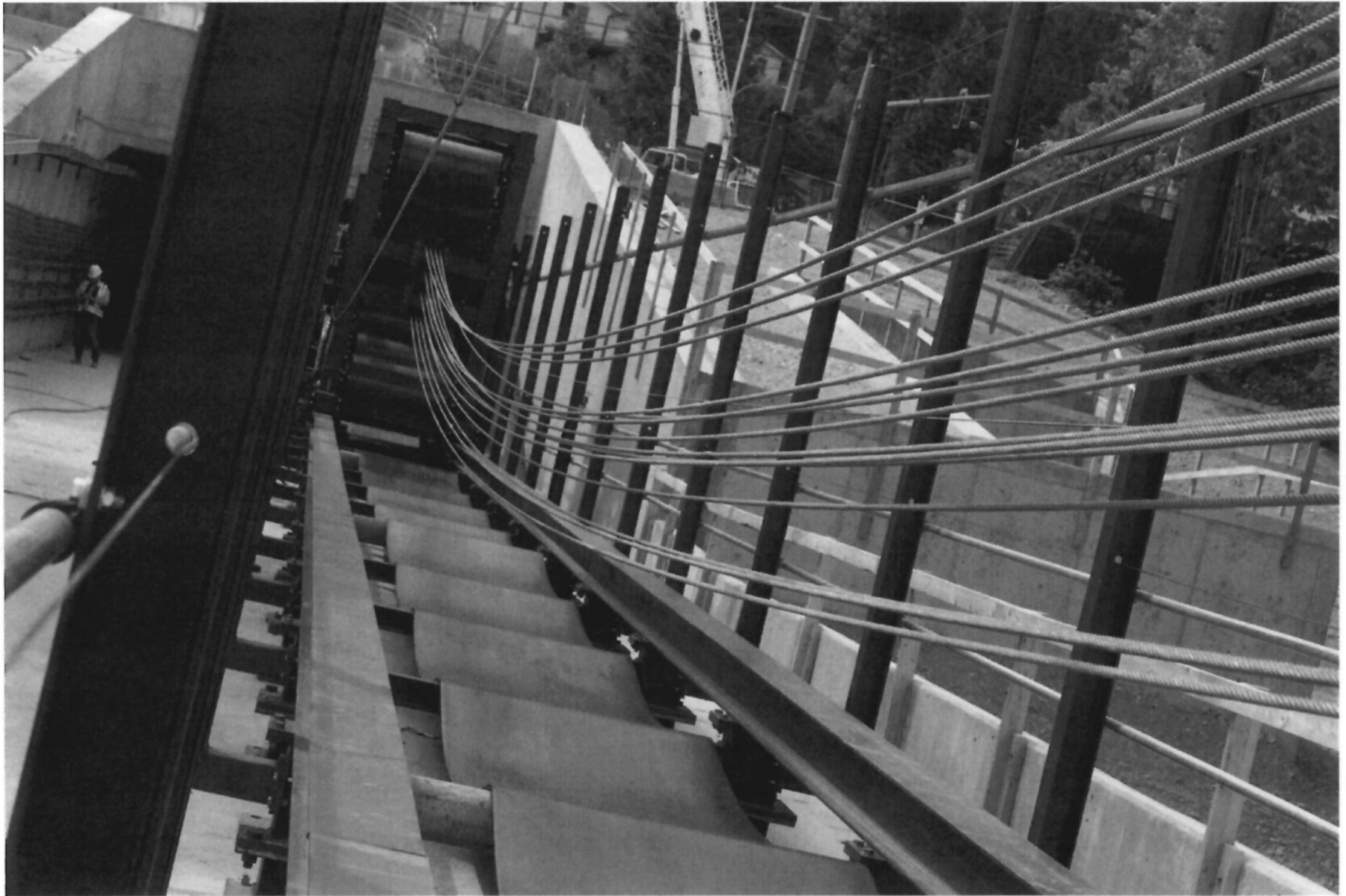
Conveyer belt assembly allows the spoils conveyer belt to be extended as the TBM progresses
