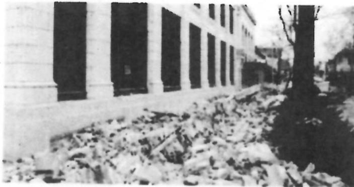
Unreinforced masonry structures may sustain significant damage from earthquakes.
