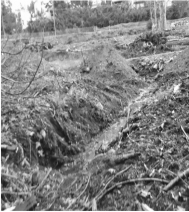
Newly constructed drainage ditch that collects sediment laden water and flows directly into Firehall Creek.
