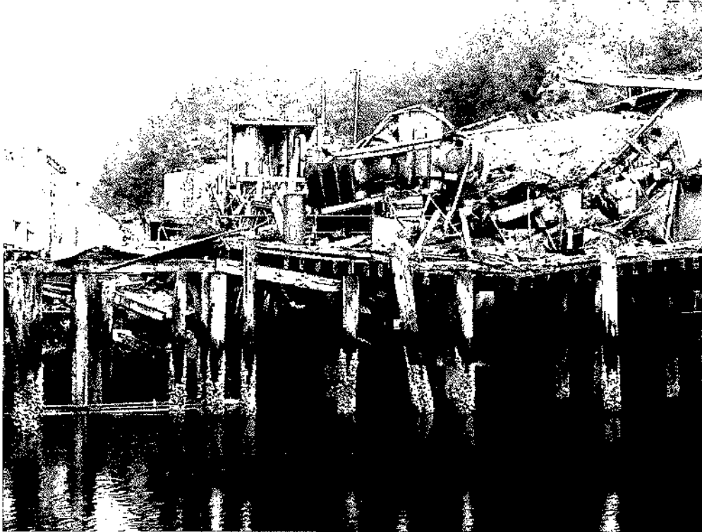
Photo 3. Metal debris (tanks and associated infrastructure) collapsed through decking onto foreshore. Obvious poor condition of pier structure.
