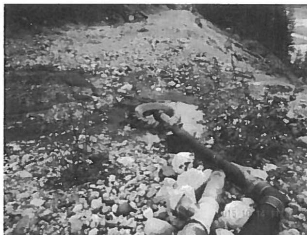
Photo 4: The neutral drainage is combined with the Portal Creek drainage into a HDPE pipe and diverted away from historical waste rock to the Tulsequah River
