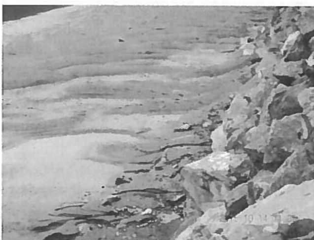
Photo 12: Diffuse discharge location through berm onto the Tulsequah river floodplain.
