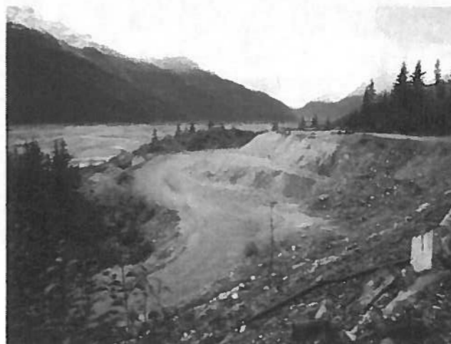
Photo 6: showing the historical PAG rock left from early mining. The ~80,000 tonnes of material to be relocated once mining restarts to the PAG dump on Rogers Creek.
