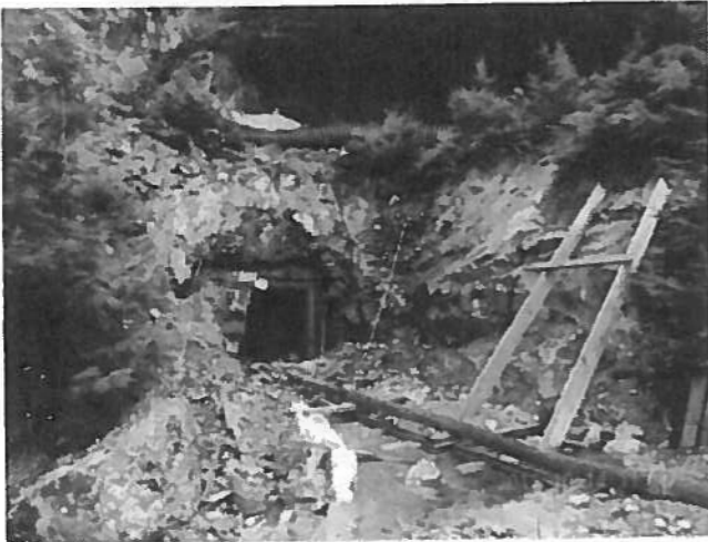
Photo 7: 5200 Portal. Acidic discharge is in smaller pipe exiting mine. 5400 non acidic and Portal creek water is contained in the larger pipe located above the portal.
