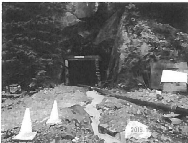
Photo 3: The black pipe is diverting neutral drainage captured underground; The Fe stained drainage (acidic) is flowing freely from the portal and is captured in a pipe in the foreground.
