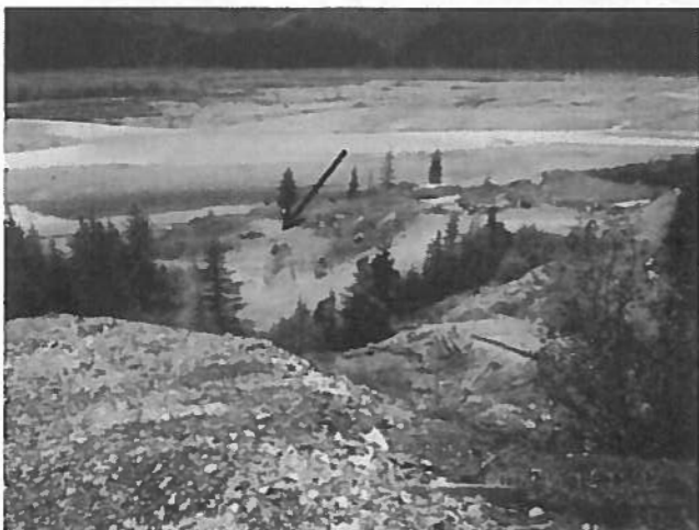
Photo 5: The black pipe (arrow) is the acidic discharge from the 5400 portal. Portal Creek and the combined non-acidic drainage discharge to the left of the picture in an underground HDPE pipe.
