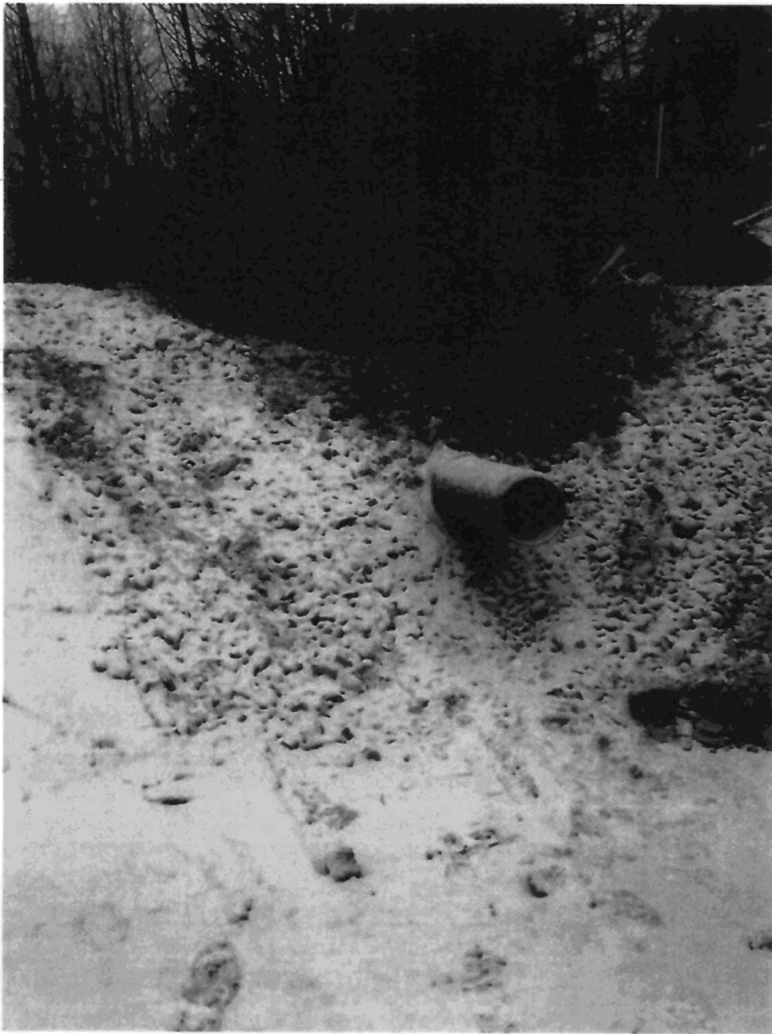
The above photo shows the low-level piped outfall and the spillway for the Sedimentation Pond.
