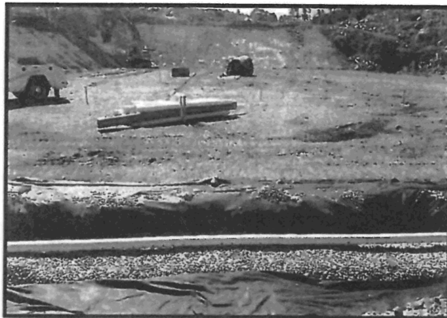
Photo 8 – Leak Detection and Leachate Collection Piping Systems
