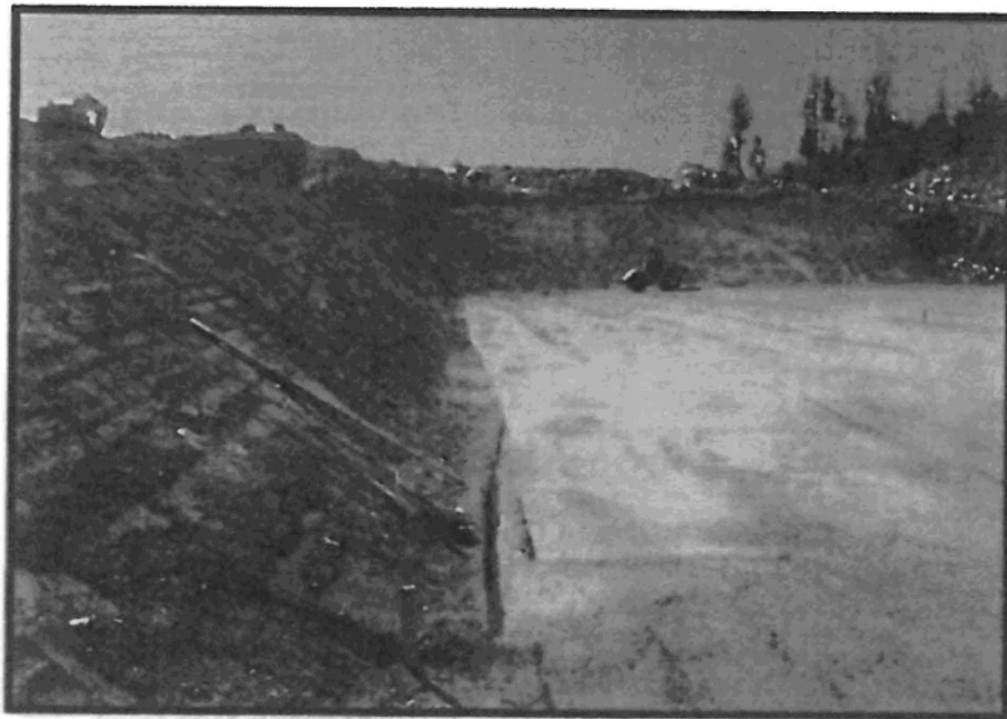
Photo 2 – Base sand surface being prepared for liner deployment
