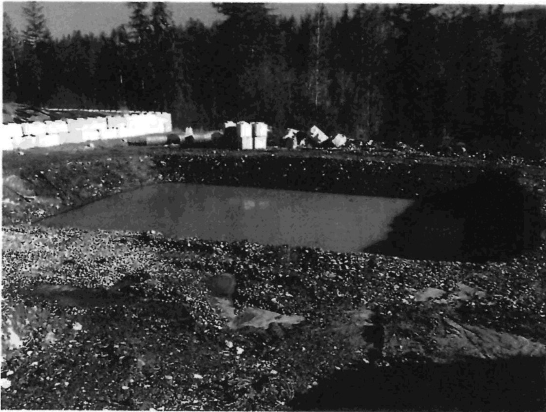
The above photo shows the Containment Reservoir prior to the liner being installed.
