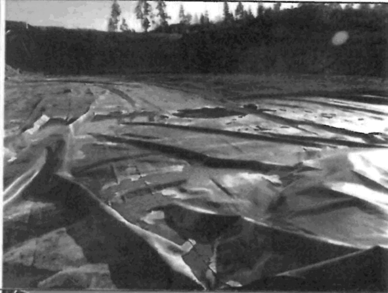
Liner in place on Nov 9 and second sand lift being placed. Looking south.
