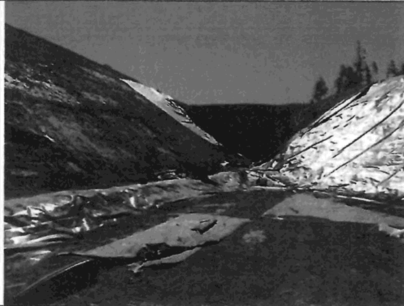
Installation of the membrane in progress at the south end of Encapsulation Cell 1C on June 29, looking south. The south end of Cell 1C is not yet finalized due to outcropping rock on the west side (red arrow).
