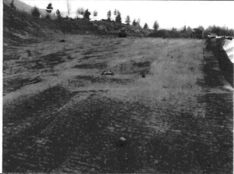
Compaction of clay liner in progress June 15, looking north
