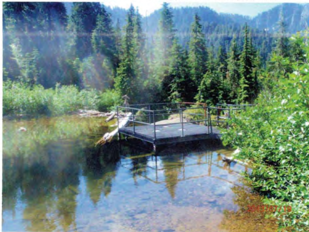
Figure 2: Current impoundment structure and platform at Chapman lake
