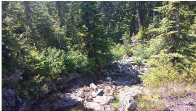
Photograph 1. ↑ Chapman lake downstream of dam left side
