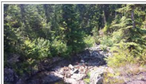
Photograph 1. ↑ Chapman lake downstream of dam left side
