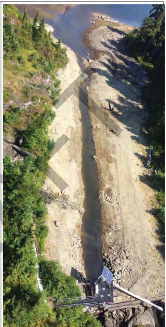
Photograph 6. ↑ Chapman Lake dam from inside lake area looking downstream
