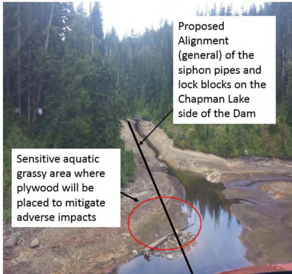
Figure 6. The proposed site at Chapman Lake showing the proposed alignment of the siphon lines and the sensitive aquatic grassy area to be protected as detailed in Table 3.
