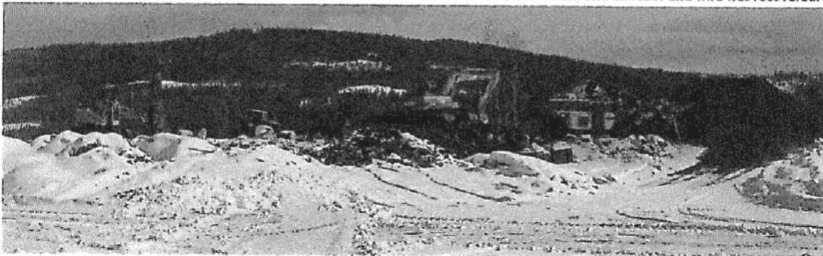
Photo below shows waste concrete reprocessing operation on March 3, 2011. This job provided full time work for 3 employees for one month during the winter "slow" season. Waste concrete was crushed and screened and all rebar and wire was recovered.
