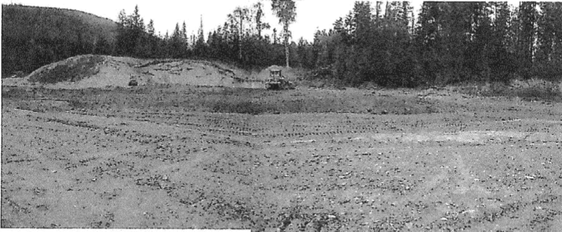
Wayne Mounce compacting the DLC landfill, recontouring/sloping as needed to achieve the required minimum slope for closure, applying final cover soil, etc. From now on, only "clean" earth fill will be deposited at this site; no more DLC waste.
