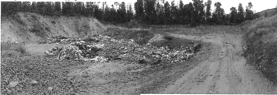
DLC waste gets compacted in 1 metre lifts and then a good layer of inorganic earth fill is applied as cover material.
