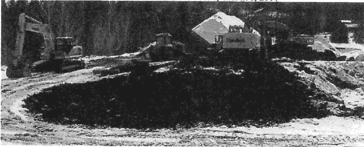
Nearing the end of the waste concrete reprocessing; 5600 m3 stockpile of aggregate (under snow) in the background.
