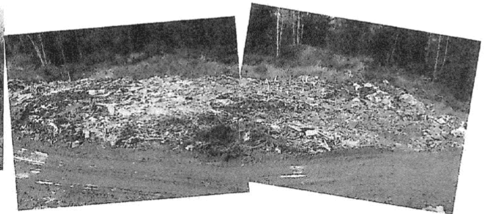
Compacted DLC waste in NW corner of landfill area. Soil cover to follow.
