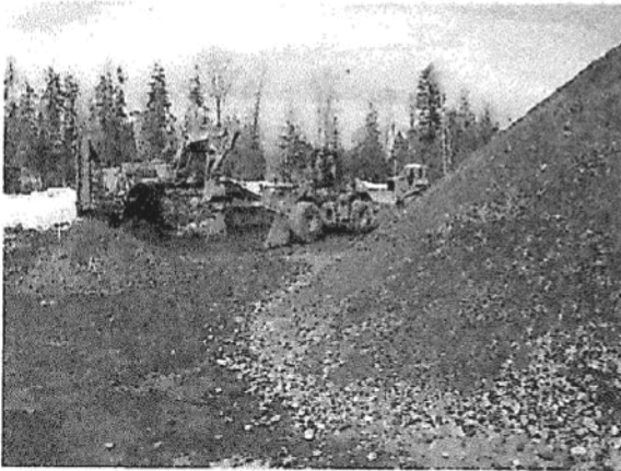
Crushed aggregate stockpile from waste concrete.
