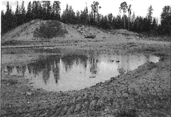
Fairly wet spring in 2011... water ponded on top of closed DLC landfill area. Final slopes will have to prevent ponding of water.
