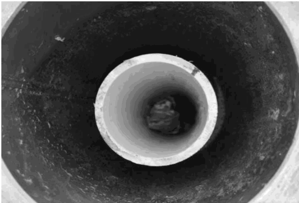
Photograph 6: Viewing the stuck waterra tubing stuck in the well.
