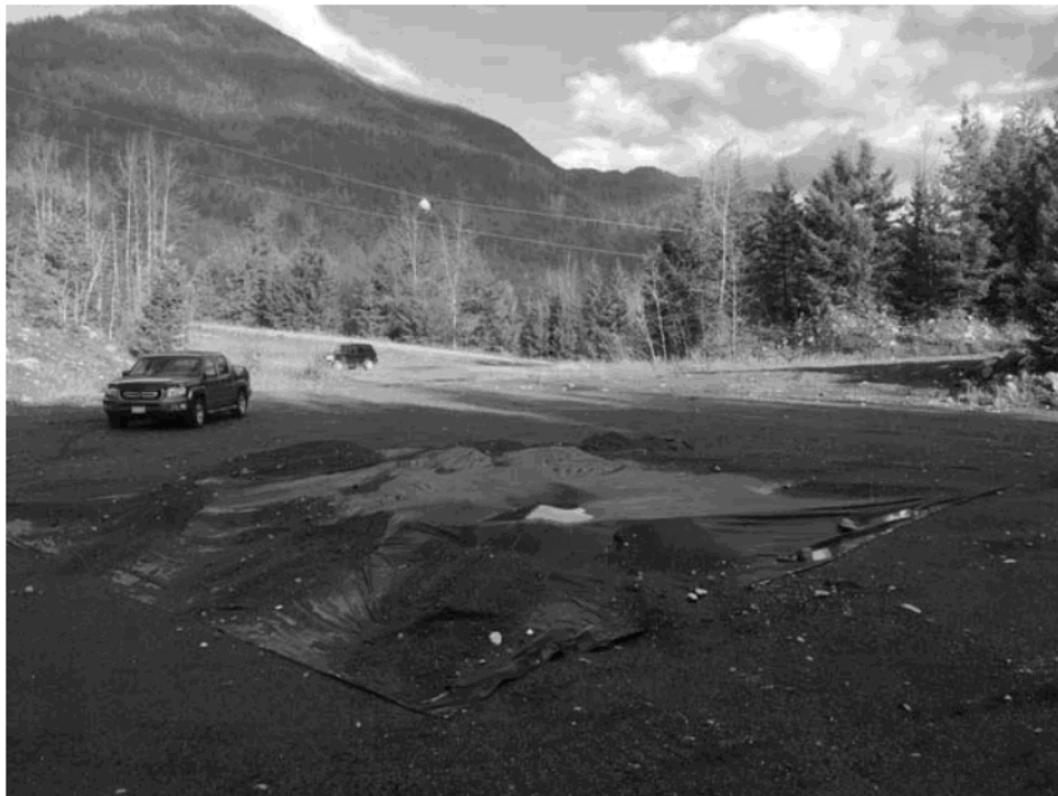
Photograph 2 – Tarp covered initial spill location looking down-gradient towards Kaslo West Road.
