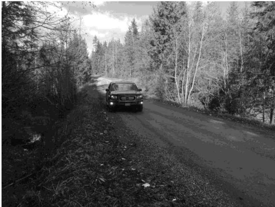
Photograph 9 – Loftstead Creek culvert crossing Kaslo Back Road. Soil sample 243.
