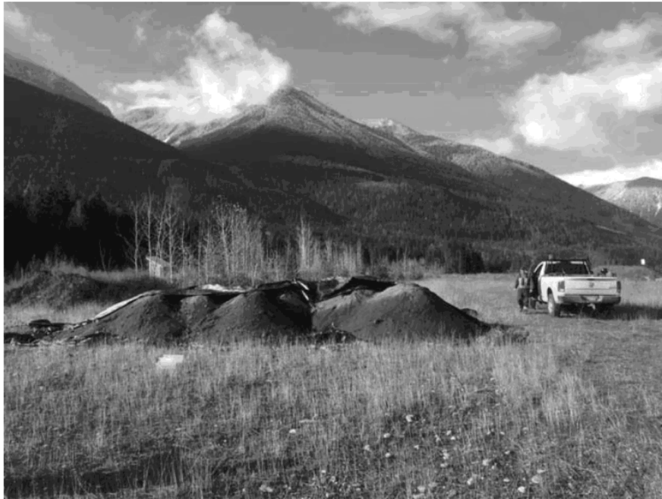
Photograph 3 – Covered and lined, suspect soil stockpile at west end of the airport.
