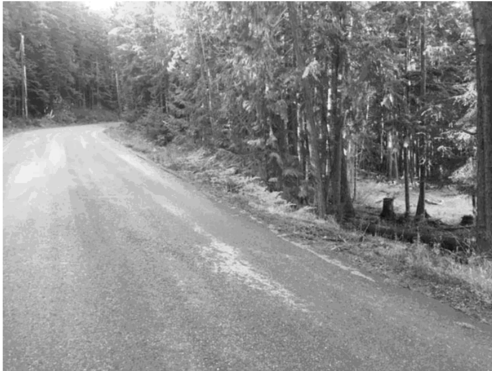
Photograph 8 – Surface water drainage swale towards bottom of Kaslo West Road hill. Soil sample 220.
