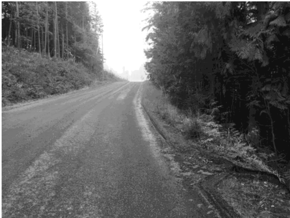
Photograph 8 – Surface water drainage swale on Kaslo West Road hill. Soil sample 217.
