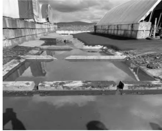
Spillway/settling chambers AFTER UPGRADES
