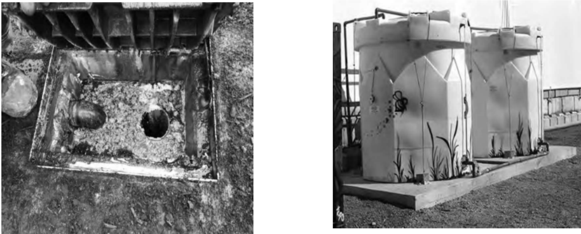
In Ground Leachate Collection – Bays 1-10 / Aerated Double Walled Leachate Storage Tanks
