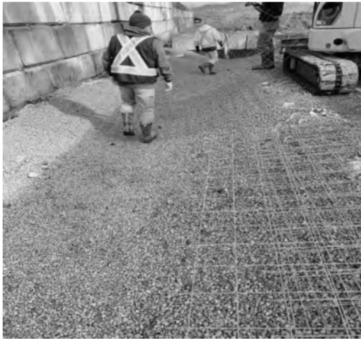
Removal of Soil / Installation of Reinforced Concrete and Pavement Skirting (cleaning)
