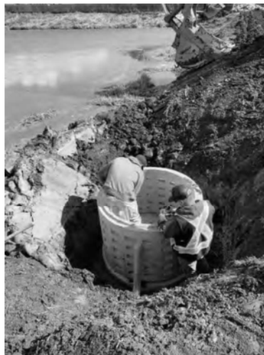
Transfer Pump and Sump (April / May 2020) / Installation of Wet Well / New Pond / Spillway
