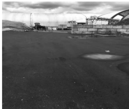
Standing Water Areas: Asphalt Damage (Before) Asphalt Re-Paving March & April 2020
