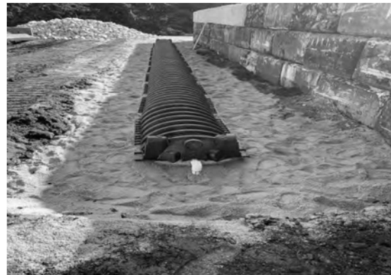
Septic Field Reconstruction (Mar.2020)
