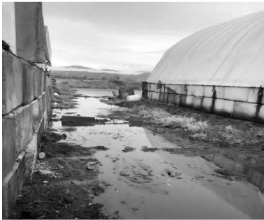
Spillway/settling chambers BEFORE
