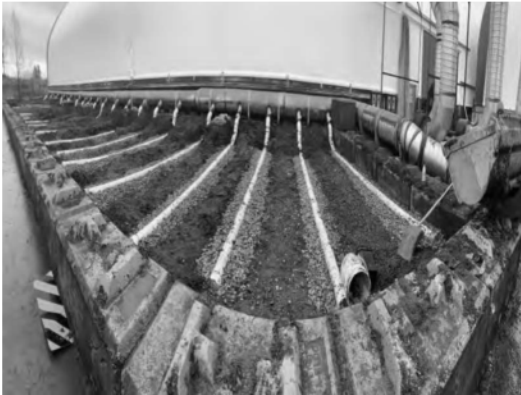
Biofilter Reconstruction (Jan / Feb. 2020)
