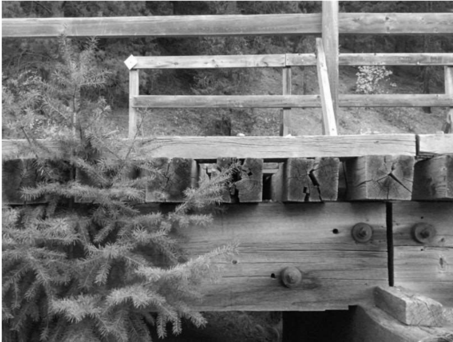
Photo 13 Typical deck tie condition
