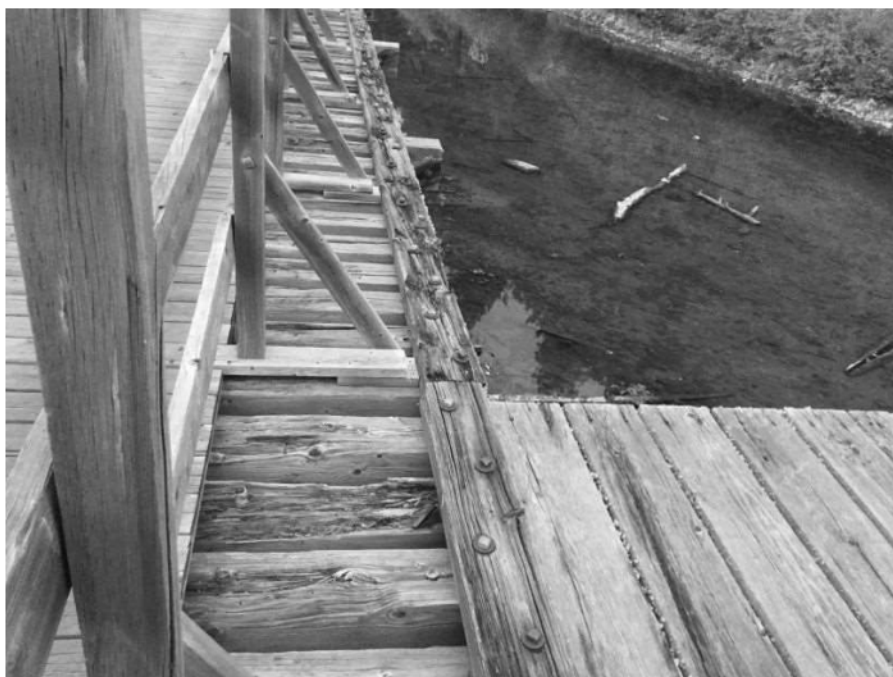
Photo 11 Typical deck tie condition
