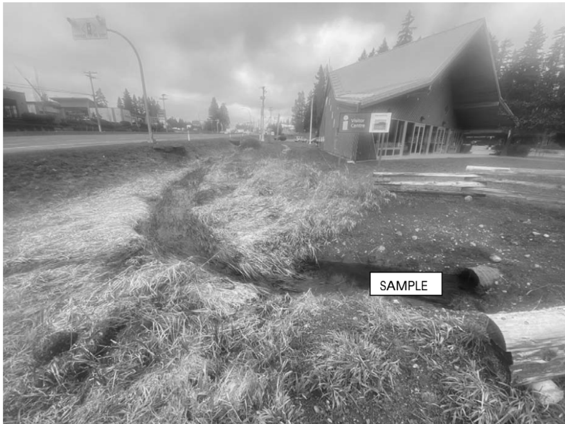
Photo 5 (above): View looking north of entire drainage ditch next to Forest Discovery Center, and where water enters the greater drainage system via underground culvert. Sample location at the culvert, annotated in photo.
