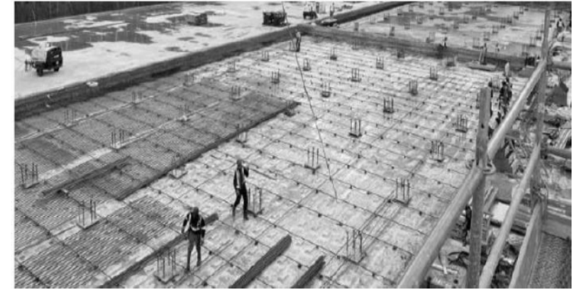
LNG Facility: Rebar Installation at Stormwater Pond
