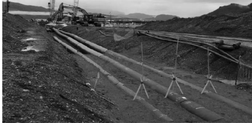
High-Density Polyethylene Pipe in main Utility Corridor (near MOF)
