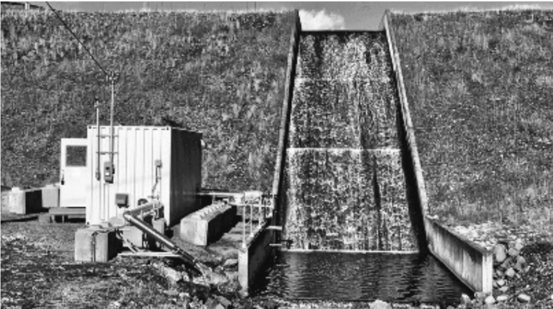
One of five treatment facilities to prevent further spread of calcite formations.
